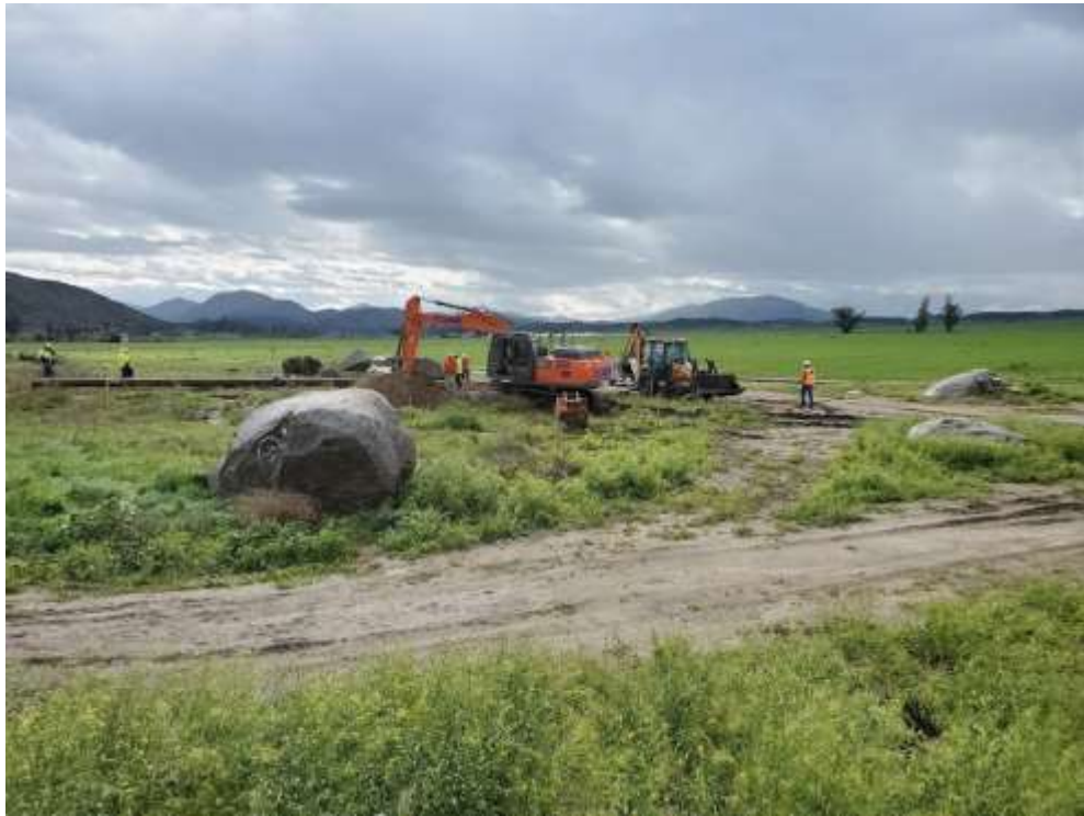
Photo 1 – Excavating to set wood pole at Construction Area UNK86 (March 10, 2020).
