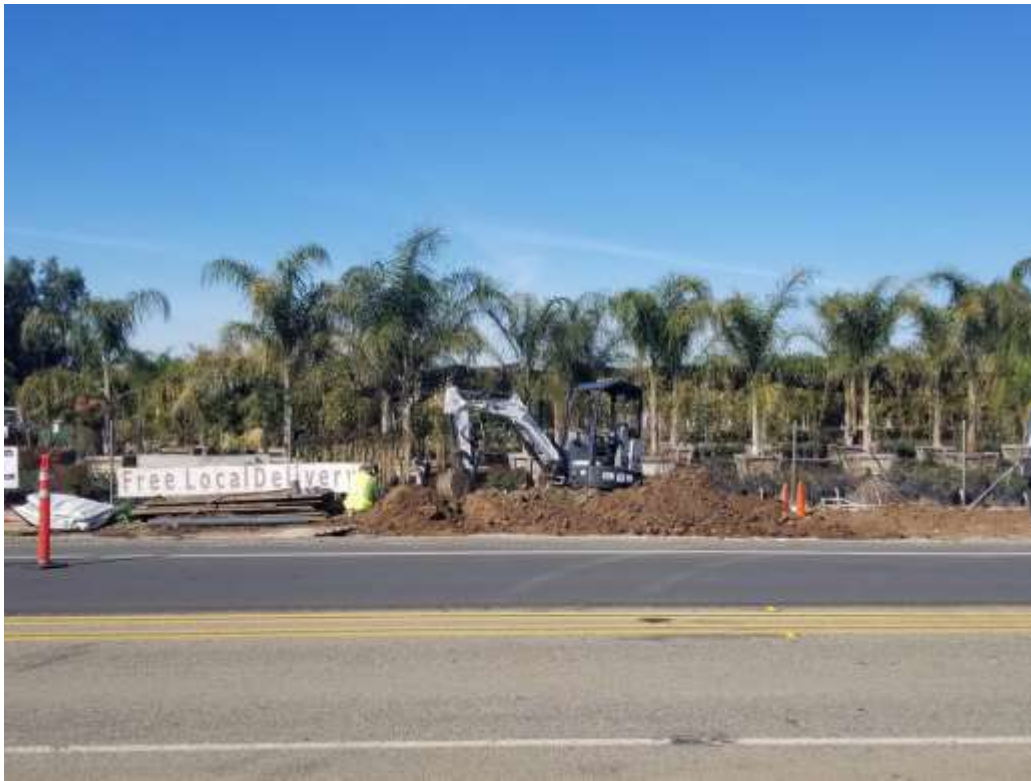
Photo 3 – Vault work at Construction Area UNK188 (March 8, 2020) (Photo courtesy of SCE).
