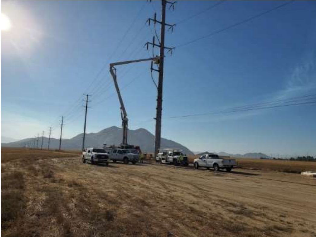
Photo 1 – Completing loops and installing cable straps at Construction Area UNK250 (August 3, 2020).
