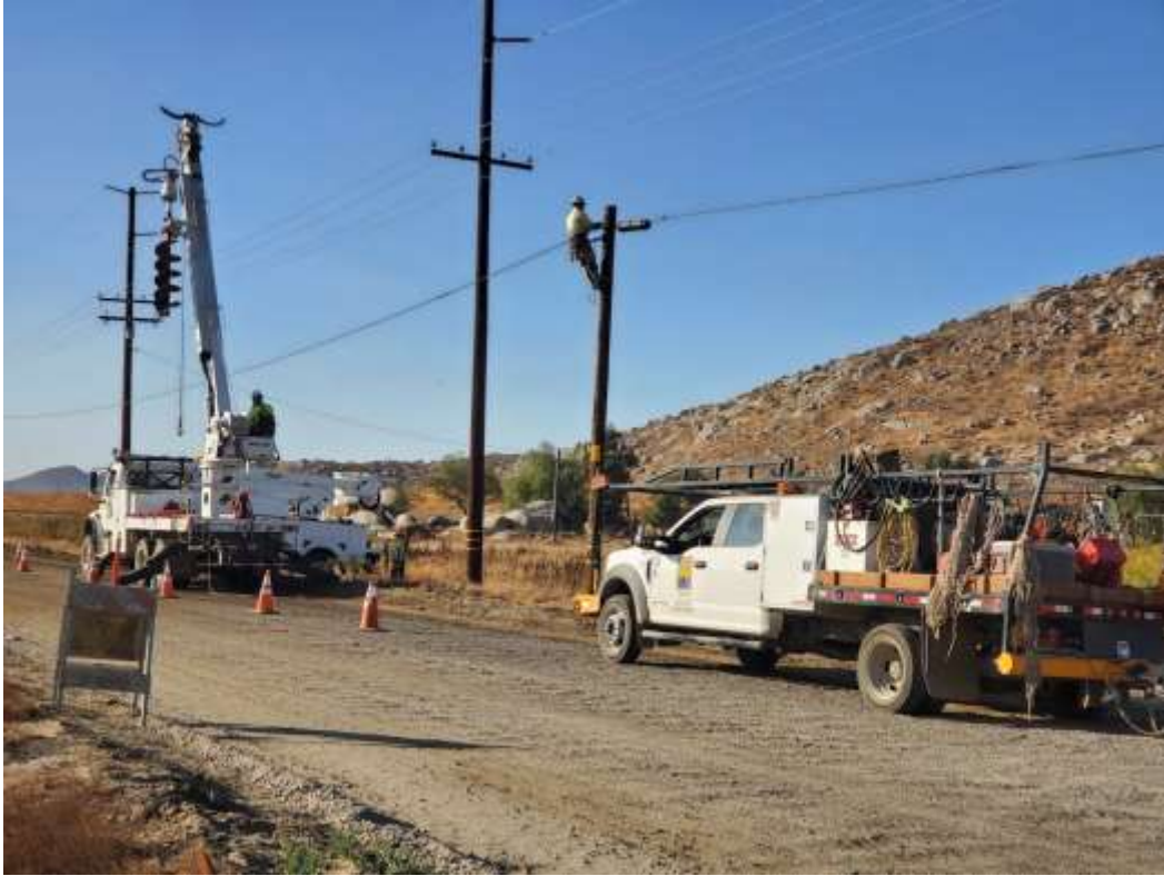
Photo 3 – Pole butt removal at Construction Area UNK56 (September 23, 2020).
