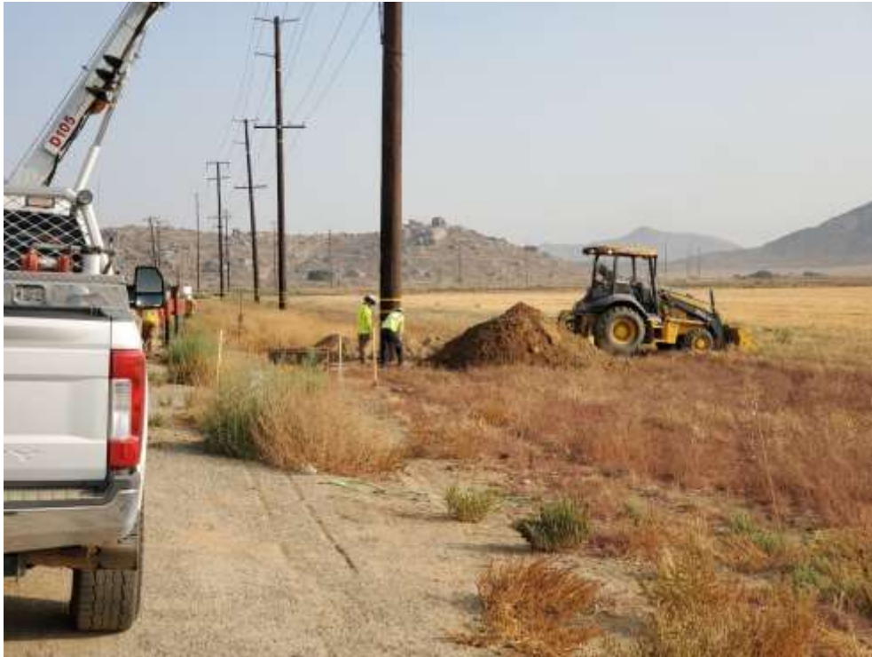
Photo 1 – Pole realignment at Construction Area UNK101 (September 15, 2020).
