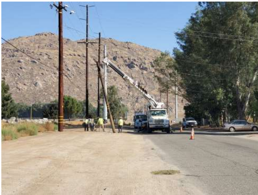
Photo 2 – Pole butt removal at Construction Area UNK21 (September 29, 2020).
