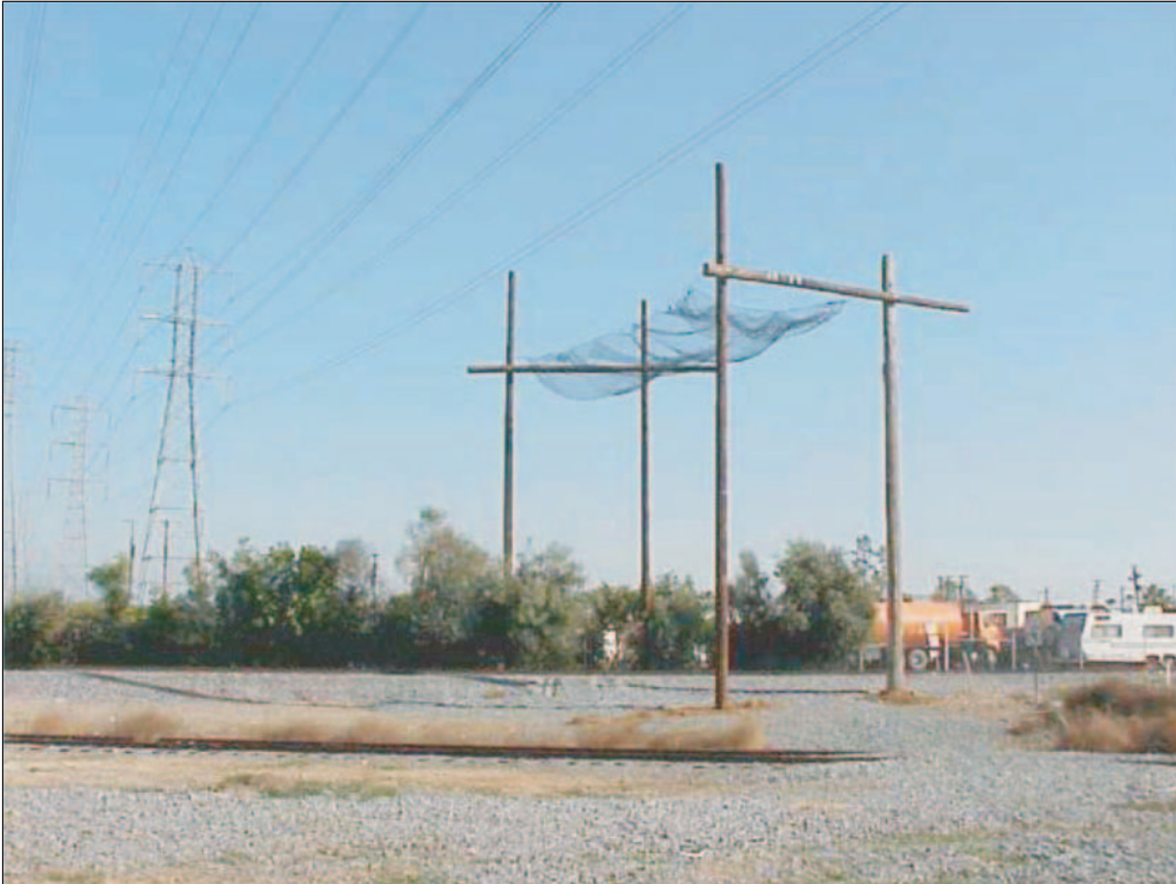
Railroad Under-Crossing (H-Frame Configuration with Net)
