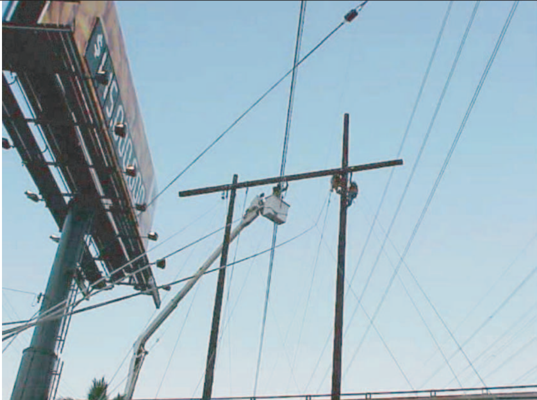
Low Voltage or Street Under-Crossing (H-Frame Configuration)
