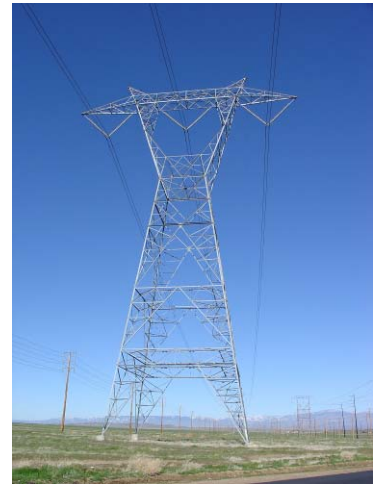
Single-circuit 500-kV tower
