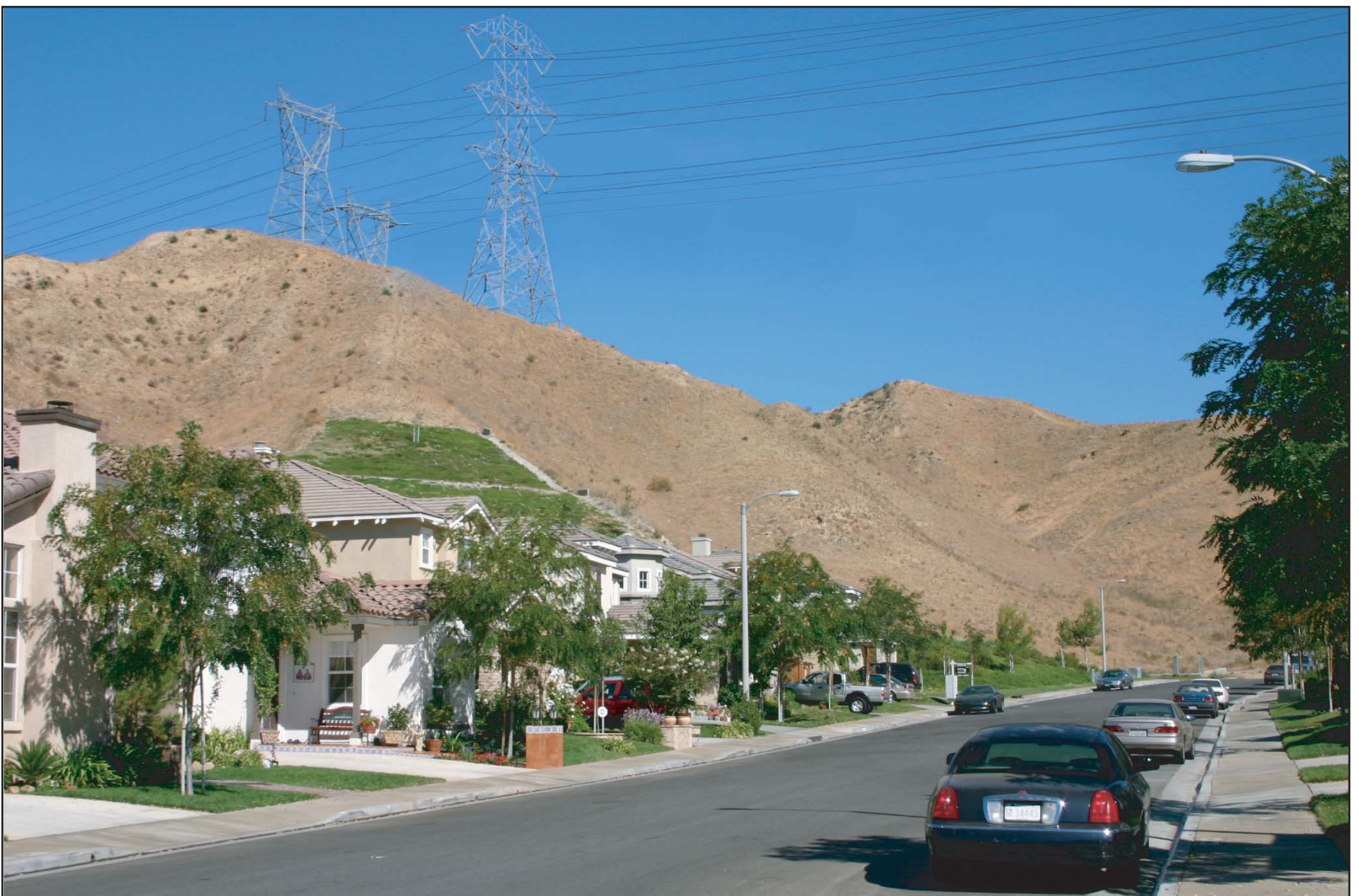
B 500 kV transmission line replacement as seen from KVA Seg 1-6.
