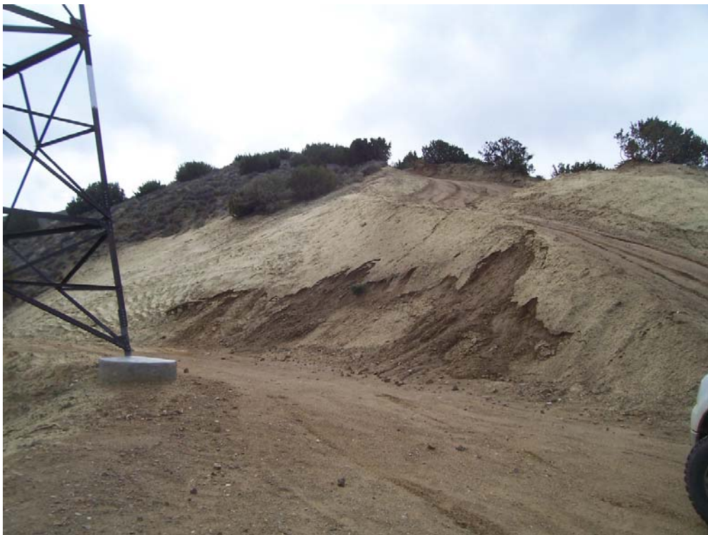
Figure 2: Erosion slumping at Tower 23, Segment 2.
