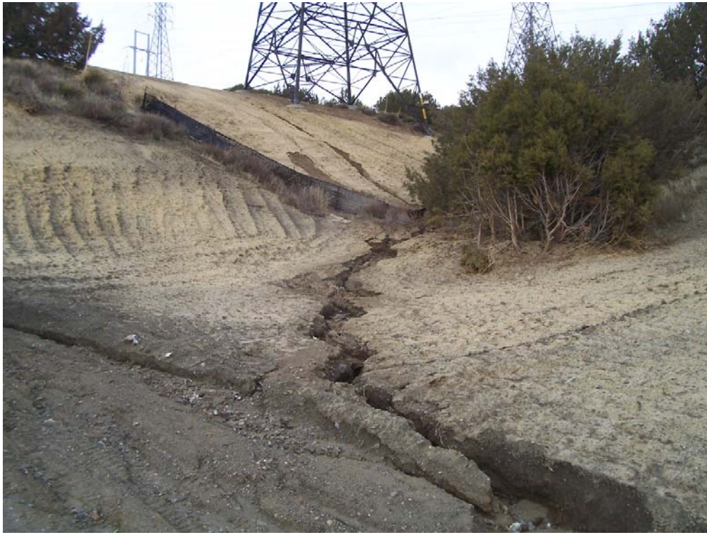
Figure 3: Erosion rilling at Tower 34, Segment 2
