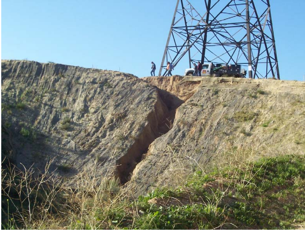
Figure 1: Erosion incising at Tower 9, Segment 1.
