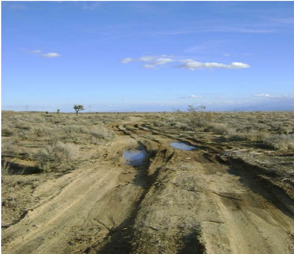
Figure 4: Rutting within Tower 43 overland travel access due to OHV use.
