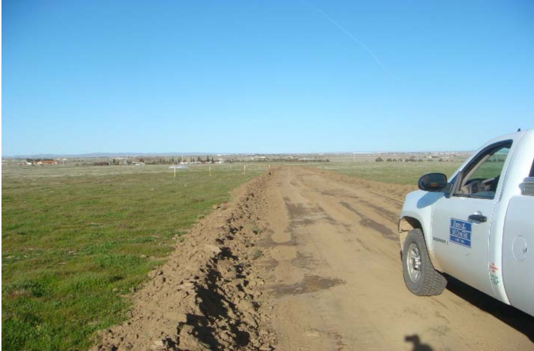
Figure 1: Permanent road construction for the 66 kV relocation surrounding the Antelope Substation expansion area.
