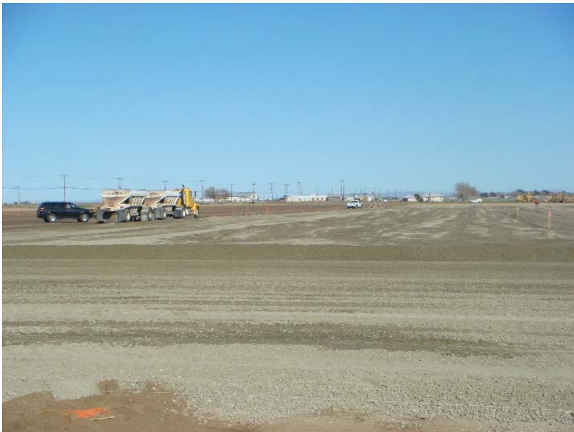
Figure 2: Rock placement at TRTP Yard 28 in Lancaster.
