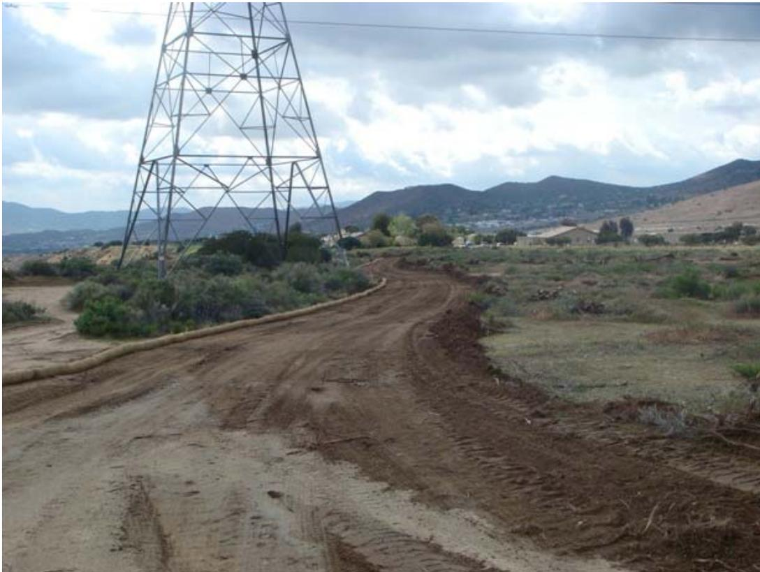
**Figure 4:** Grading of an access road for BMP installation at the Vincent Substation Expansion area.
