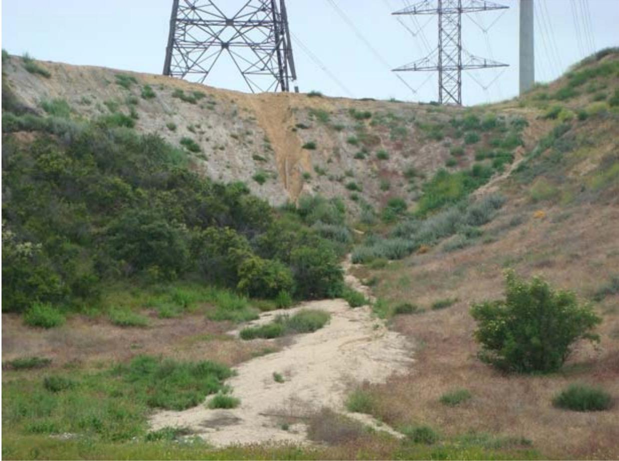
**Figure 1:** Erosion at Tower 9 in the City of Santa Clarita, Segment 1. A plan for repairs at this location is currently under review by SCE.
