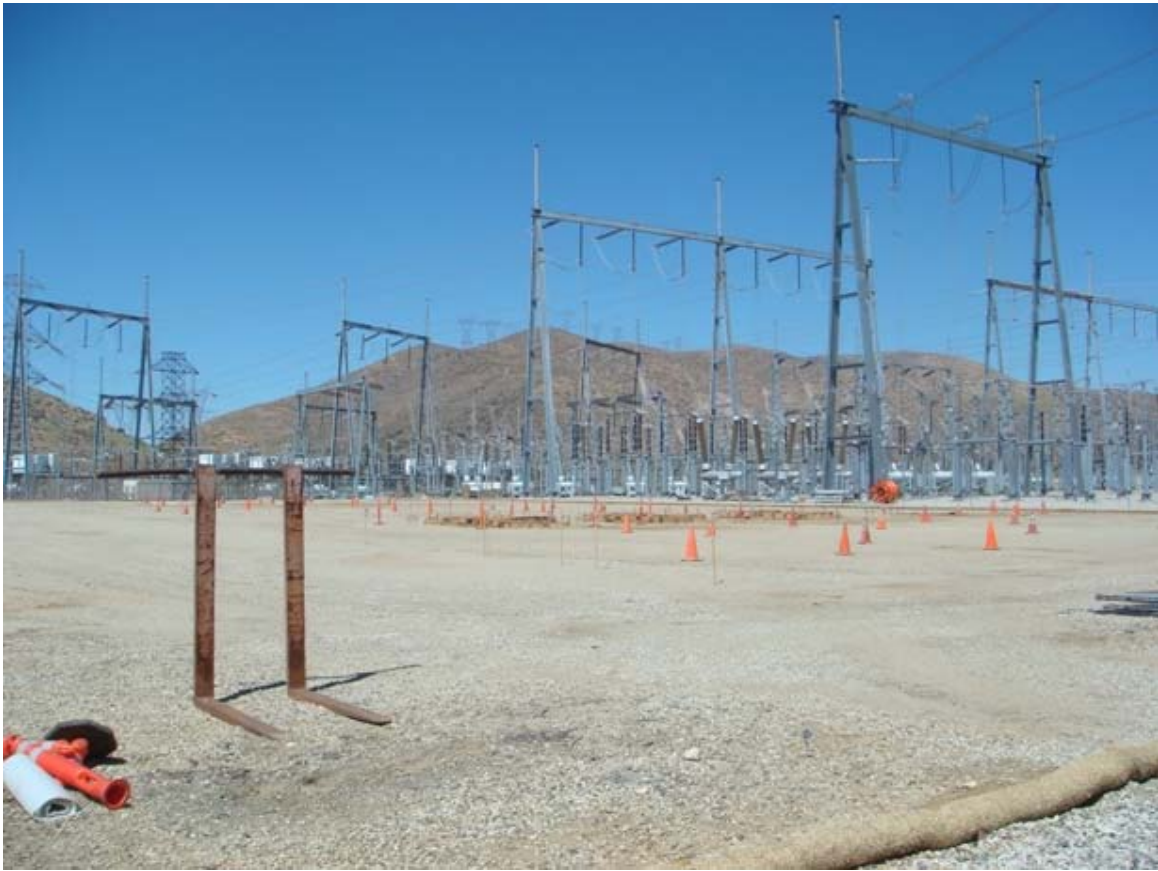
Figure 2: Construction at the Vincent Substation within the existing substation.
