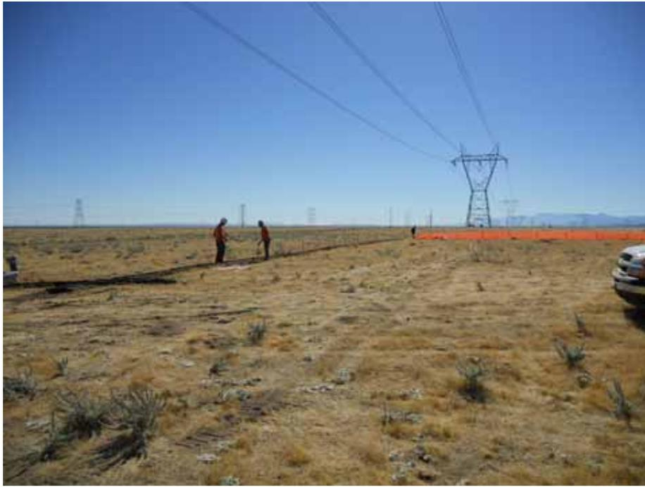
**Figure 3:** H&H Grading installing silt fence at Tower 34, Segment 4.
