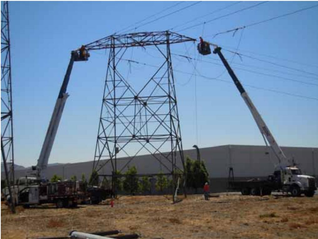
**Figure 6:** Segment 8 Phase 1 crews attach travellers to wreck-out towers in preparation to remove 220 kV wire.
