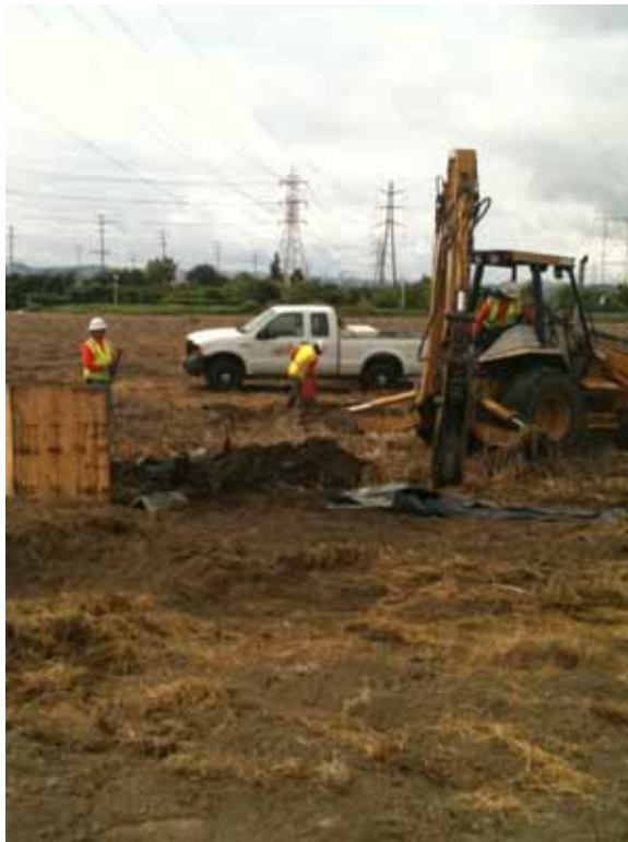
Figure 4: A DCX crew removes a foundation in the City of Chino, Segment 8 Phase 2.
