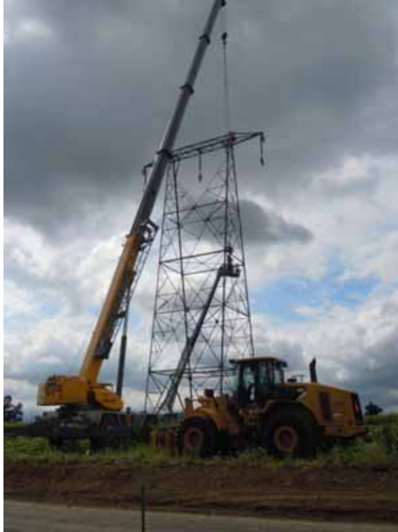
Figure 3: A Wilson crew works to remove a tower in the City of Ontario, Segment 8 Phase 2.
