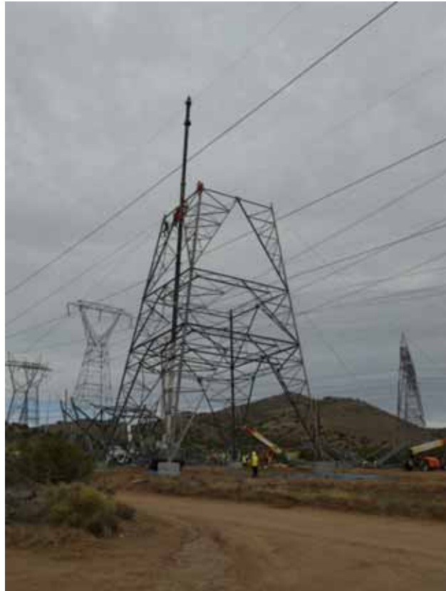
Figure 1: Tower 61 steel assembly near the Town of Acton, Segment 5.
