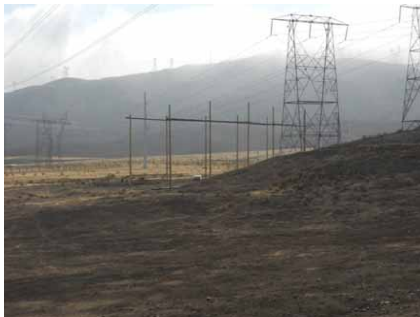
Figure 2: Guard pole structure to protect the Sagebrush Transmission Line at Tower 37, Segment 5.
