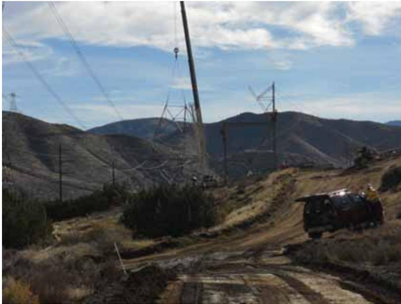
**Figure 3:** Wreck-out of 220 kV Tower M75-T2, Segment 5.
