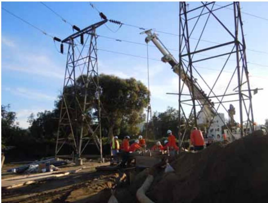
**Figure 4:** A Wilson crew sets a riser pole foundation within the Duck Farm, Segment 7 66kV.
