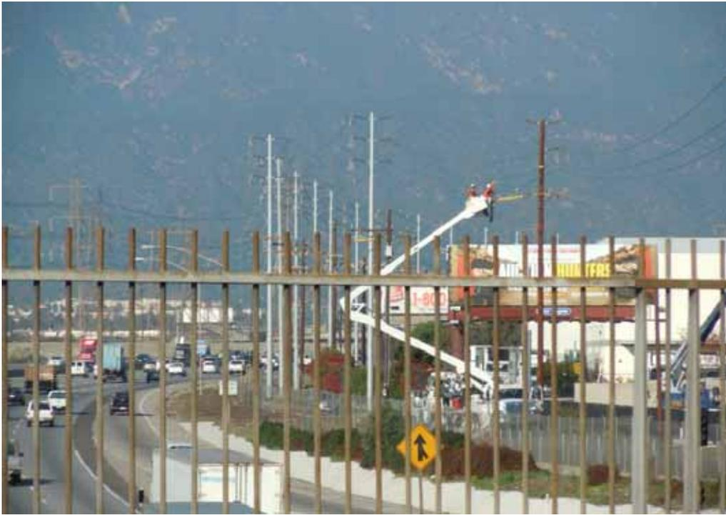
**Figure 5:** A Wilson crew installs lightweight steel poles adjacent to the I-605 freeway on the Rio Hondo–Amador-Jose-Mesa 66kV line, Segment 7.
