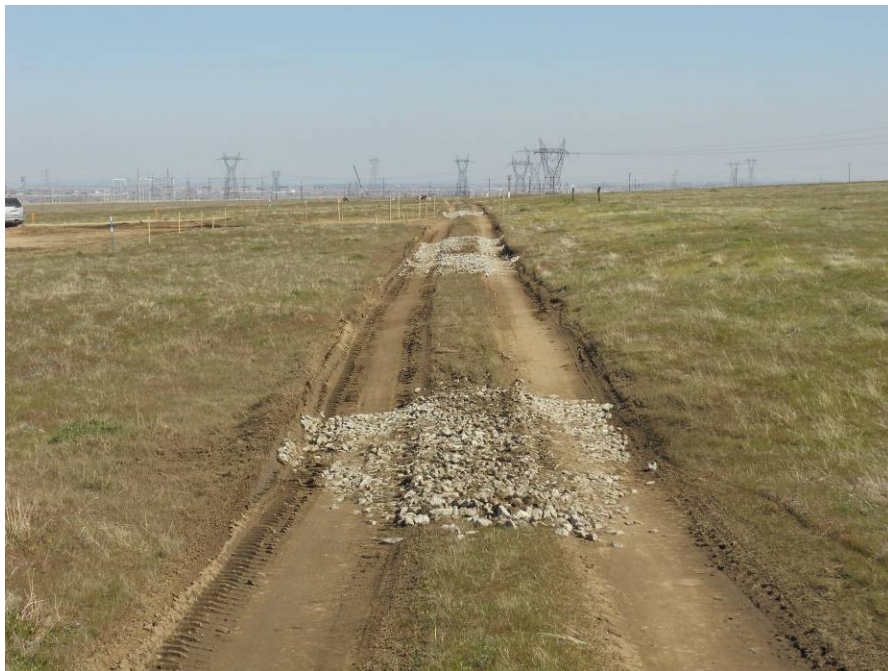
Figure 2: Rock placed in access road that leads from 110 th Street to the Antelope Substation, Segment 4.
