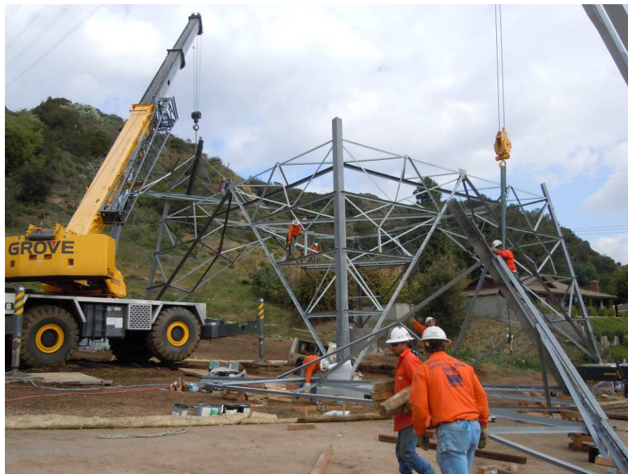
Figure 6: Crews assembling Tower M54-T3a, Segment 7.
