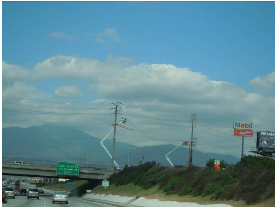
Figure 5: Crews stringing wire, Segment 7 66 kV.
