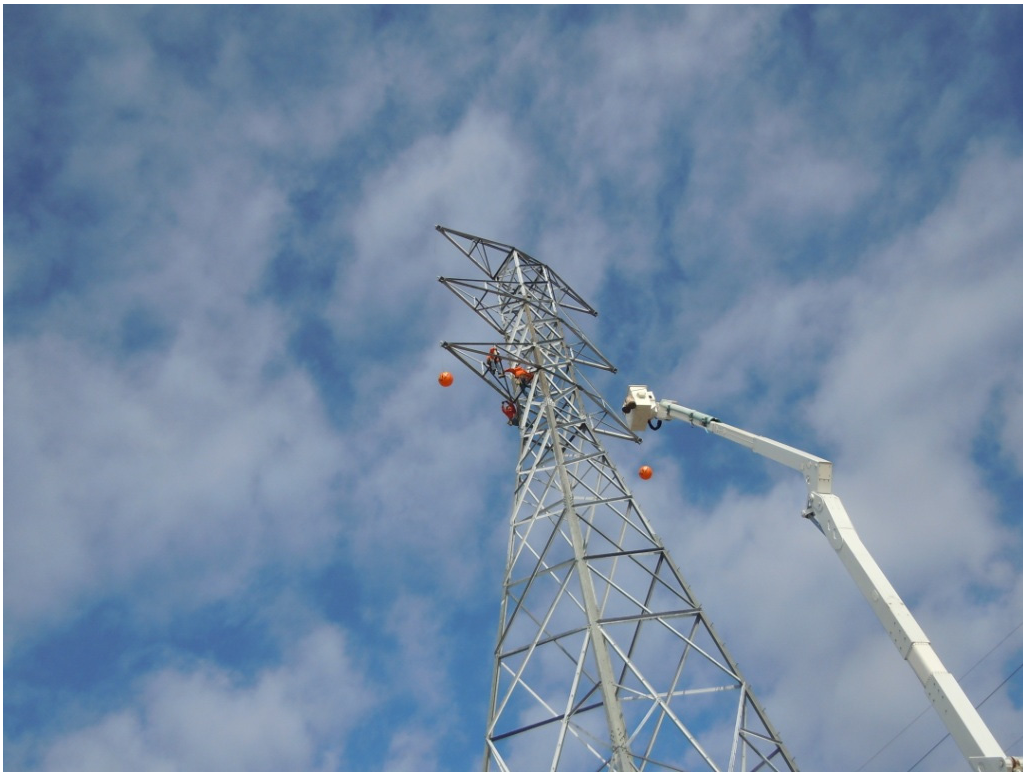
Figure 7: Crews assembling a tower and installing bird deterrents, Segment 8 Phase 2.
