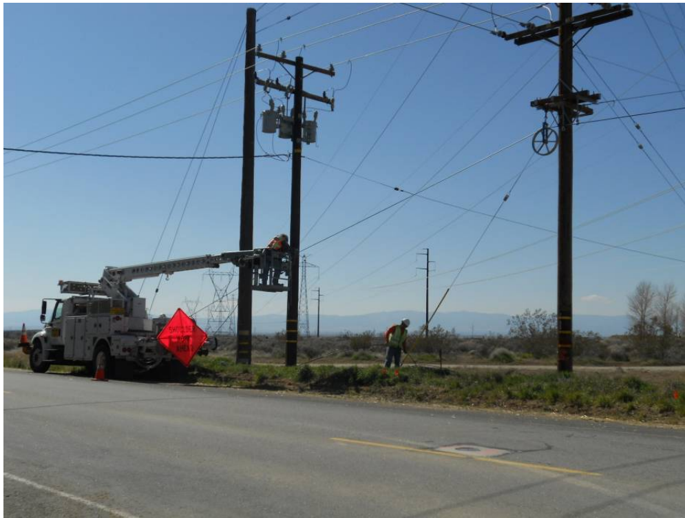
Figure 3: H&M crew pulling fiber optic cable along Tehachapi Willow Springs Road, Segment 10 Telecom.
