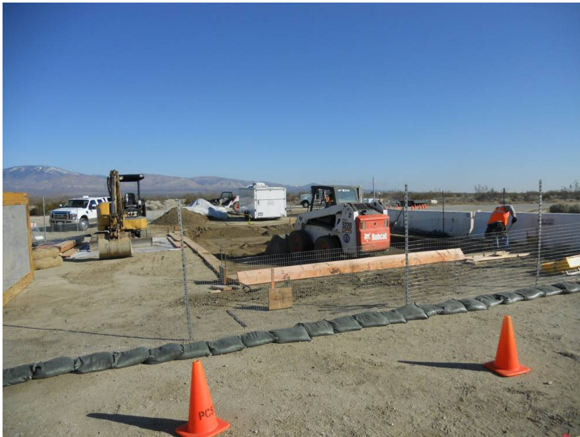
Figure 4: Concrete slab installation over the LADWP aqueduct in the disturbed area along Rosamond Boulevard and 170 th Street at Whirlwind Substation, Segment 9.
