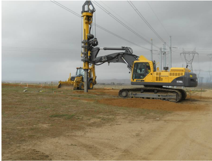
Figure 1: KV Structures drilling Tower 3A-102, Segment 4.
