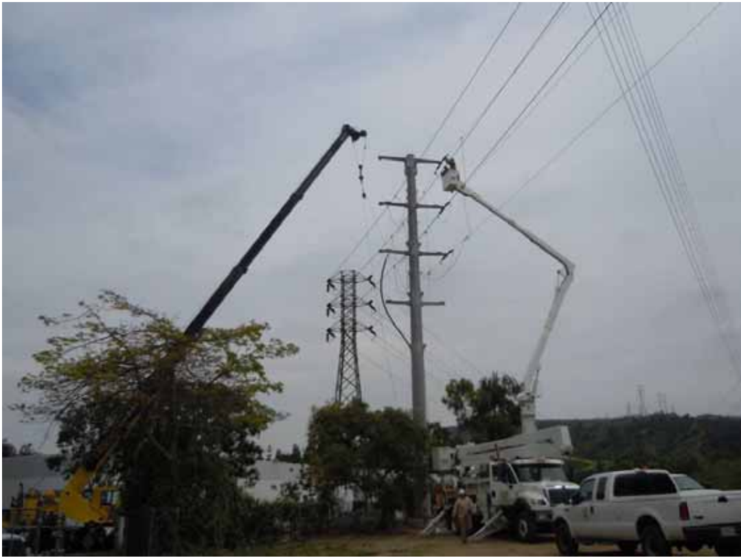
Figure 7: Crews install a pole at Pellisier Place, Segment 8 66 kV in the City of El Monte.
