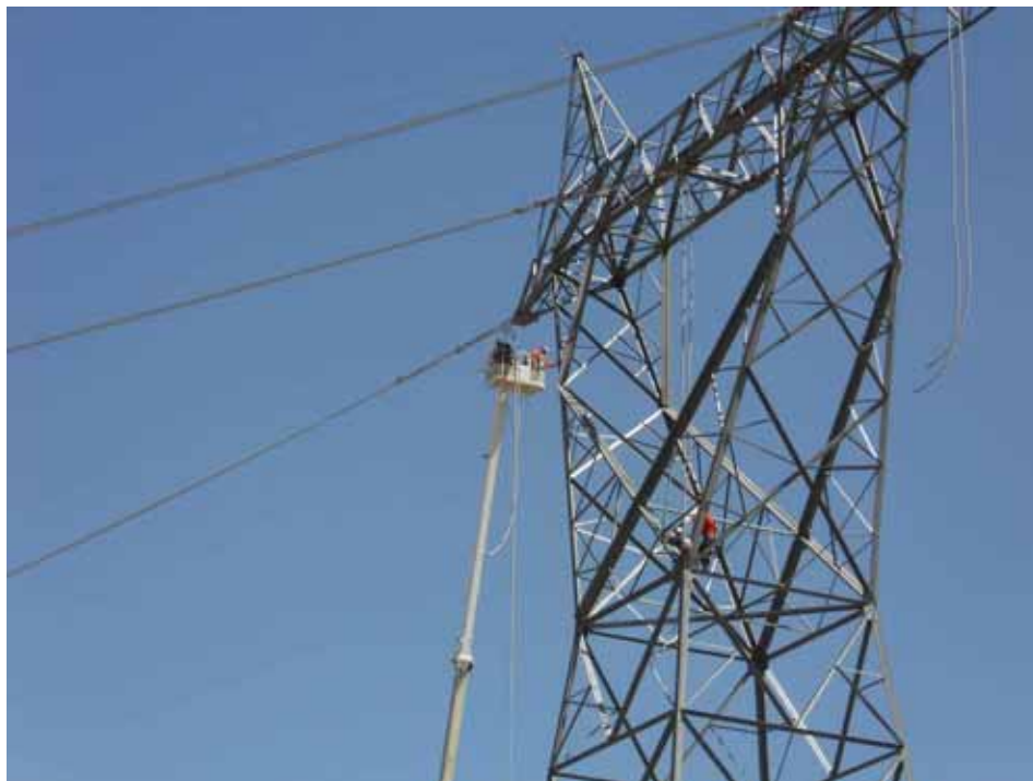
Figure 4: H&M wire crew tensioning wire from Tower 2 into the Antelope Substation, Segment 5.
