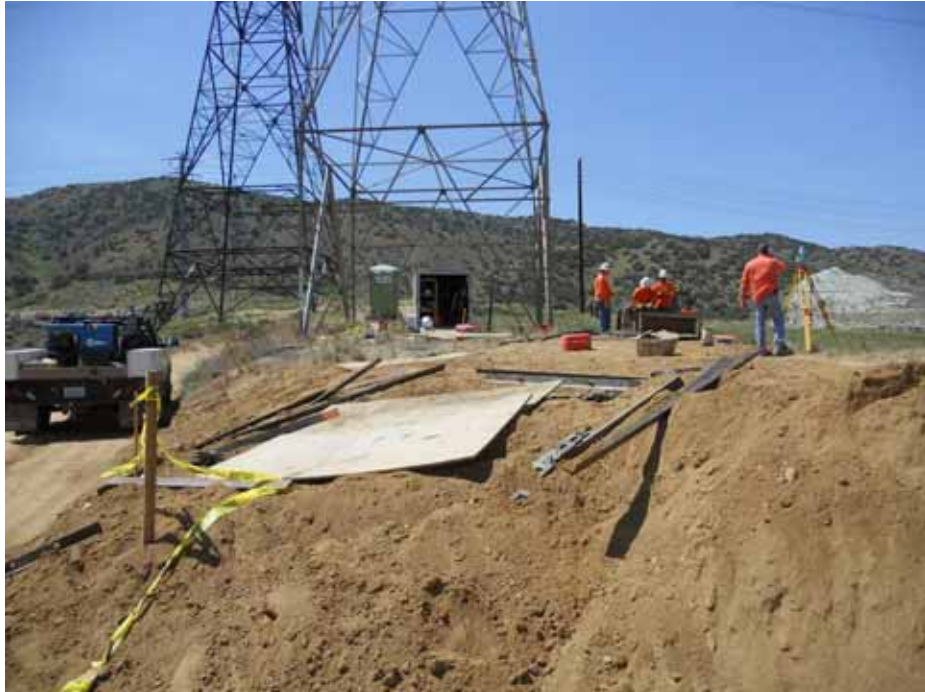
Figure 2: Woodward Brothers (drilling contractor) setting up Tower 16, Segment 5.
