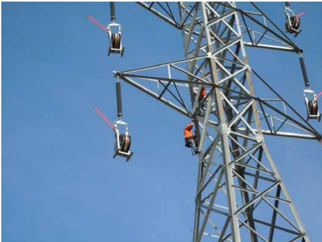
Figure 10: Wilson linemen remove a partially built Cassin's kingbird nest Segment 8, Phase 2.
