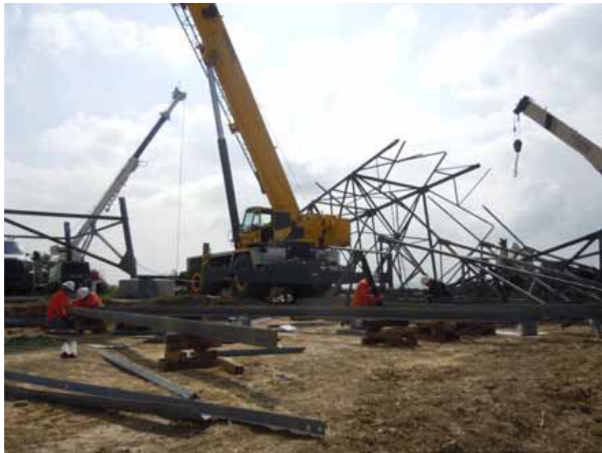
Figure 8: Crews assemble a tower, Segment 8, Phase 1.
