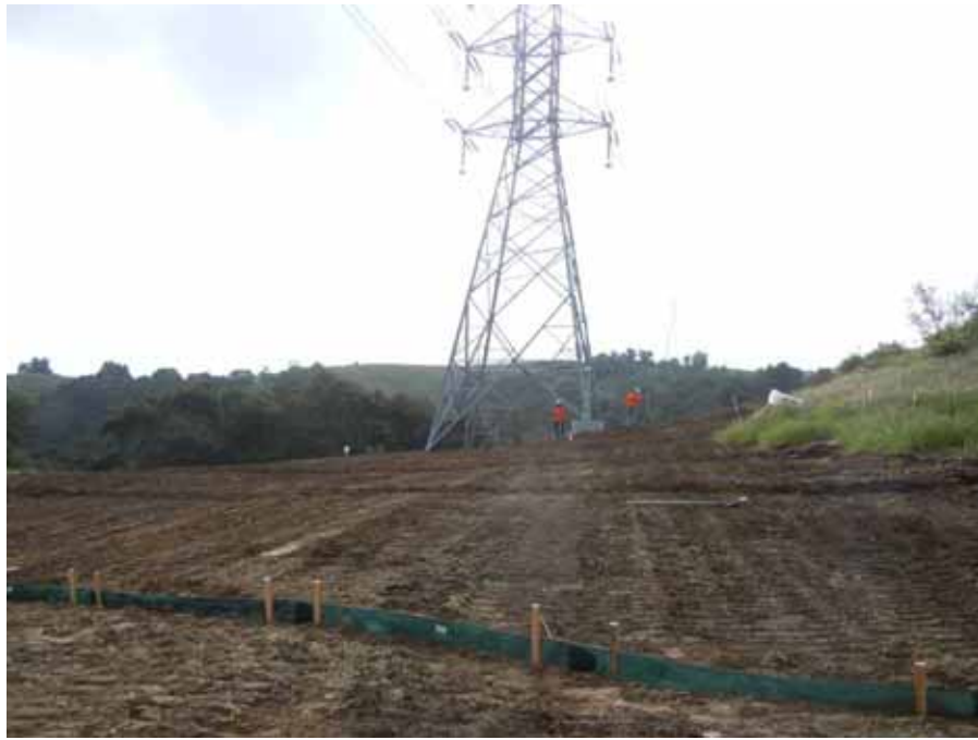
Figure 11: Wilson crews begin restoration at the Tonner Canyon shoo-fly, Segment 8, Phase 1.
