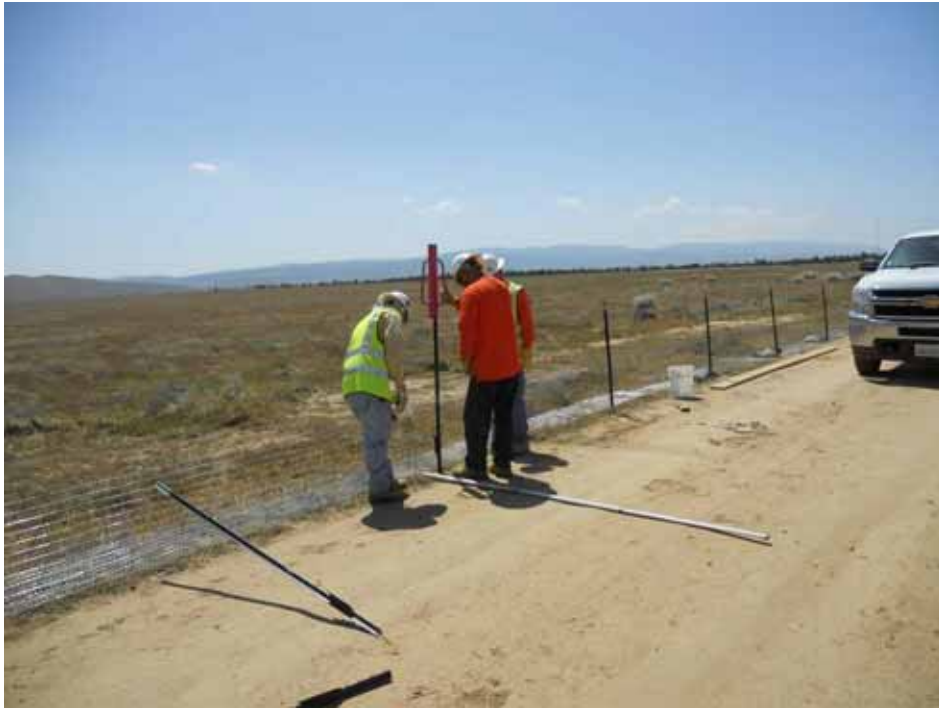
Figure 1: Tortoise fence installation (no-dig option) along Avenue C, Segment 4.
