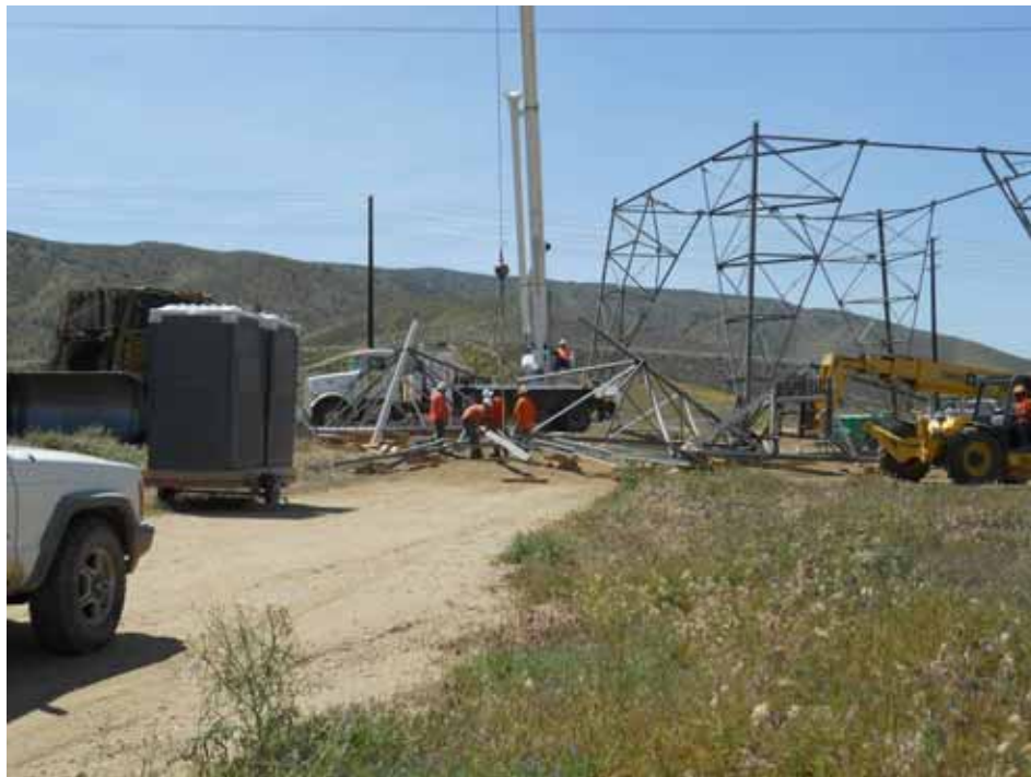
Figure 3: H&M steel crew assembling Tower 14, Segment 5.
