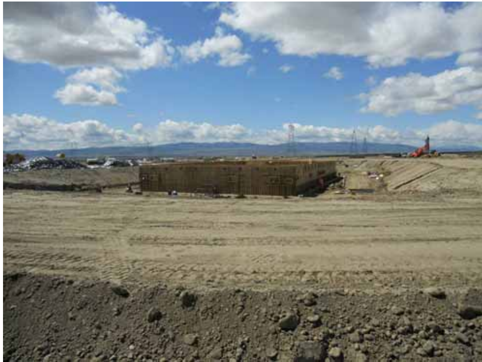
Figure 5: View of the MEER building inside the Whirlwind Substation, Segment 9.
