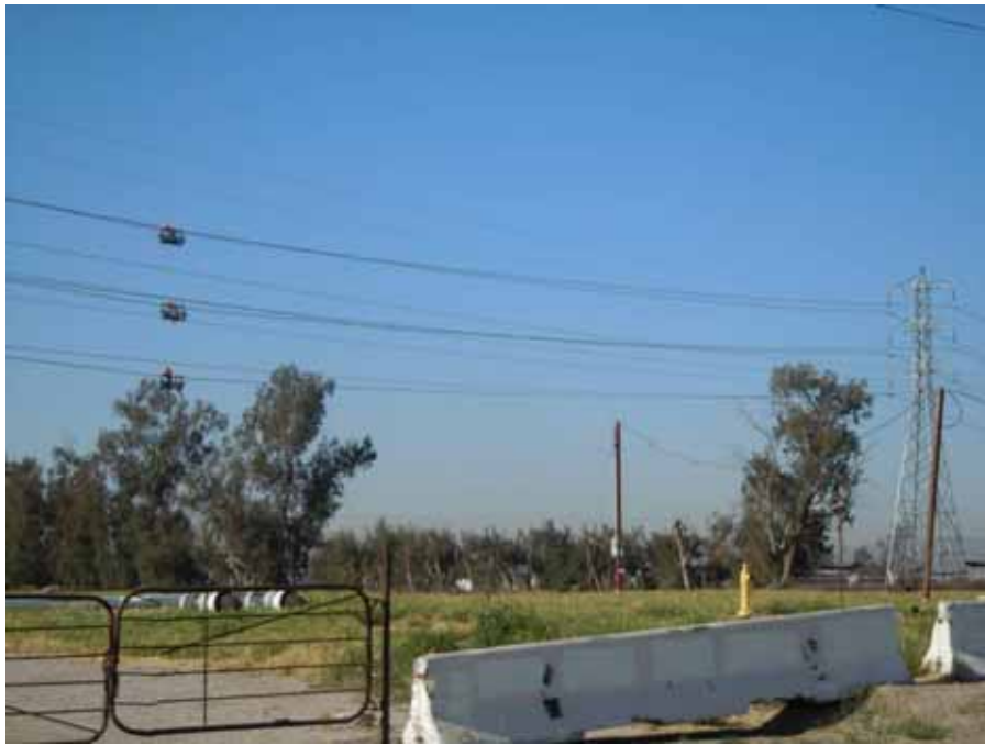
Figure 9: Crews install spacers along the Chino–Mira Loma No. 1 line, Segment 8, Phase 2.
