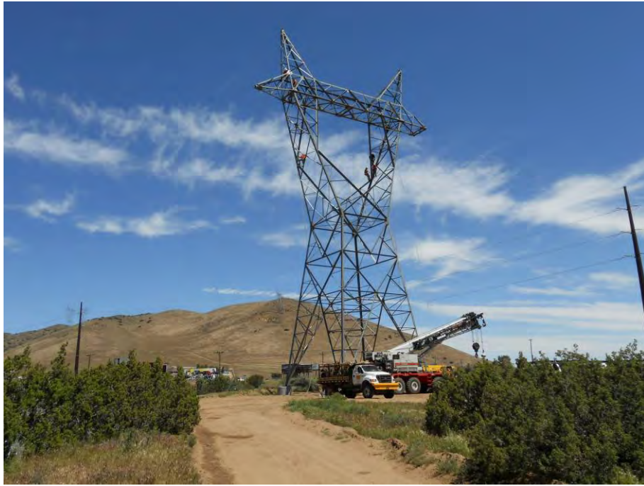
Figure 1: H&M steel crew assembling Tower 65, Segment 5.
