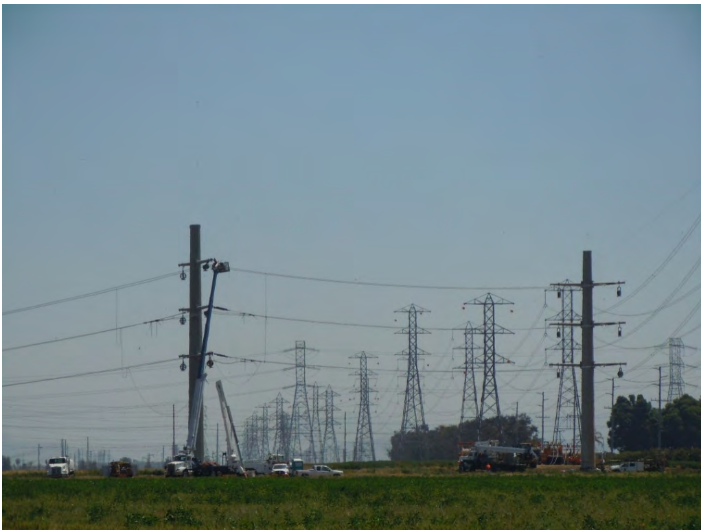
Figure 8: Crews string conductor, Segment 8, Phase 2.
