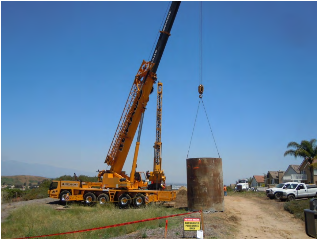
Figure 6: Crews move a casing for foundation drilling in Chino Hills, Segment 8, Phase 1.
