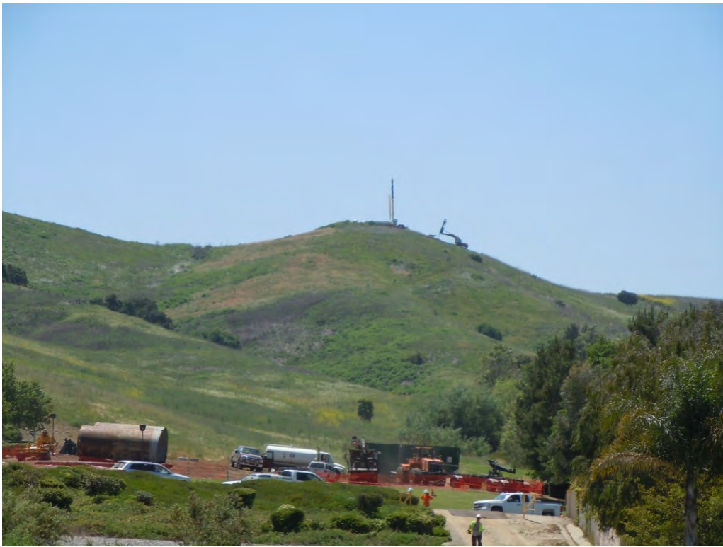
Figure 7: Crews drill foundations in the foreground and background in Chino Hills, Segment 8, Phase 1.
