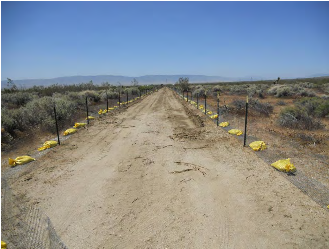
Figure 3: View of General Petroleum Access Road after grading was conducted, Segment 10.
