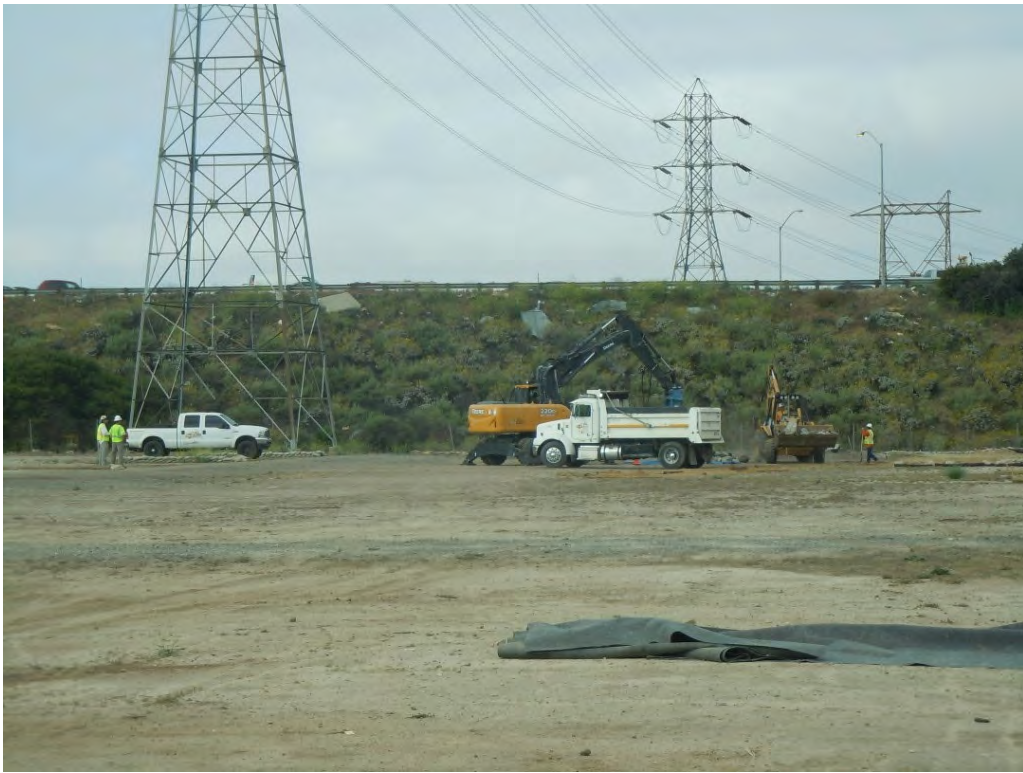
Figure 5: Crews remove a foundation in the City of Duarte, Segment 7.
