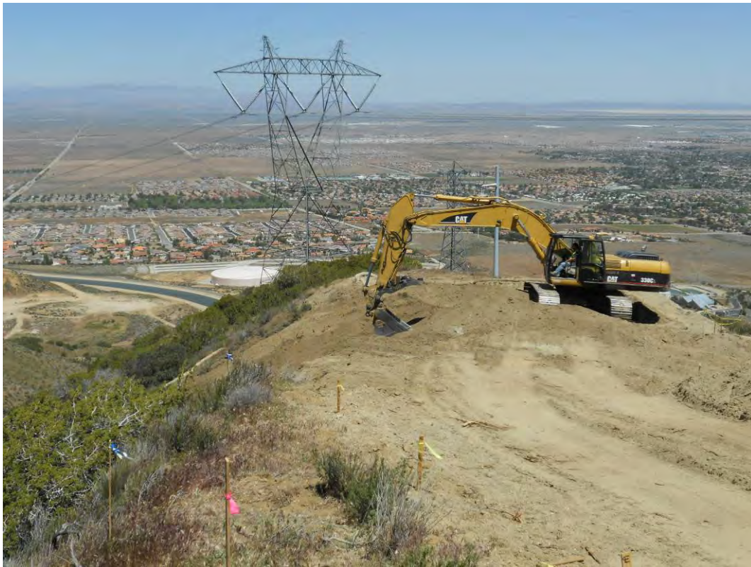
Figure 2: H&H Grading re-contouring Tower 20 pad site, Segment 5.
