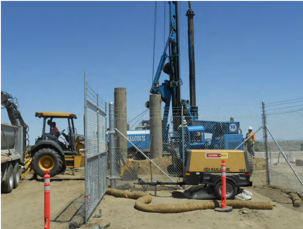
Figure 4: Bragg (drilling contractor) working on the underground bridge along 170 th Street outside Whirlwind Substation, Segment 9.
