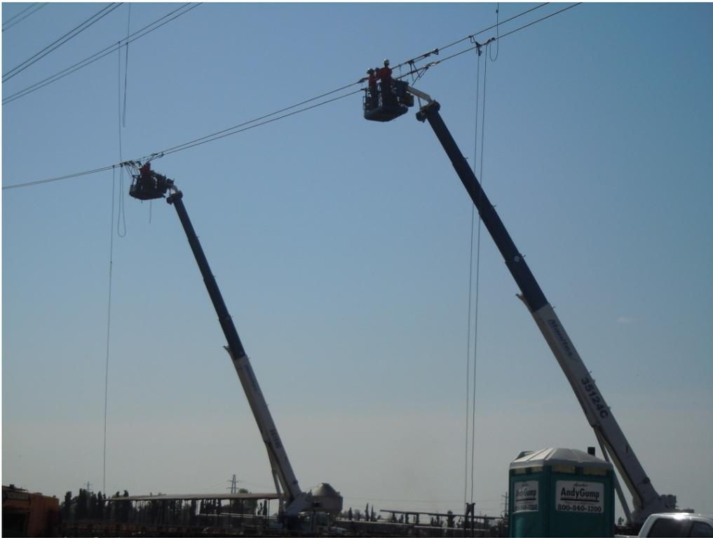
**Figure 7:** Crews install mid-span sleeves, Segment 8 Phase 2.
