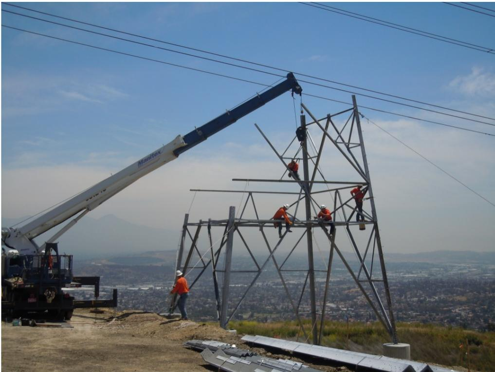
**Figure 8:** Crews assemble a tower, Segment 8, Phase 4.
