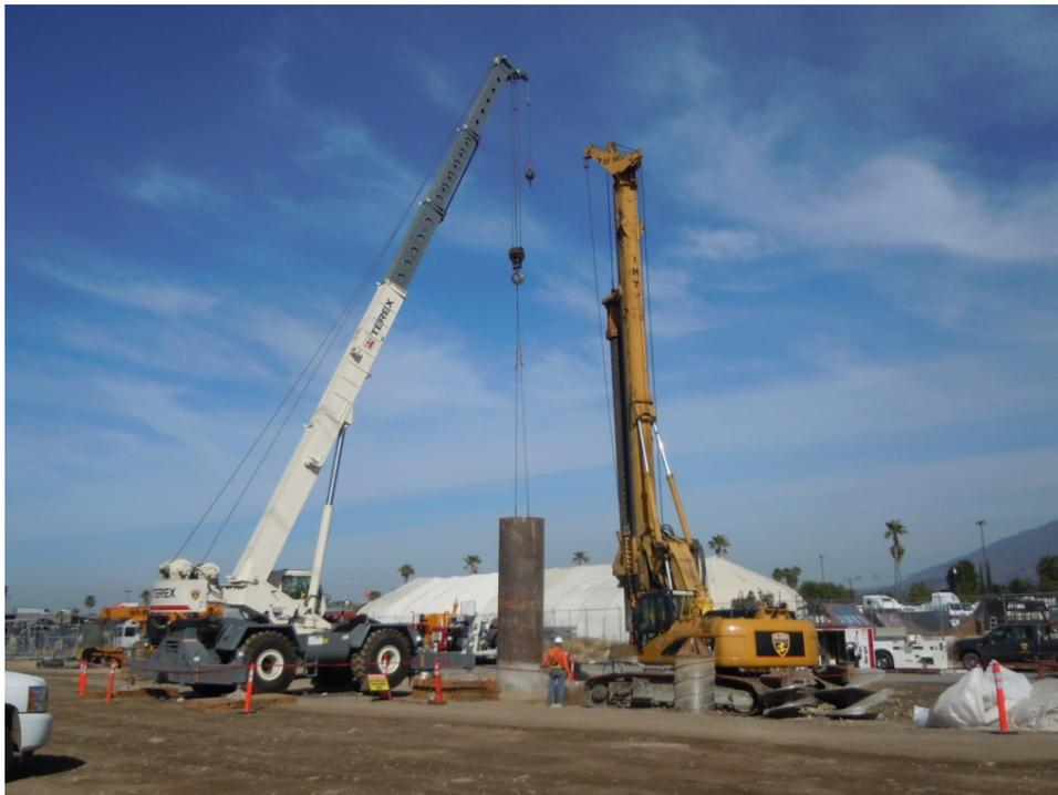
**Figure 6:** Crews set a casing for a tower foundation, Segment 7.
