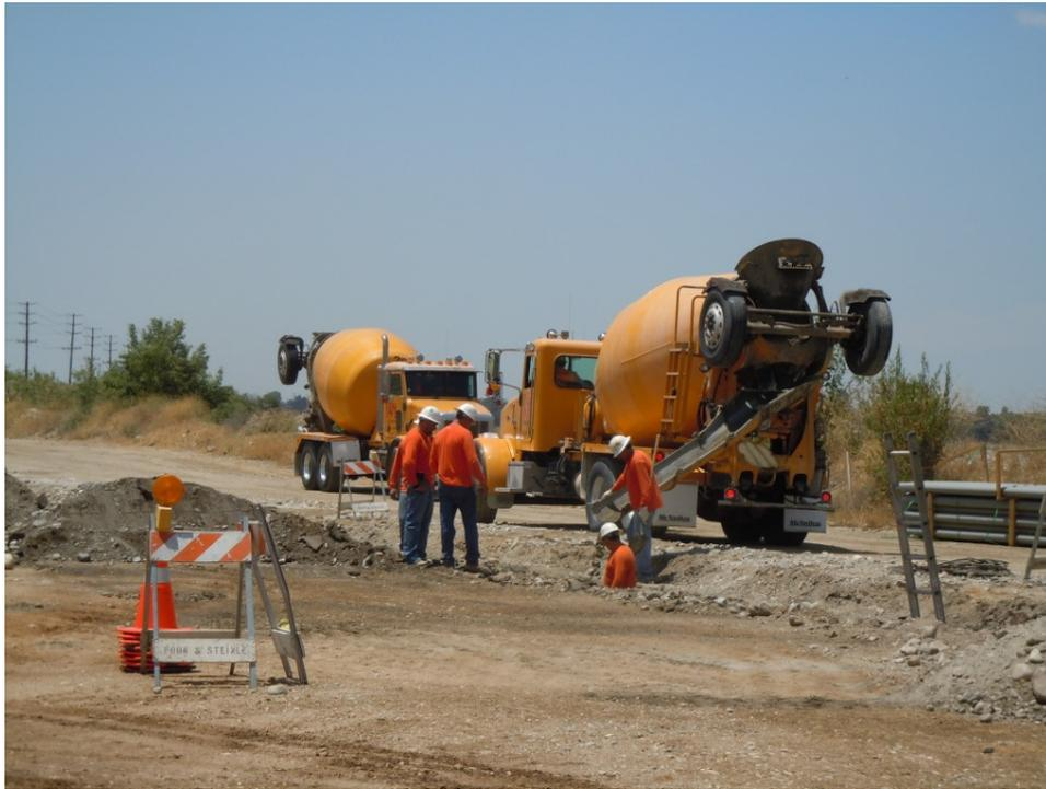
**Figure 5:** Wilson pouring concrete on the underground portion of the Rio Hondo–Amador-Jose-Mesa line, Segment 7, 66 kV.
