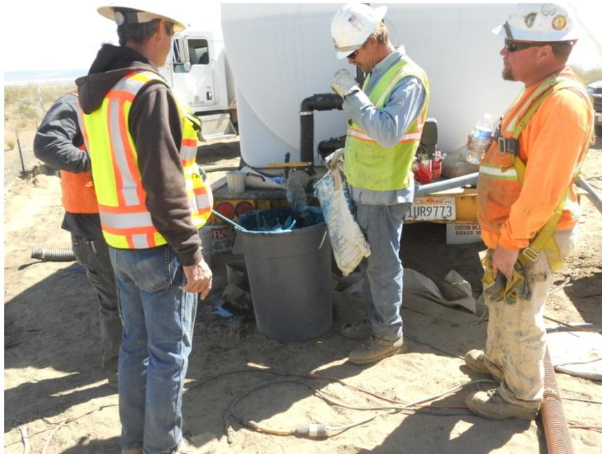
**Figure 2:** KV Structures mixing Revert Polymer with water at Tower M74-T1X, Segment 4.
