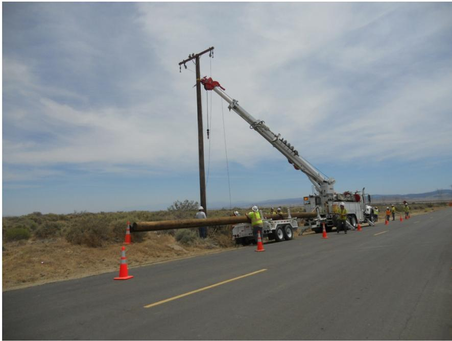
**Figure 3:** SCE setting a wood pole on the east side of 170<sup>th</sup> Street, Segment 10 Telecom.
