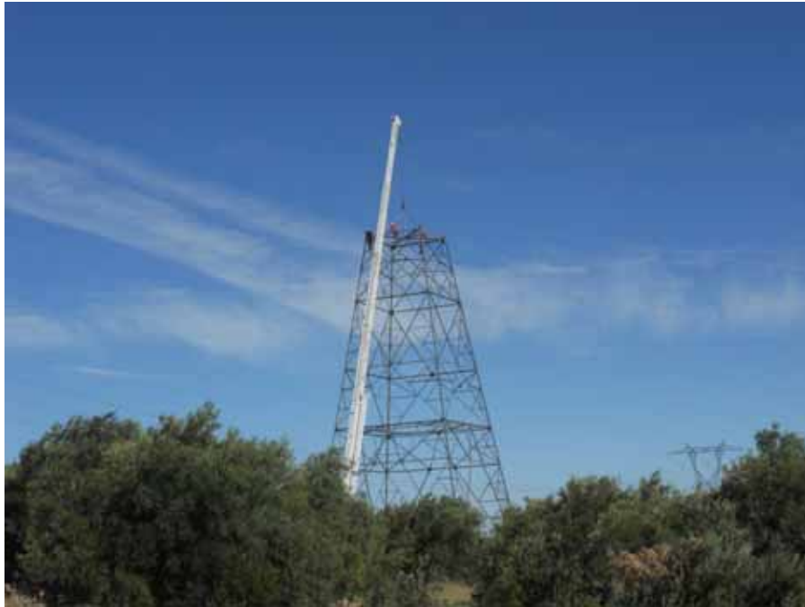
Figure 1: H&M steel crew erecting Tower 8, Segment 5.
