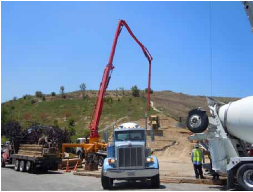
Figure 5: Crews pour concrete for a foundation, Segment 8, Phase 1.
