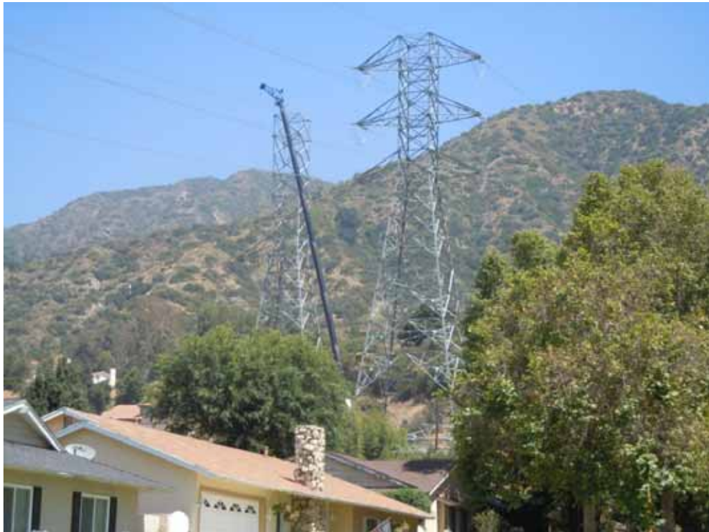
Figure 4: Crews assemble a tower in the City of Duarte, Segment 7.
