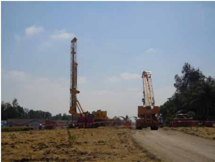
Figure 6: Tri-State mobilizes to a TSP foundation site, Segment 8 Phase 1.
