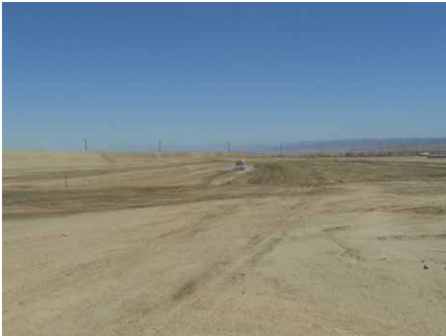
Figure 2: Water truck spraying for dust control in Whirlwind Substation, Segment 9.
