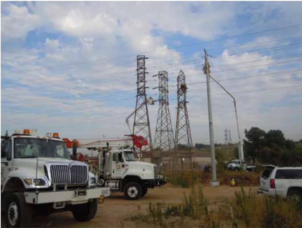
**Figure 7:** SCE crews work on a newly installed lightweight steel pole, Segment 7 66 kV.
