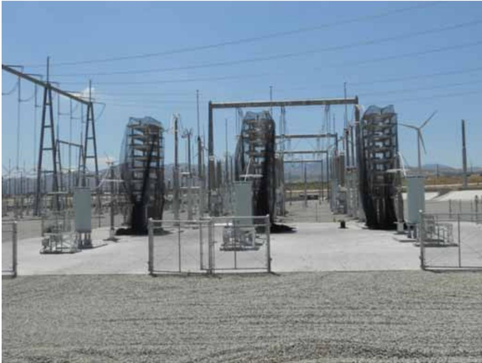
**Figure 1:** Bird netting covering capacitors in the Windhub Substation, Segments 1-3.
