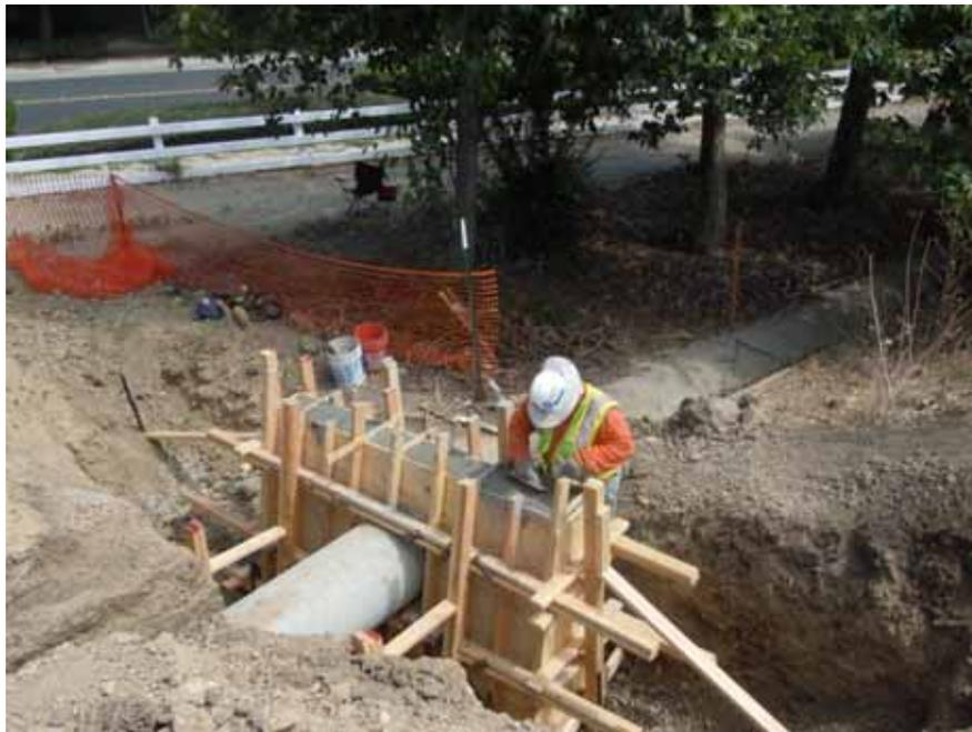
**Figure 8:** DCX installs a head wall, Segment 8, Phase 1.
