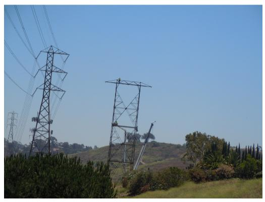
**Figure 6:** Crews disassemble a tower, Segment 8, Phase 4.
