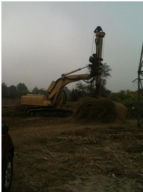
**Figure 6:** Foundation drilling of a 66 kV footing within Whittier Narrows.
