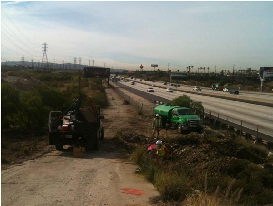
**Figure 5:** Foundation excavation of a 66 kV footing adjacent to the I-605 freeway.
