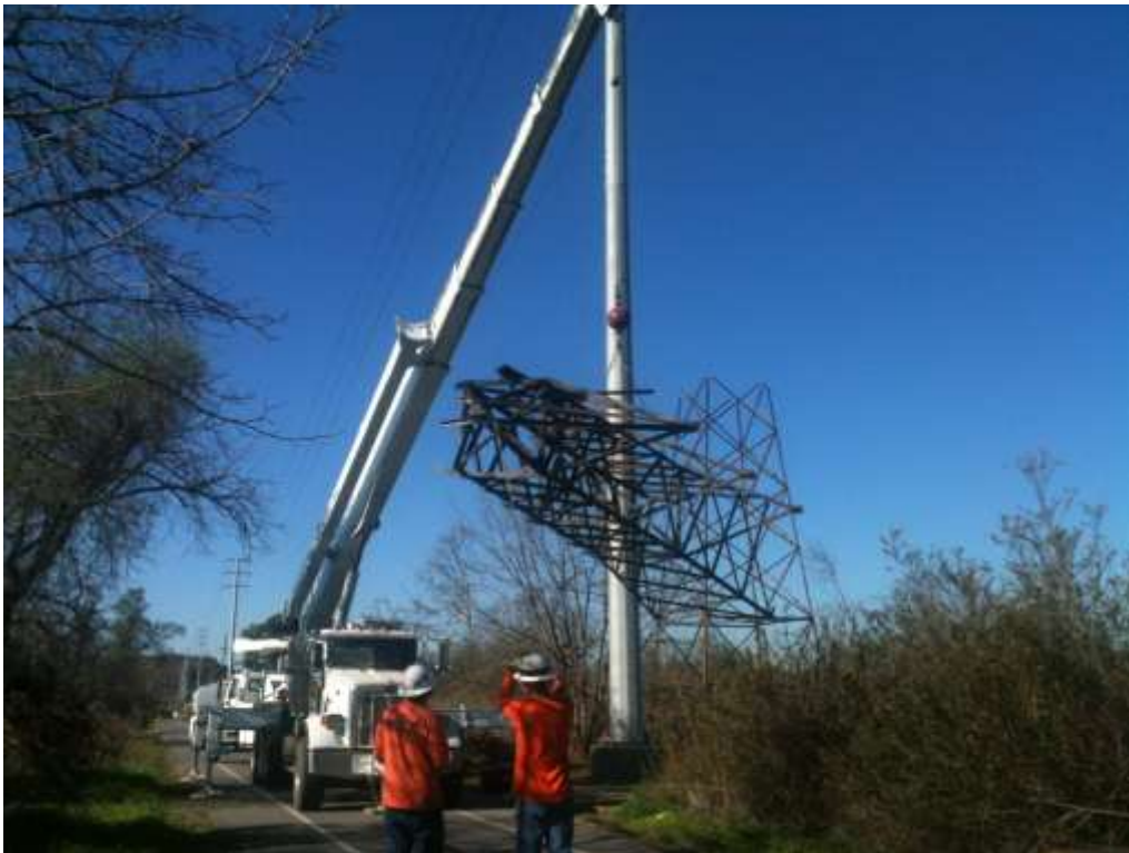
Figure 4: Crews remove a lattice steel tower along Siphon Road, Segment 8, 66 kV.
