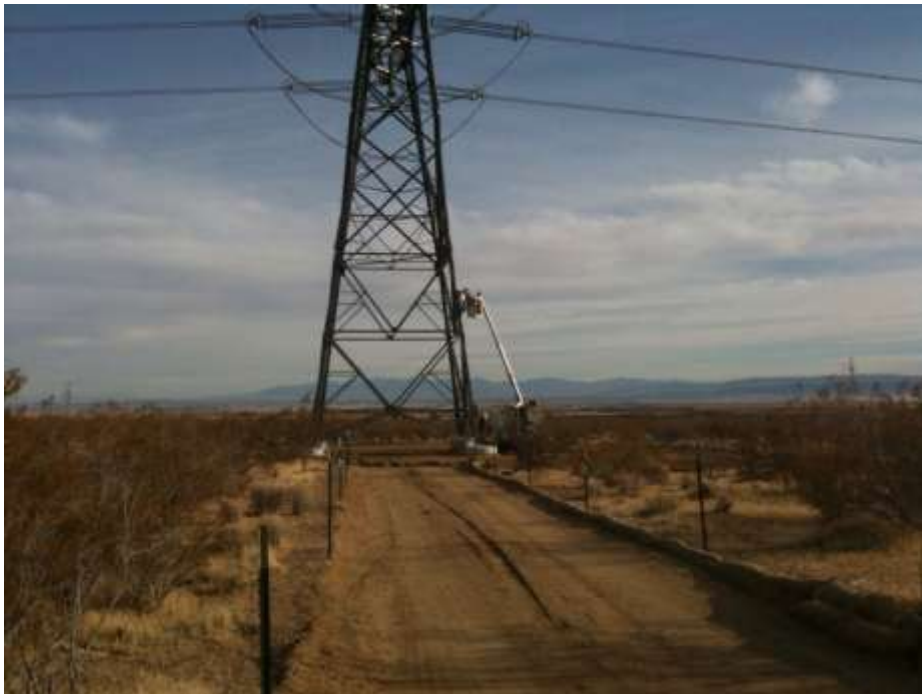
Figure 2: SCE splice crew at Tower 73, Segment 10.
