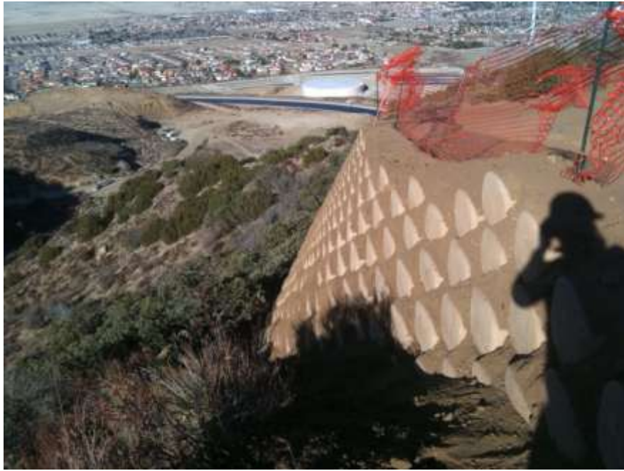
Figure 1: Completed retaining wall at Tower 19, Segment 5.
