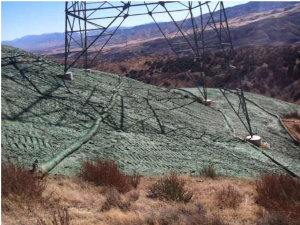
**Figure 4:** Hydro Straw and burlap fiber rolls applied to Tower 24, Segment 5.
