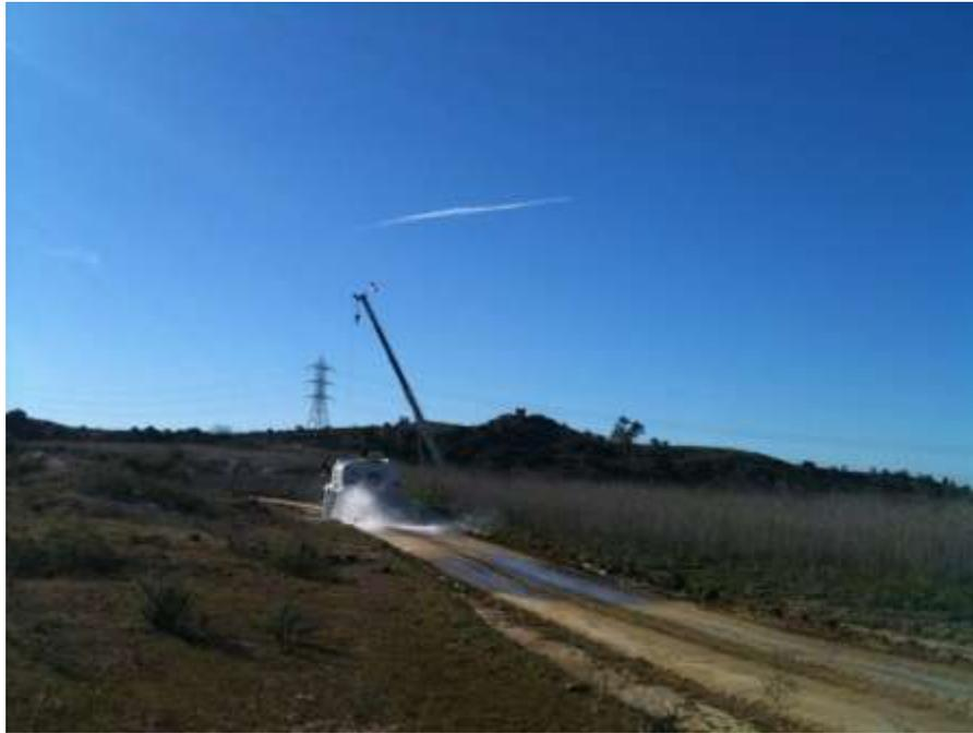
**Figure 5:** Dust abatement on an access road in Rose Hills, Segment 8 Phase 4.
