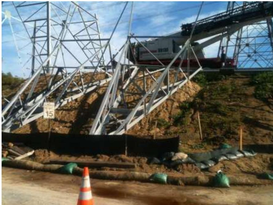
**Figure 6:** Failed BMPs after a rain event, Segment 7.
