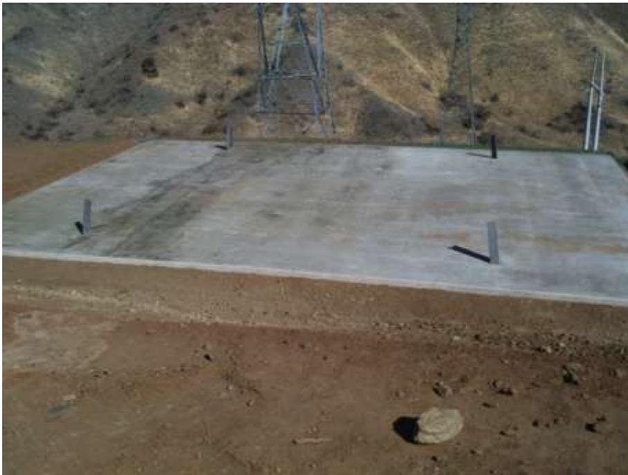
**Figure 2:** Concrete slab for the seismic foundation at Tower 30, Segment 5.
