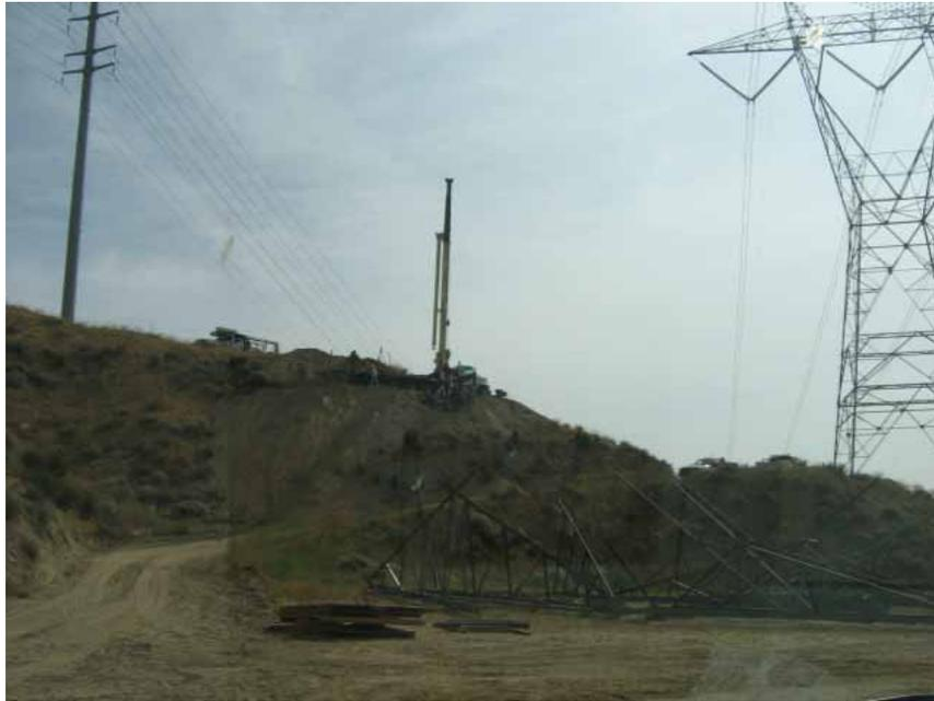
**Figure 1:** Foundation drilling at NC 7. Crews have already started assembling steel tower pieces seen in the foreground.
