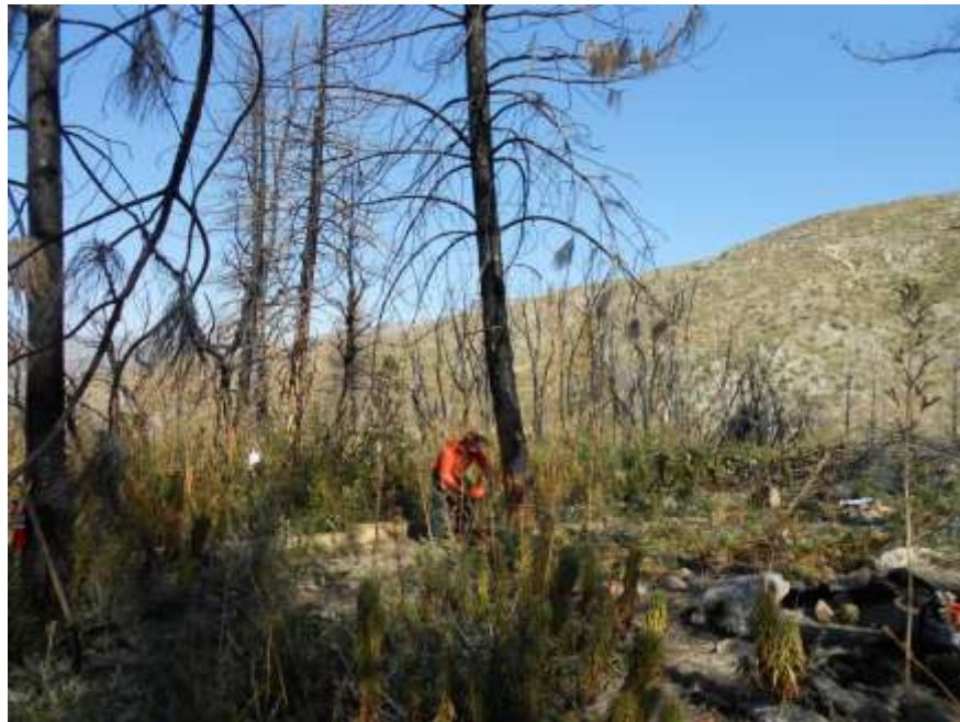
Figure 2: A vegetation clearing crew working on the new access road to Tower 69, Segment 6B.
