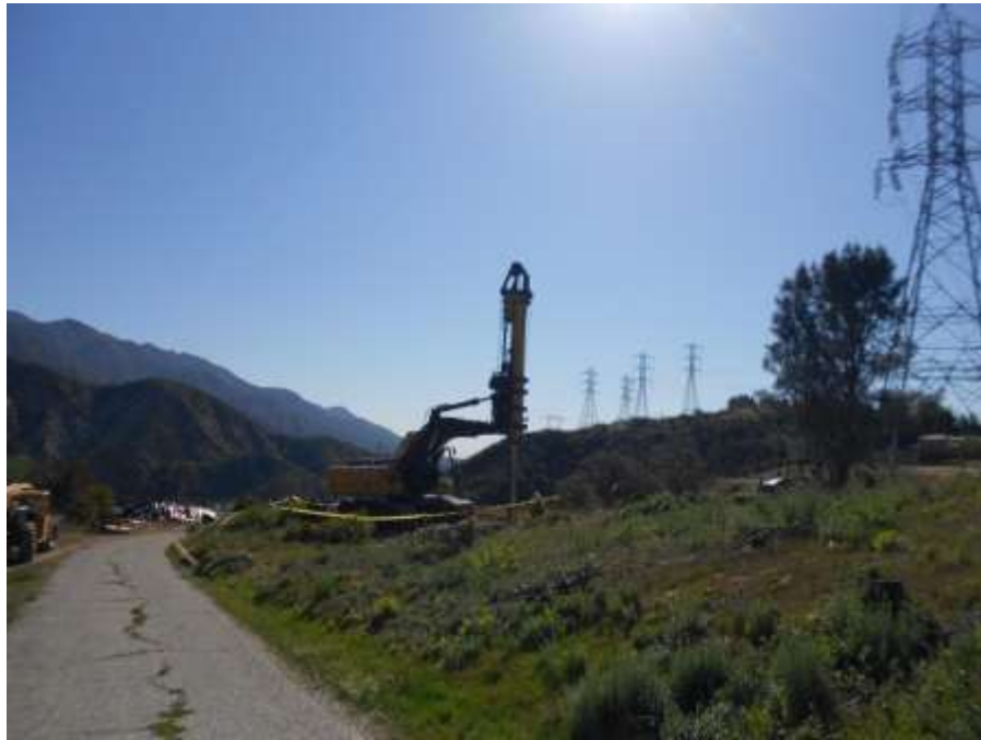
Figure 3: Newly established concrete washout and new structure foundation at Gould Substation, Segment 11D.
