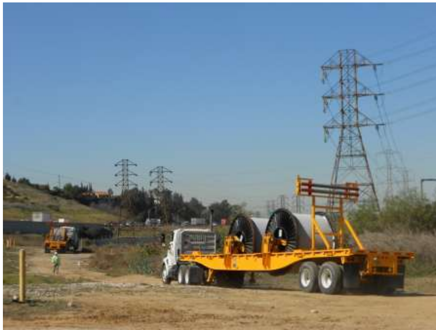
Figure 5: Stringing equipment being demobilized, Segment 7.
