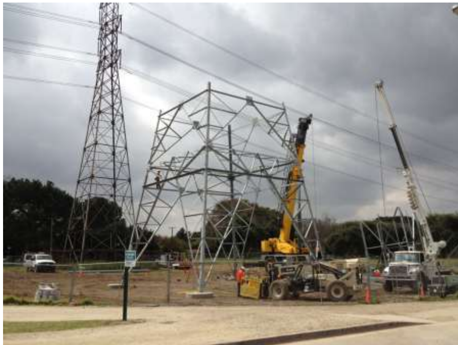
Figure 4: A crew assembles a tower in Legg Lake recreation area behind a fence to protect the public, Segment 7.
