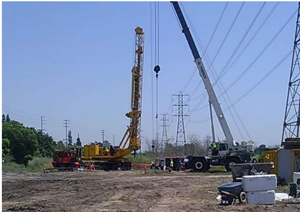
Figure 6: A crew drills a foundation, Segment 7.
