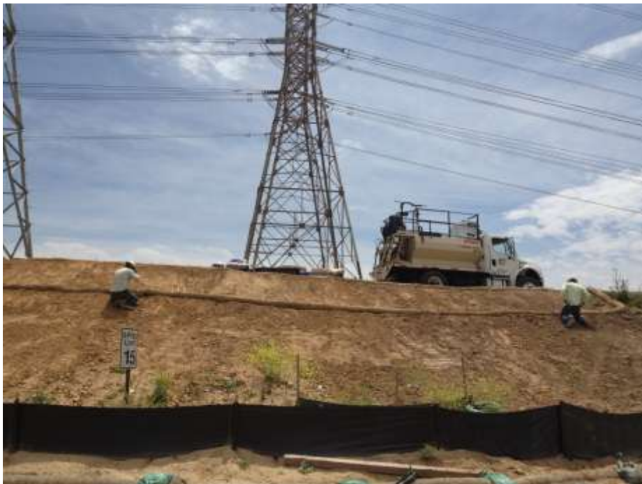
Figure 4: A Wilson crew installs fiber rolls prior to hydroseeding, Segment 7.
