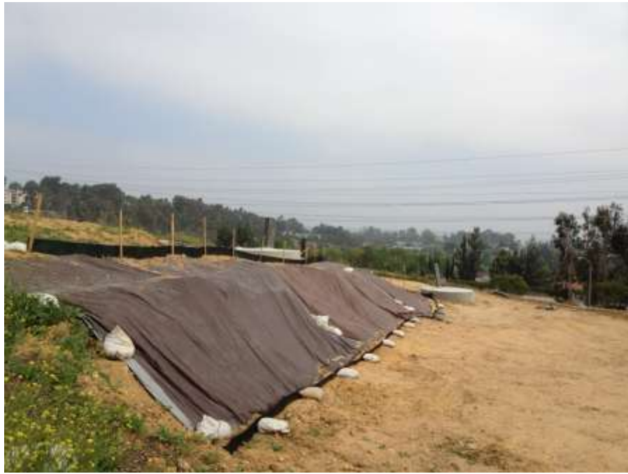
Figure 5: Newly installed BMPs, Segment 7.
