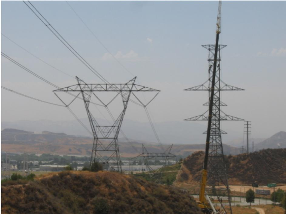
**Figure 1:** Between the Pardee Substation and the beginning of the Shoofly, the new 500 kV towers are being constructed in the center position of an existing SCE right-of-way. The towers on the left are currently supporting the Santa Clara-Vincent line, these towers will be dismantled and the conductor strung onto one side of the new double circuit towers.
