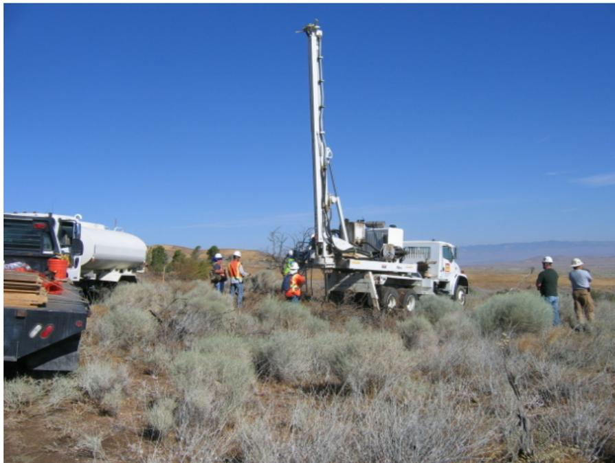
**Figure 4:** Drilling for the Hughes Lake Distribution Line near the California Aqueduct.
