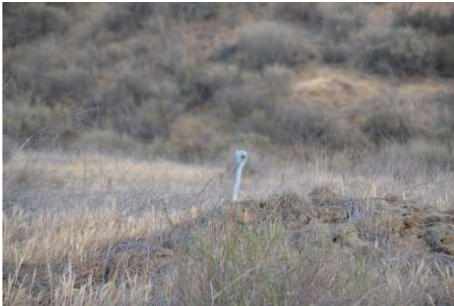
Figure 2: Anchor visible at the Haskell Canyon Segment 1 crossing location.
