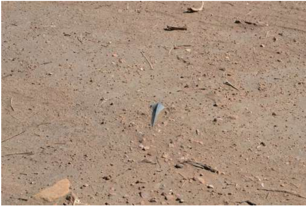
Figure 7: Pieces of steel from tower wreck-out at Aliso HAY were partially buried in many locations at the yard.
