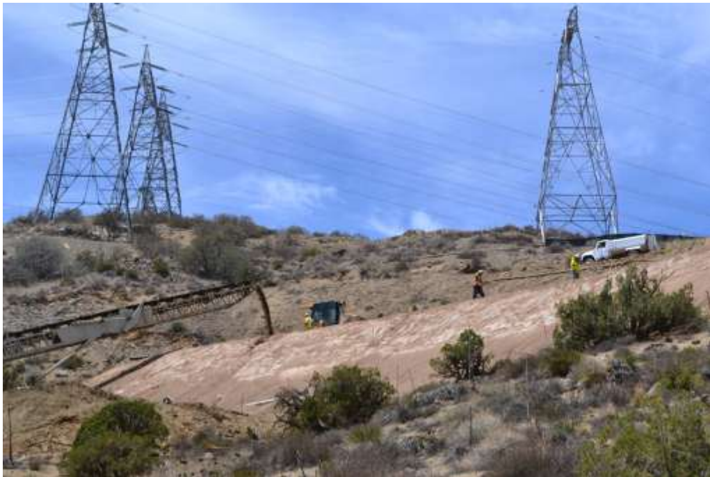
Figure 4: Dirt work continues at Structure 5 in Segment 6A.
