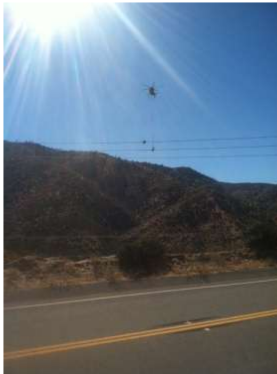
Figure 2: Wire stringing activities between Constructs 28 and 29 on Segment 6.
