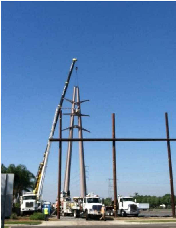
Figure 8: Tower demolition in Segment 8 Phase 3.
