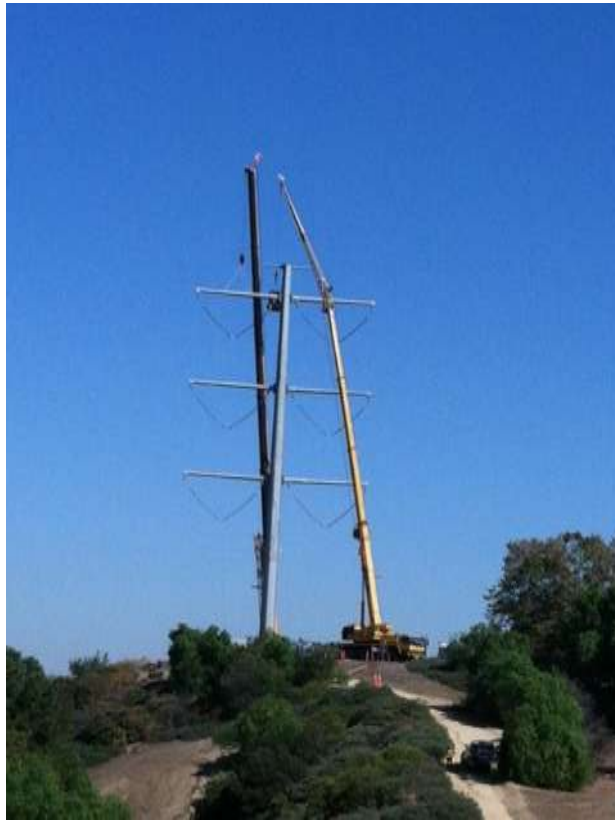
Figure 7: TSP demolition in Chino Hills, Segment 8.
