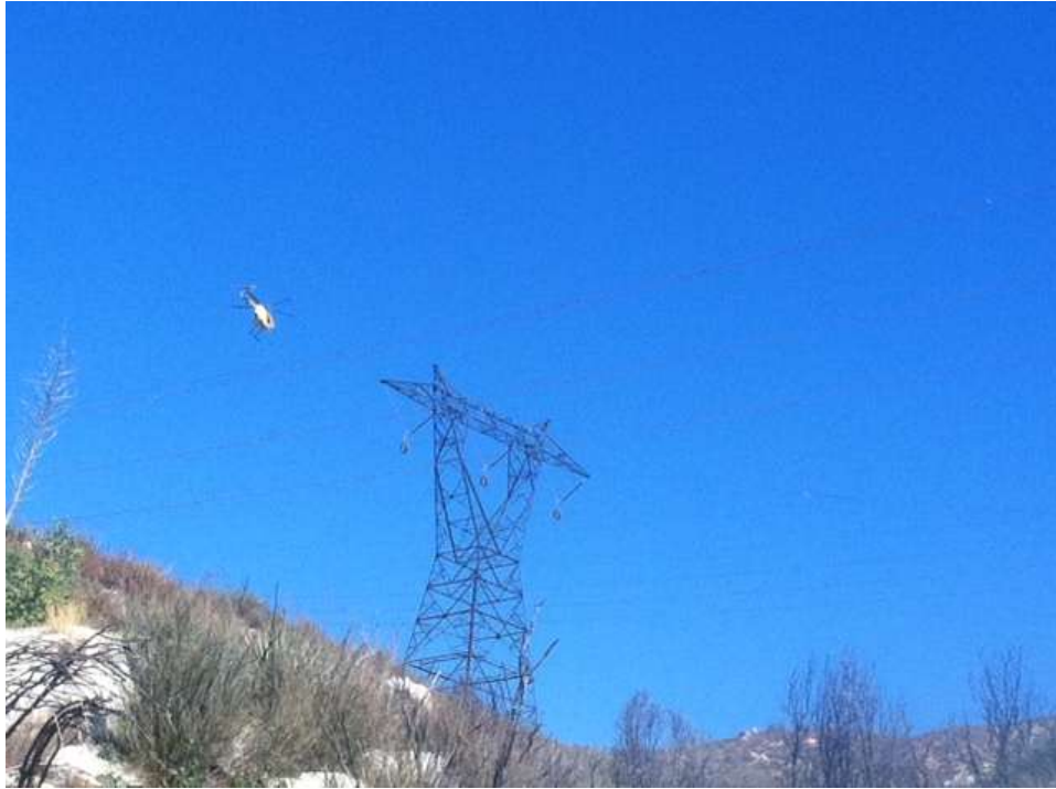
Figure 1: Wire stringing operations between Constructs 61 and 62 on Segment 6.
