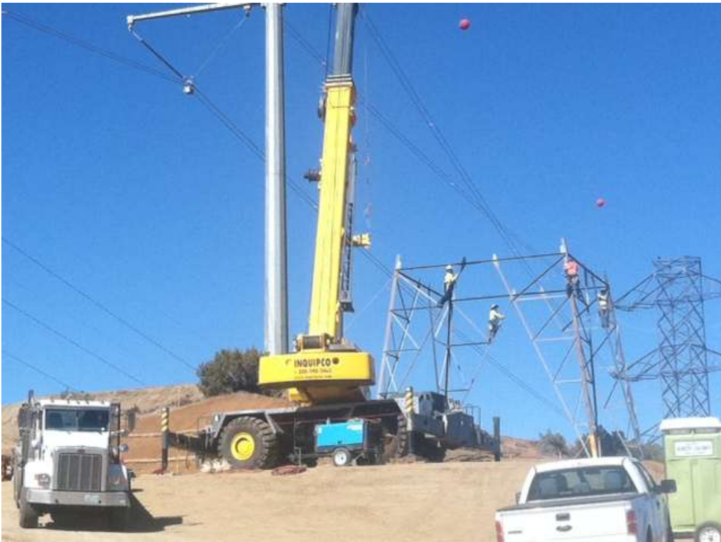
Figure 3: Tower wreck-out activities at Construct 3 on Segment 6.
