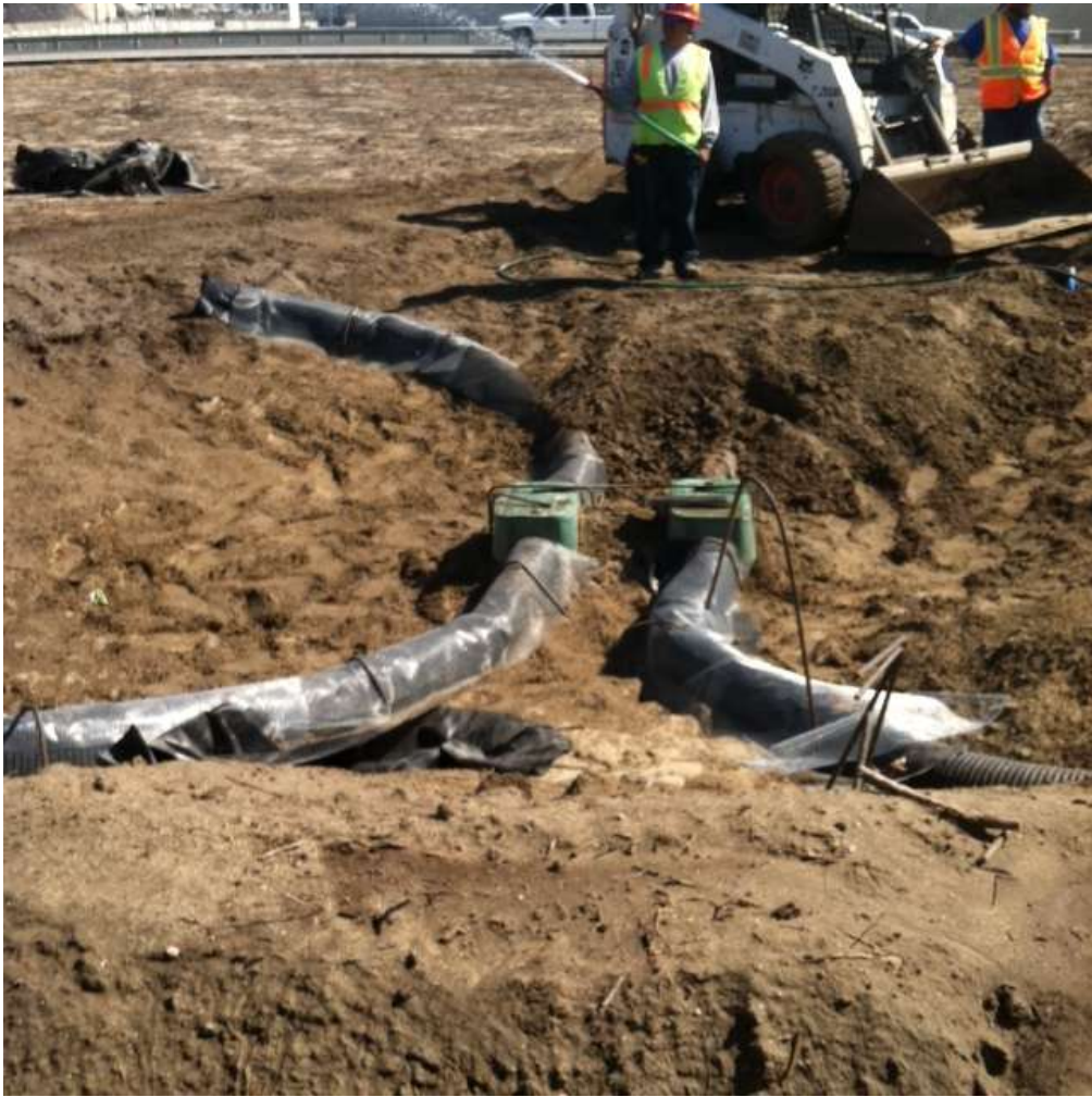
Figure 9: Artificial burrow installation near Rancho Vista Yard for burrowing owl relocation.
