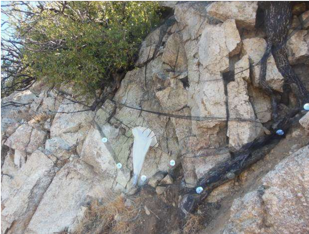
Figure 5: Bat exclusionary netting installation completed near Construct 30 along Segment 11C (FRED ID #217).
