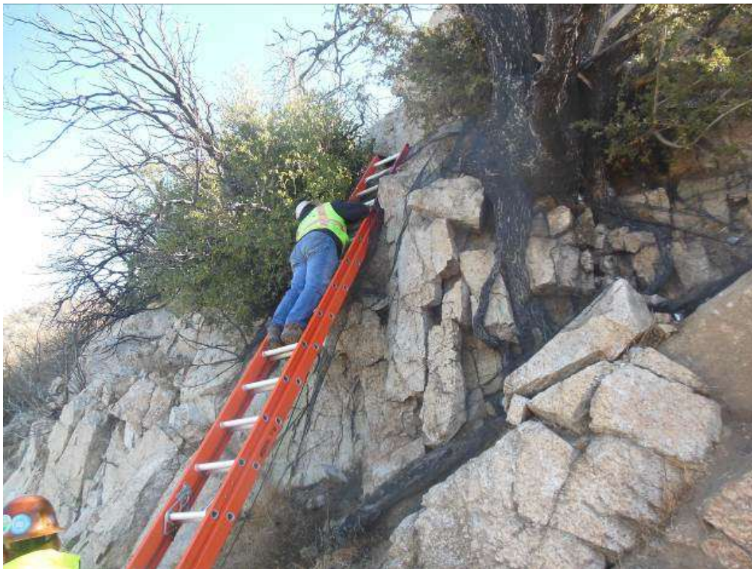
Figure 4: Installation of bat exclusionary netting near Construct 30 along Segment 11C (FRED ID# 217).
