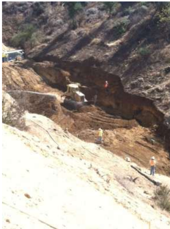
Figure 6: Road construction in Tonner Canyon to Tower M57-T1.
