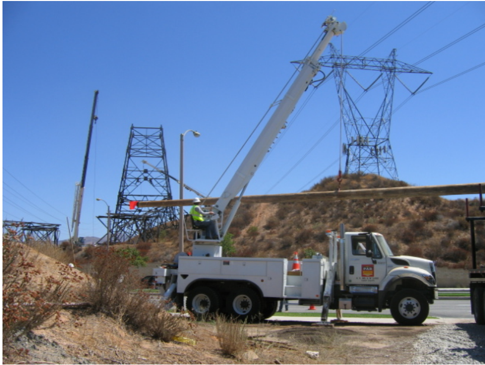
Figure 1: Guard pole installation along McBean Parkway near NC 11.
