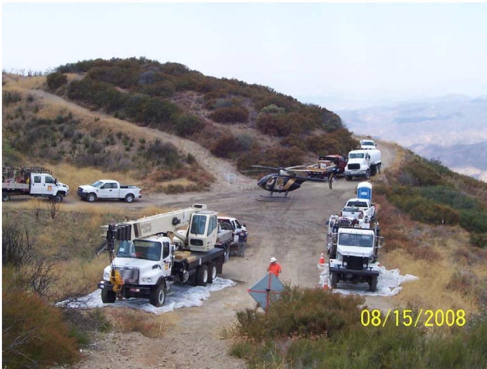
Figure 5: Crews staging equipment and materials along Del Sur Ridge Road within Section 2, on the ANF.
