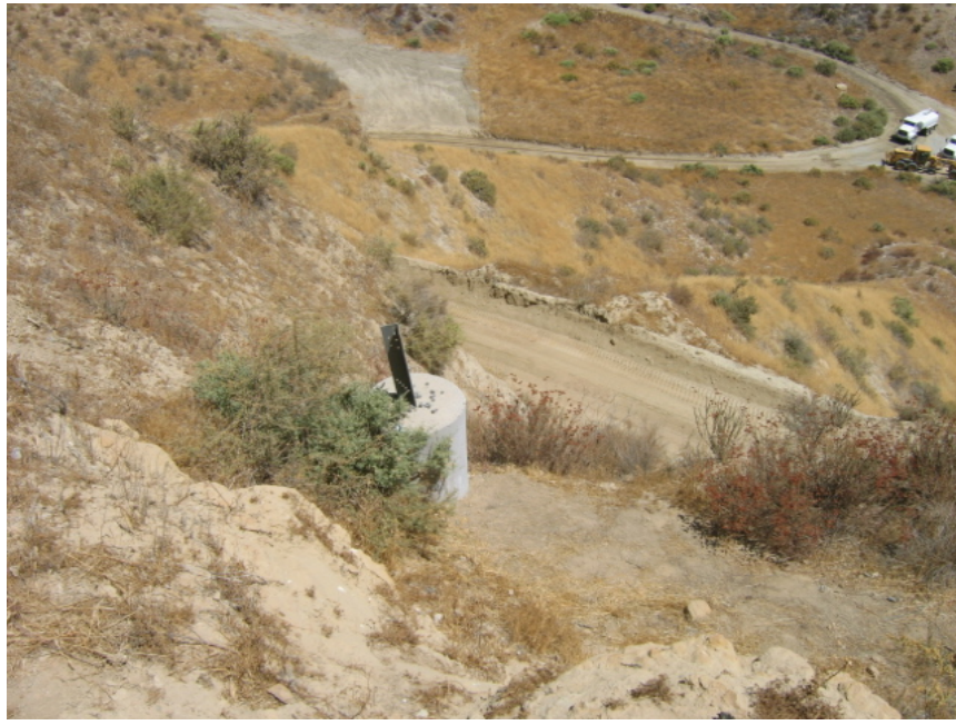
Figure 3: A foundation at the site of wreck out Tower 24/2 is proposed to be left in place, due to slope failure concerns if removed. A Variance Request was approved by CPUC to leave the footing in place.
