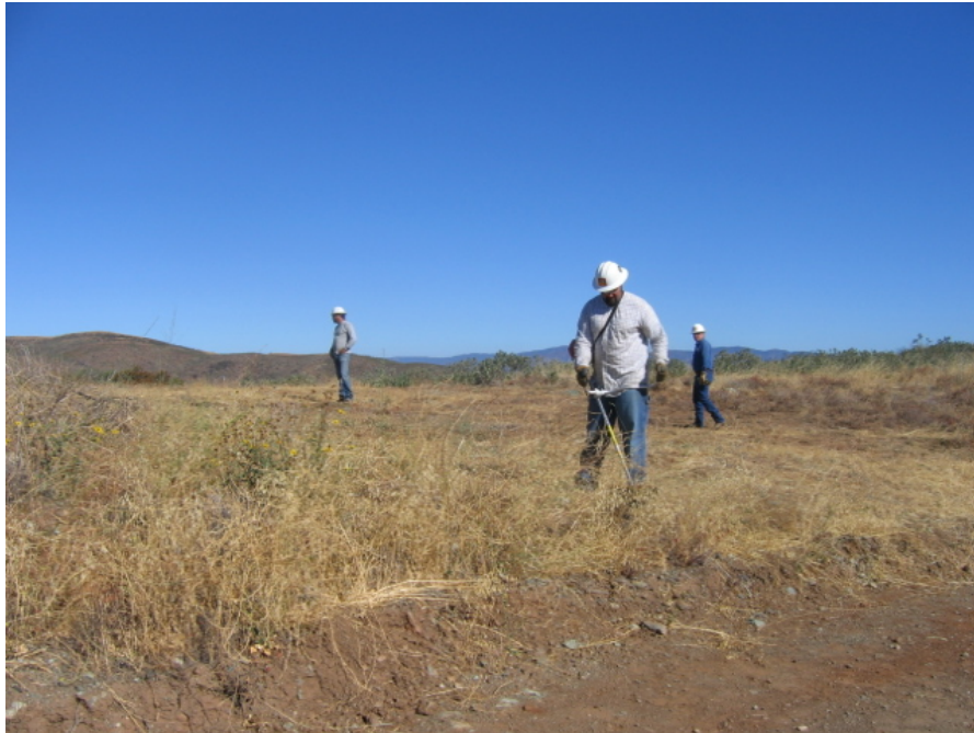
Figure 4: Vegetation clearing at a helicopter landing zone along Del Sur Ridge Road on the ANF.
