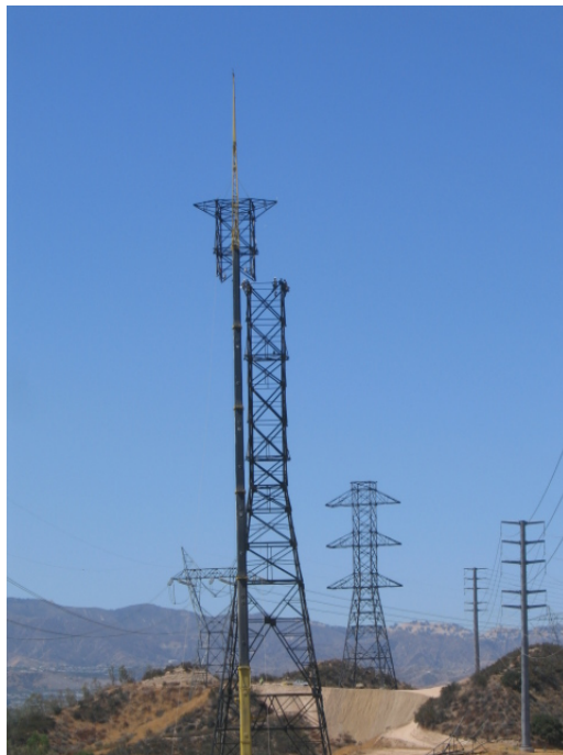
Figure 2: Tower erection near McBean Parkway in Section 1.
