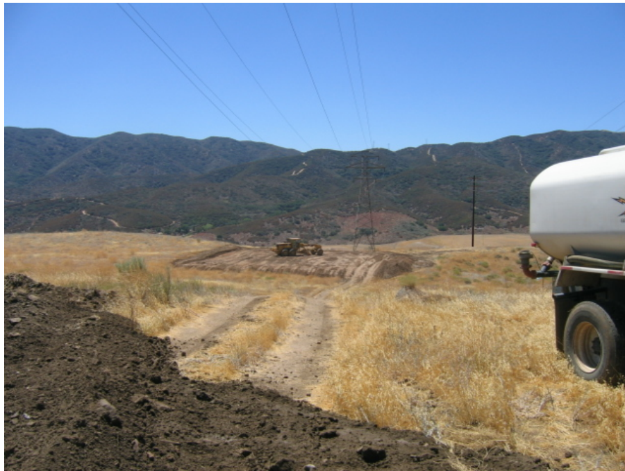
Figure 7: Section 3 construction of crane pads and roads near Elizabeth Lake Road.
