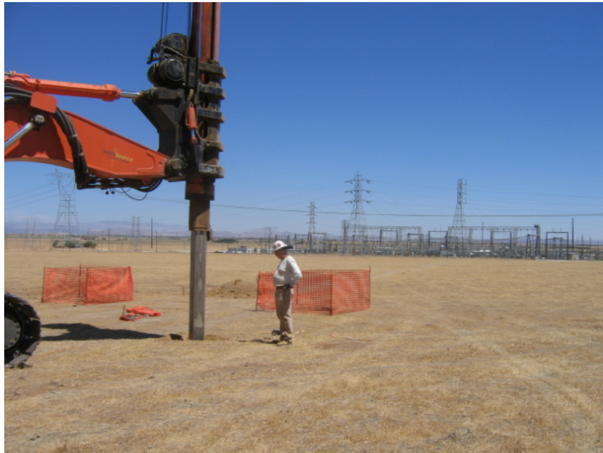
Figure 6: Section 3 construction on foundations near the Antelope Substation.
