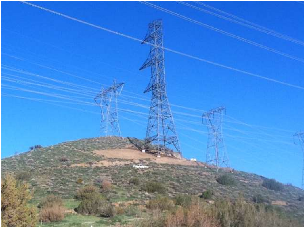
Figure 1: Grading activities occurred at Construct 3, Segment 11C.
