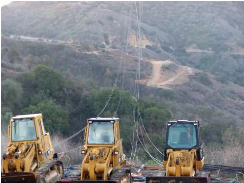
Figure 6: On March 18 and 19, Biological Monitors observed the conductor between Towers M6-T2 and M6-T3 dropping several times onto California walnut trees, coast live oak trees, and Laurel sumac bushes during wire stringing activities on Segment 8, Phase 4. This area is outside of approved disturbance limits and within designated critical habitat for coastal California gnatcatcher. The area disturbed was surveyed and several branches of the trees were broken.
