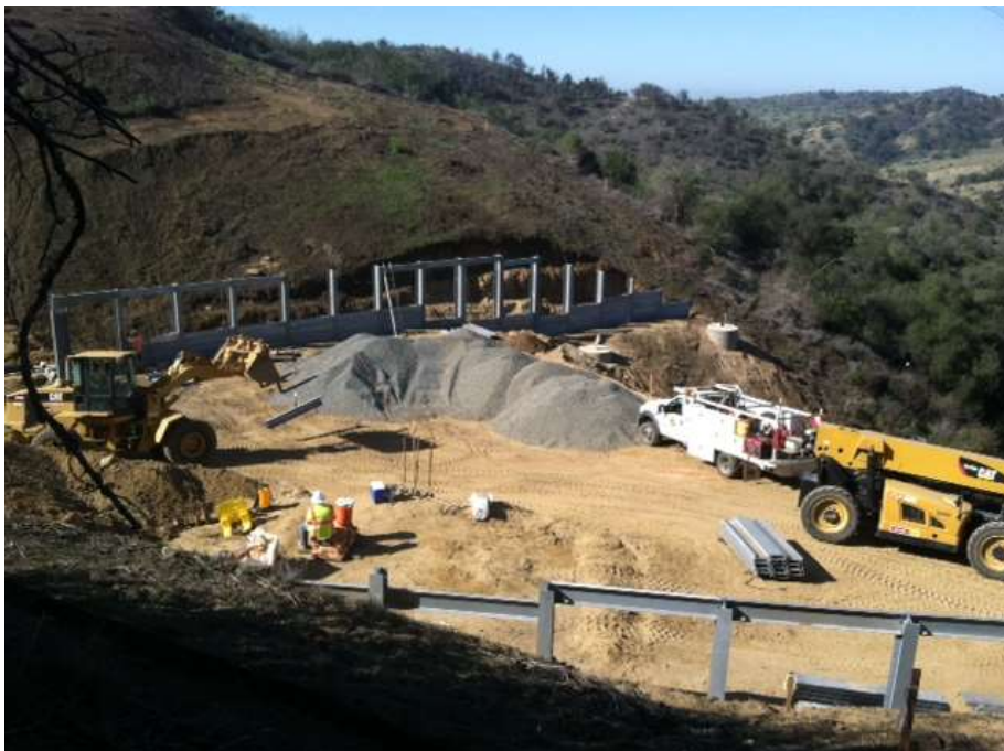
Figure 4: Union Construction crews continued road grading, retaining wall installation, and importing drain rock at Tower M57-T1, Segment 8, Phase 1.
