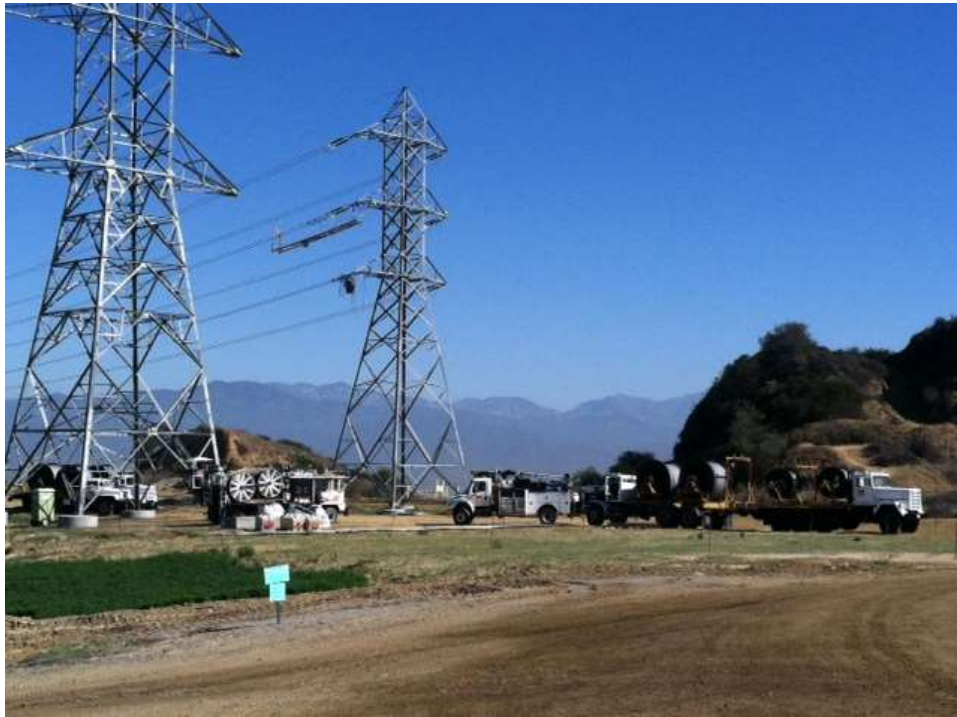
Figure 5: Wire stringing activities in Rose Hills, Segment 8, Phase 4.
