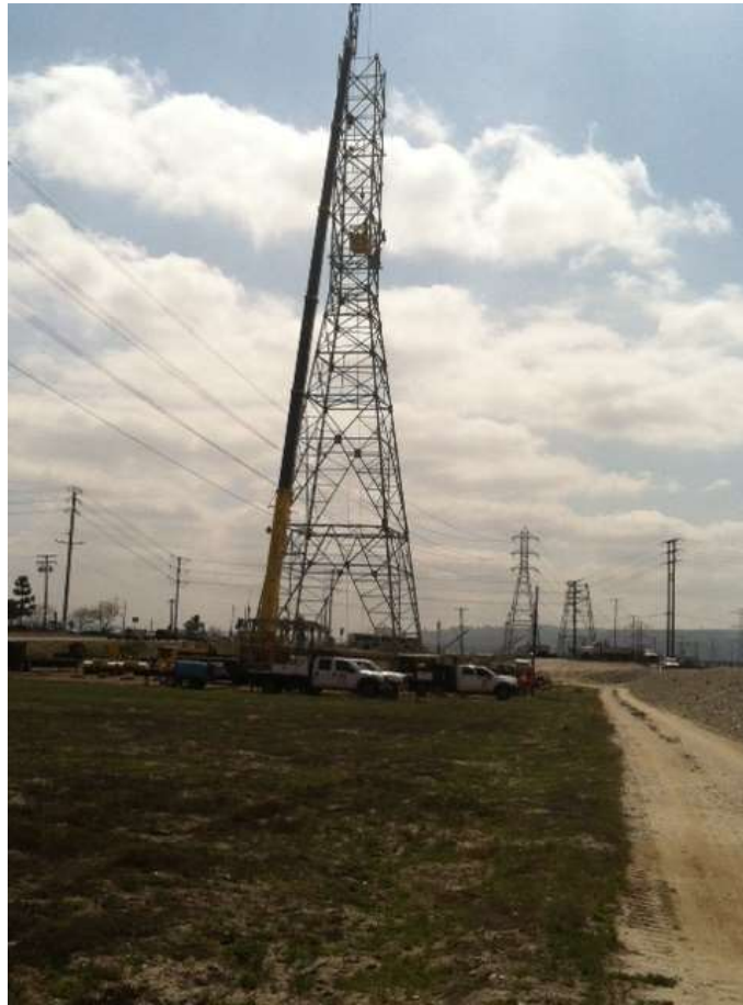
Figure 3: Tower assembly at Tower M34-T2, Segment 7.
