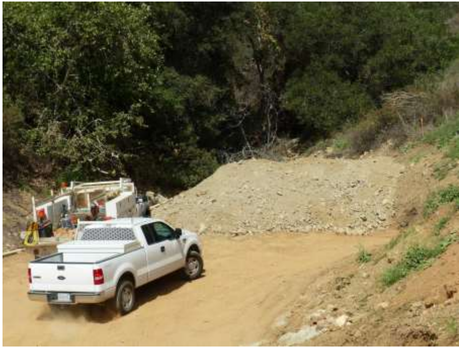
Figure 7: On March 20, a Biological Monitor observed a large pile of dirt stockpiled in JD ID 7-3-S-1 along the access road to Tower M27-T3, Segment 7. Photo courtesy of FRED.
