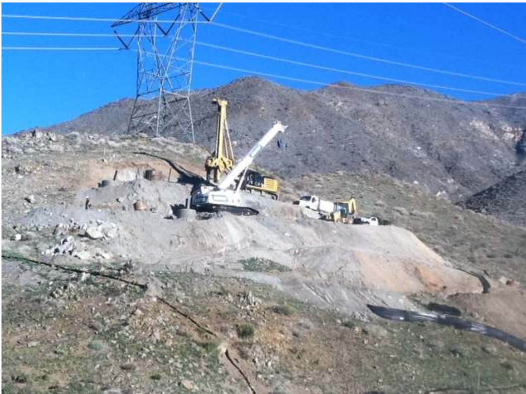
Figure 2: Foundation activities occurring at Construct 11X, Segment 11C.
