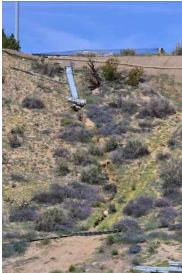
Figure 2: BMPs were installed surrounding the work area for Tower 1, Segment 6.
