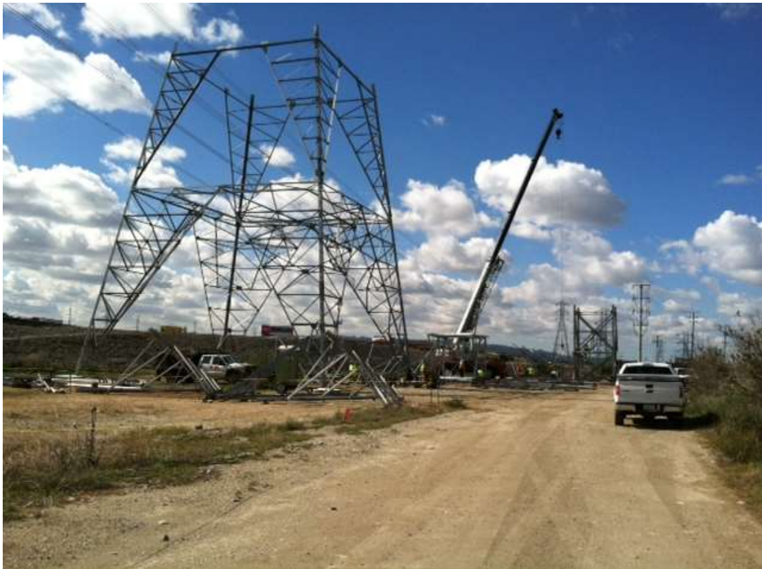
Figure 6: Tower assembly at Tower M32-T4, Segment 7.
