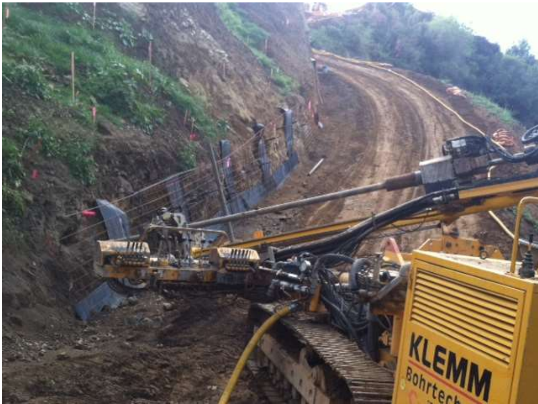
Figure 5: Soil nail wall installation at Tower M27-T3 in Duarte, Segment 7.
