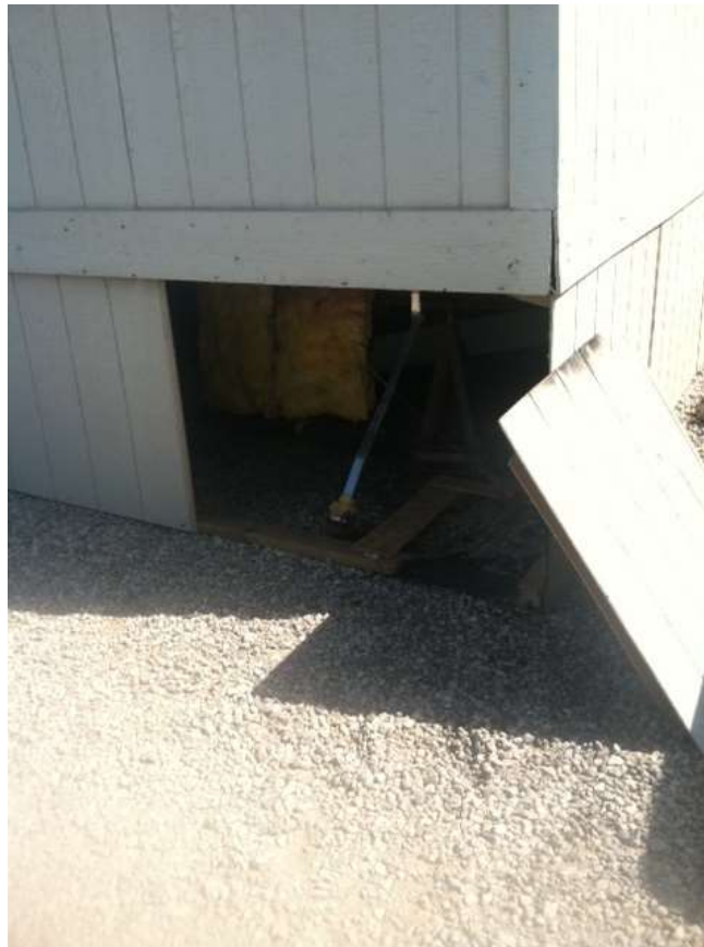
Figure 6: Vincent North Material Yard construction trailer area that was burned.
