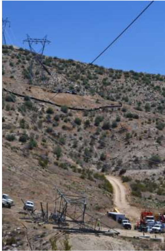
Figure 1: Wire removal activities at Construct 12, Segment 11C.
