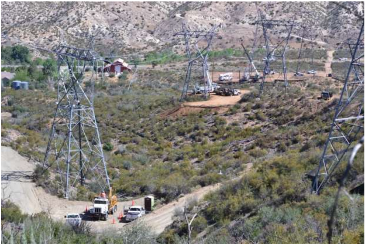
Figure 4: Wire removal activities at Constructs 16 and 17, Segment 11C.
