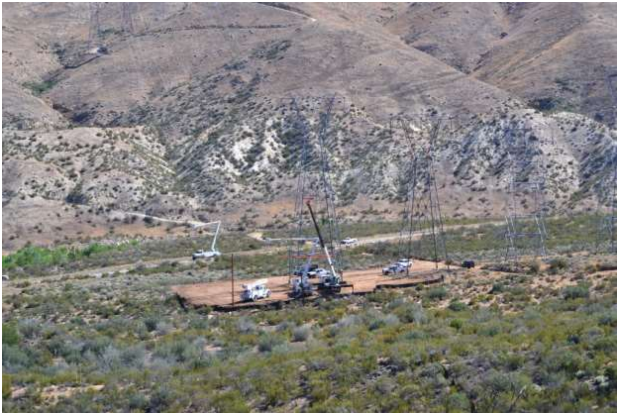
Figure 3: Wire removal activities at Construct 15, Segment 11C.
