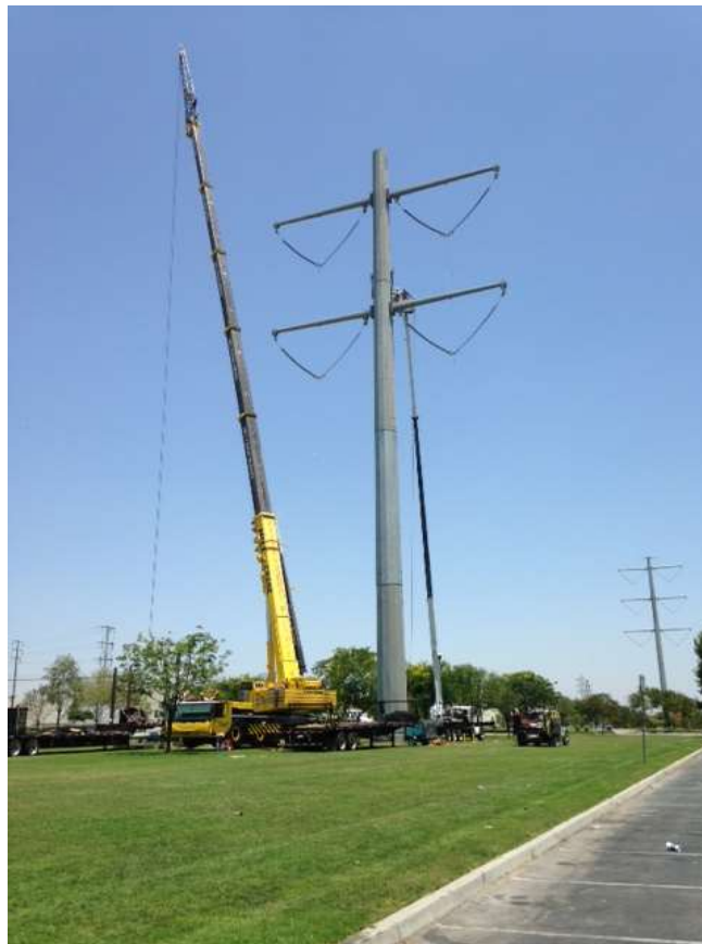
Figure 8: Assembly of Tower M66-T8 in the City of Chino, Segment 8, Phase 3.
