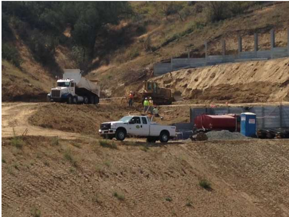
Figure 7: Soil import for road construction to Tower M57-T1 in Tonner Canyon, Segment 8, Phase 1.
