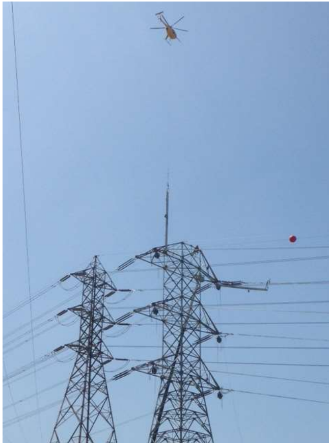
Figure 10: Helicopter activities during wire stringing installation at Tower M44-T1, Segment 8, Phase 4.
