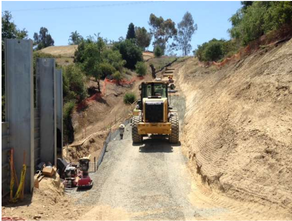
Figure 9: Hilfiker wall and grading activities continue at Tower M49-T1, Segment 8, Phase 4.
