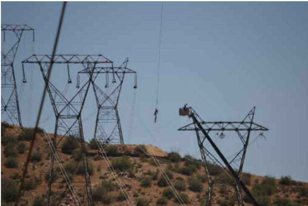
Figure 2: Wire removal activities at Construct 12, Segment 11C
