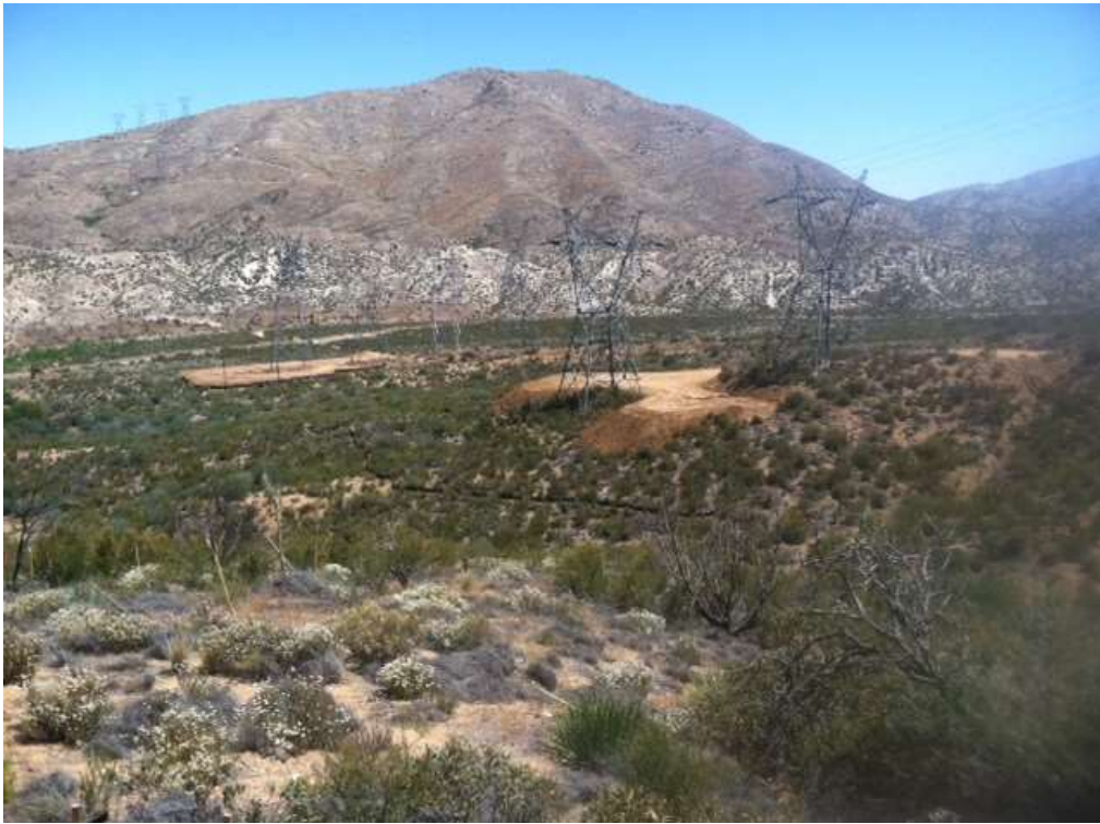
Figure 5: BMP installation at Constructs 15 and 16, Segment 11C.
