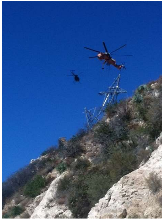
Figure 3: Tower erection activity with Air Crane at Construct 57, Segment 11C.
