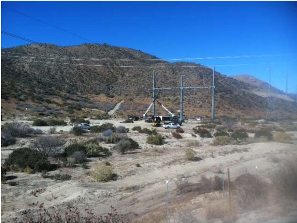
Figure 1: Wire activities at Construct 11, Segment 6.
