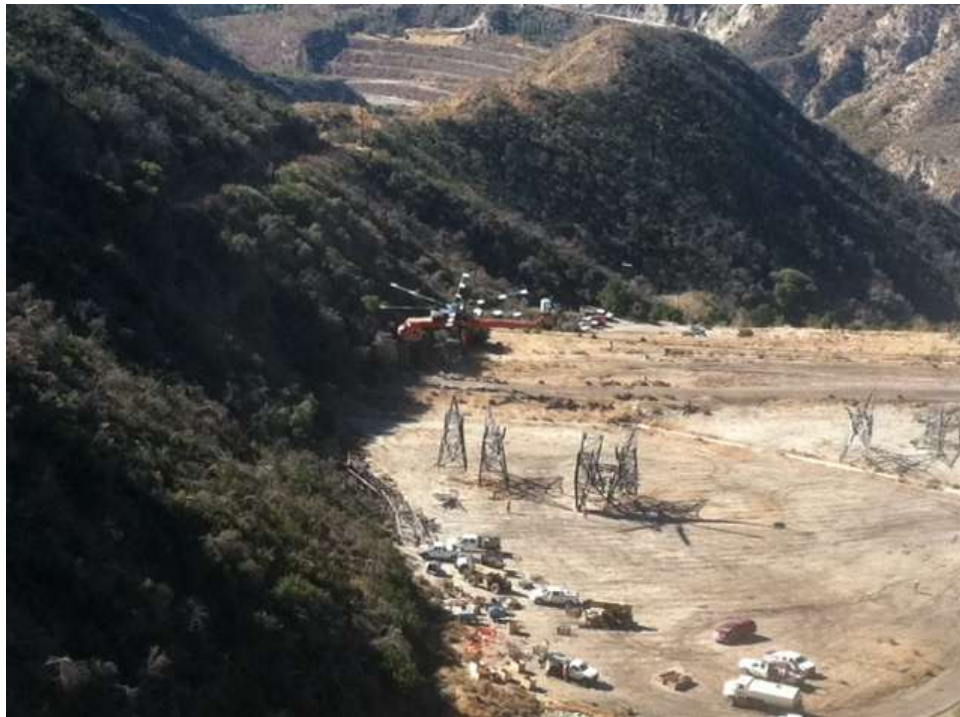
Figure 4: Maple Canyon HAY during tower erection activities, Segment 11C.
