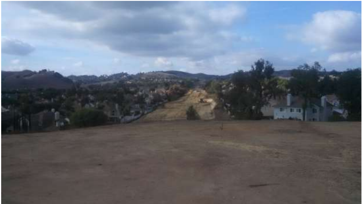
Figure 5: Vegetation has been removed and the right-of-way is being prepared for underground infrastructure installation.
