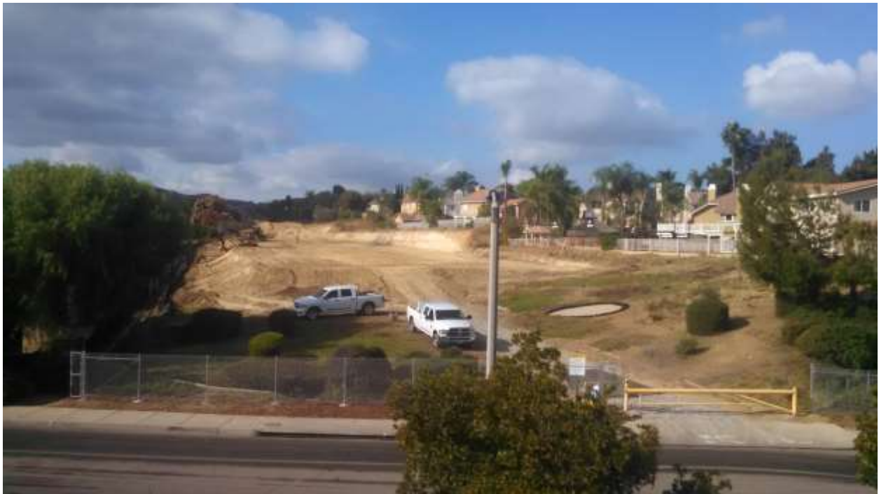
Figure 6: Grading in preparation for vault installation along the Chino Hills right-of-way.
