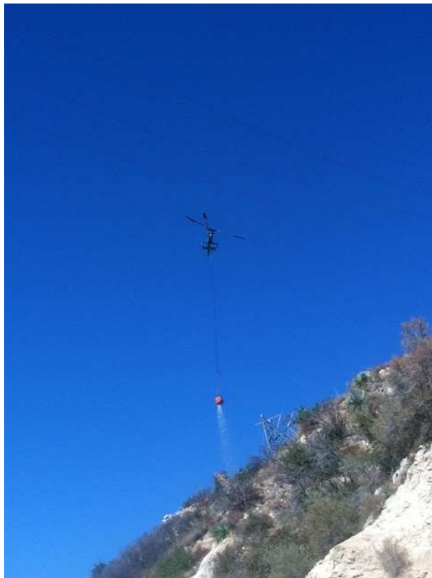
Figure 2: Dust control activity during tower erection at Construct 57, Segment 11C.
