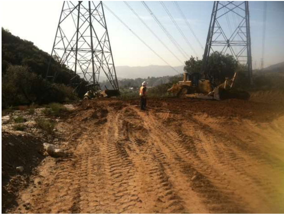
Figure 3: Restoration grading activities at Chaney Trails Wire Setup Site, Segment 11B.
