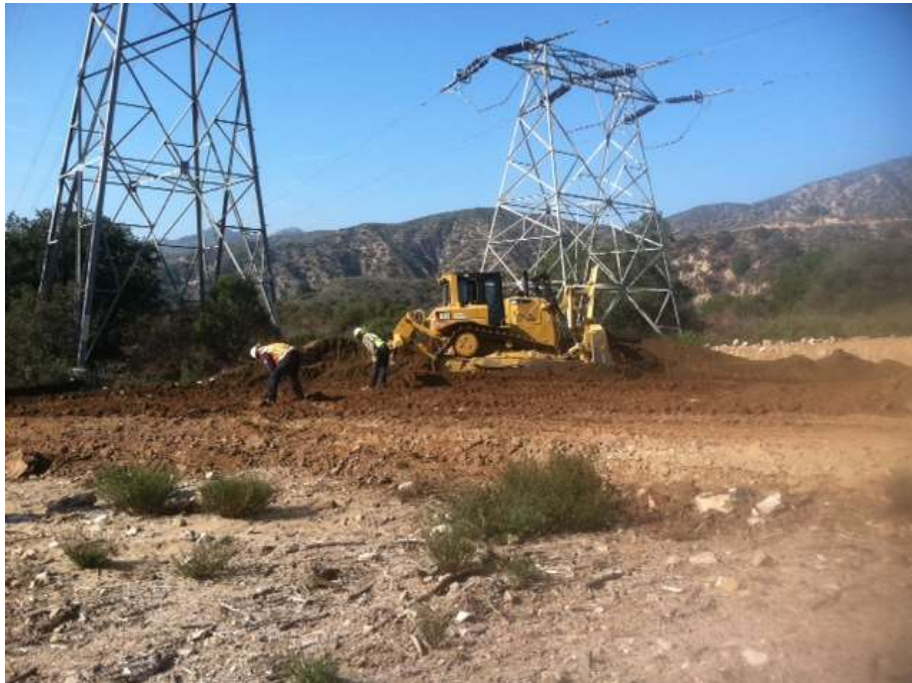
Figure 4: Restoration grading activities at Chaney Trails Wire Setup Site, Segment 11B.
