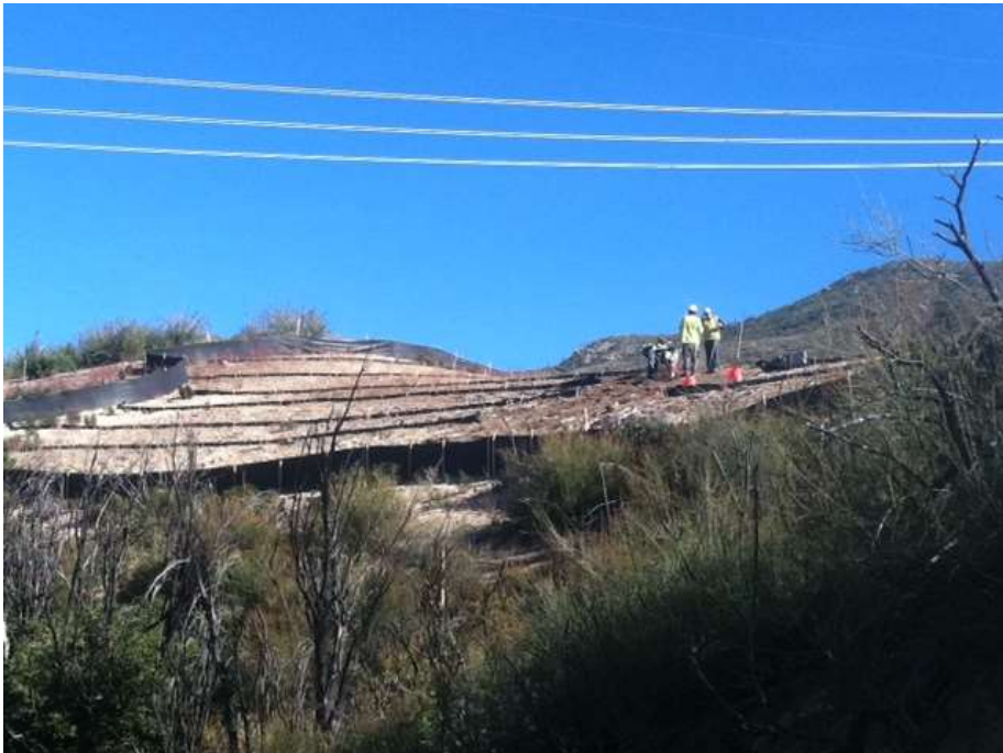
Figure 2: Gully repairs and re-installation of BMPs at Puller/Tensioner Site 62/63, Segment 6B.
