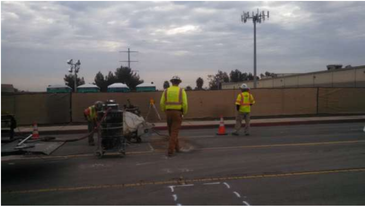
Figure 5: Utility potholing along Pipeline Avenue.
