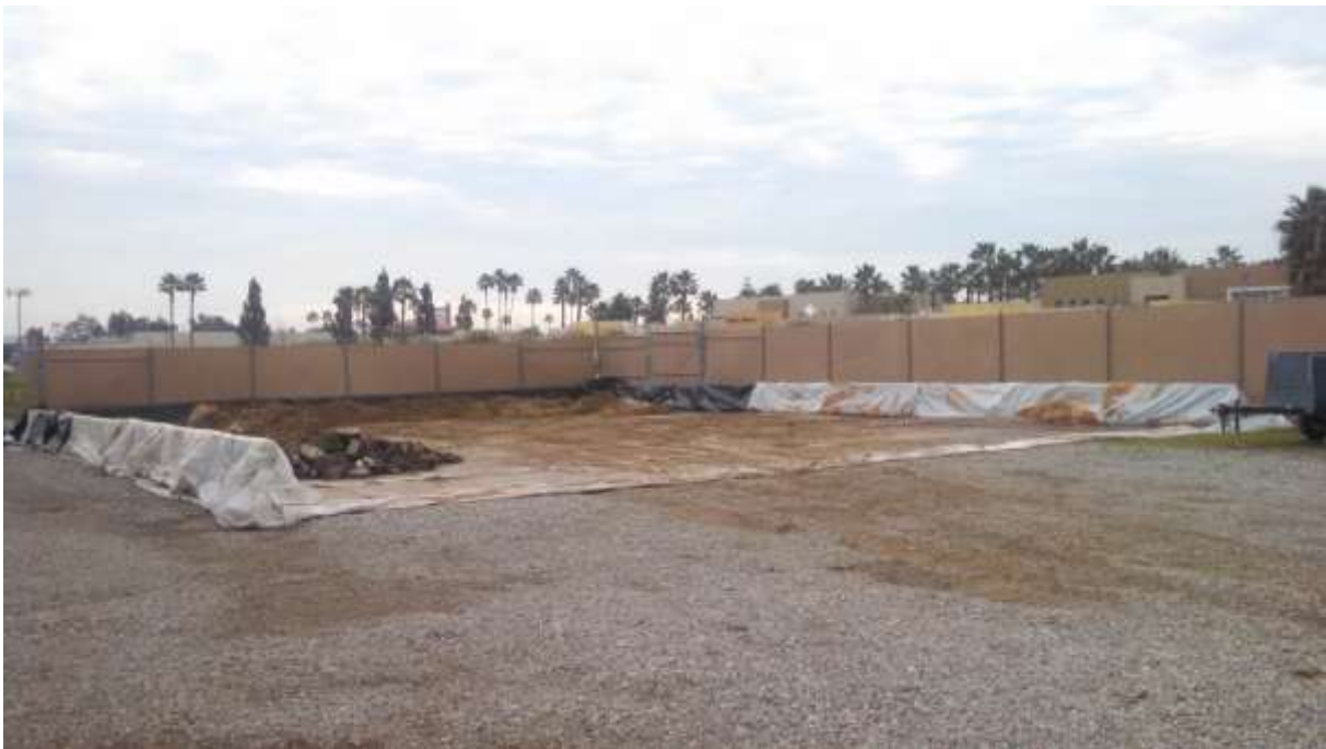
Figure 6: Storage area for cuttings leftover from the directional drilling process.
