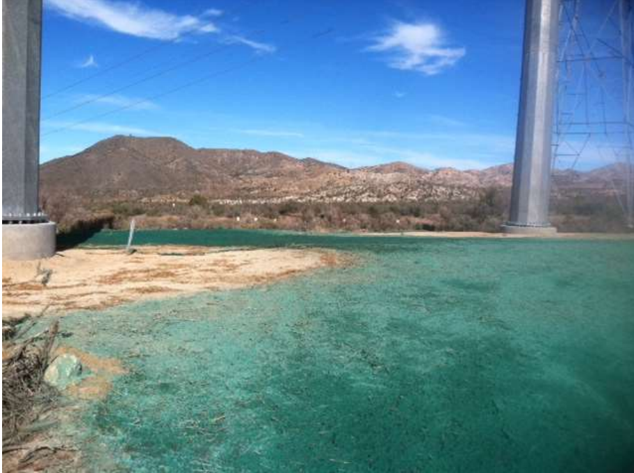
Figure 1: Hydroseeding completed at Construct 15, Segment 6A (USFS).
