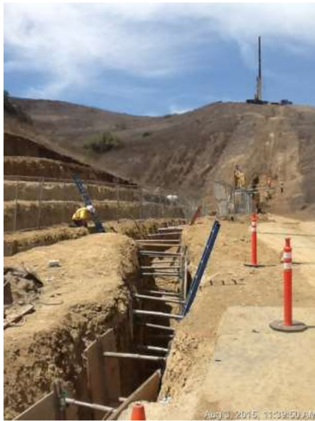
Figure 5: Trenching activities between VC #3 and VC #4, 500 kV Underground.
