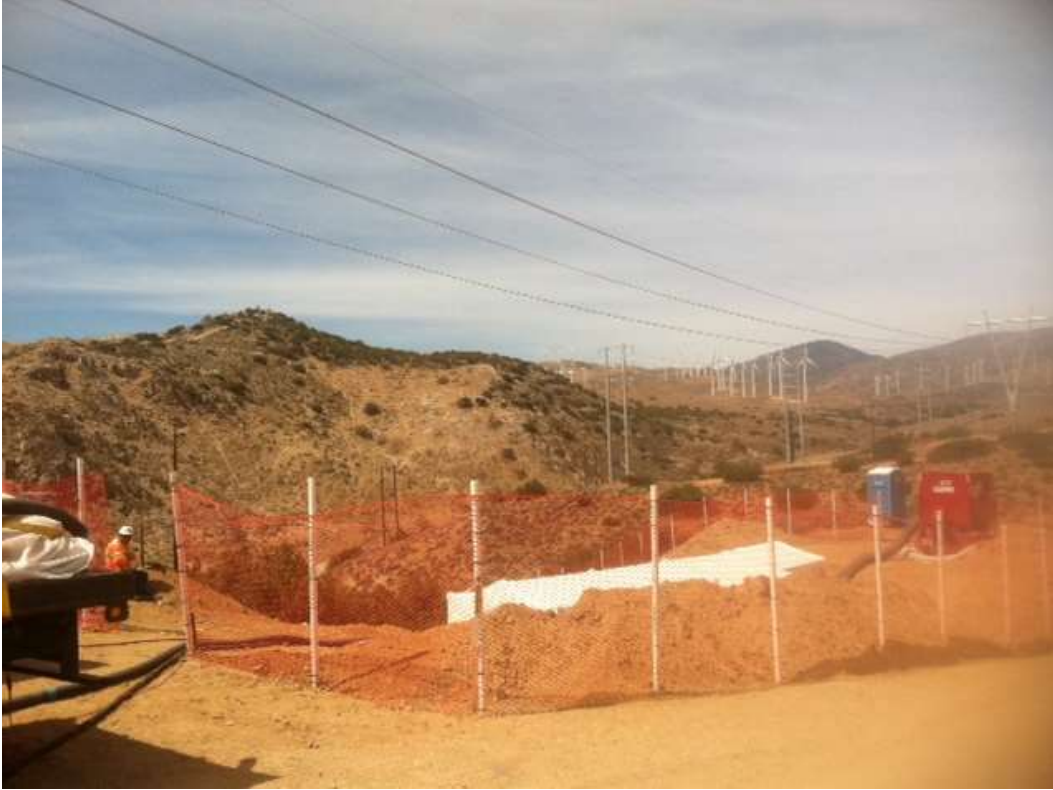
Figure 1: Gas pipeline span burial activities on Segment 3B.
