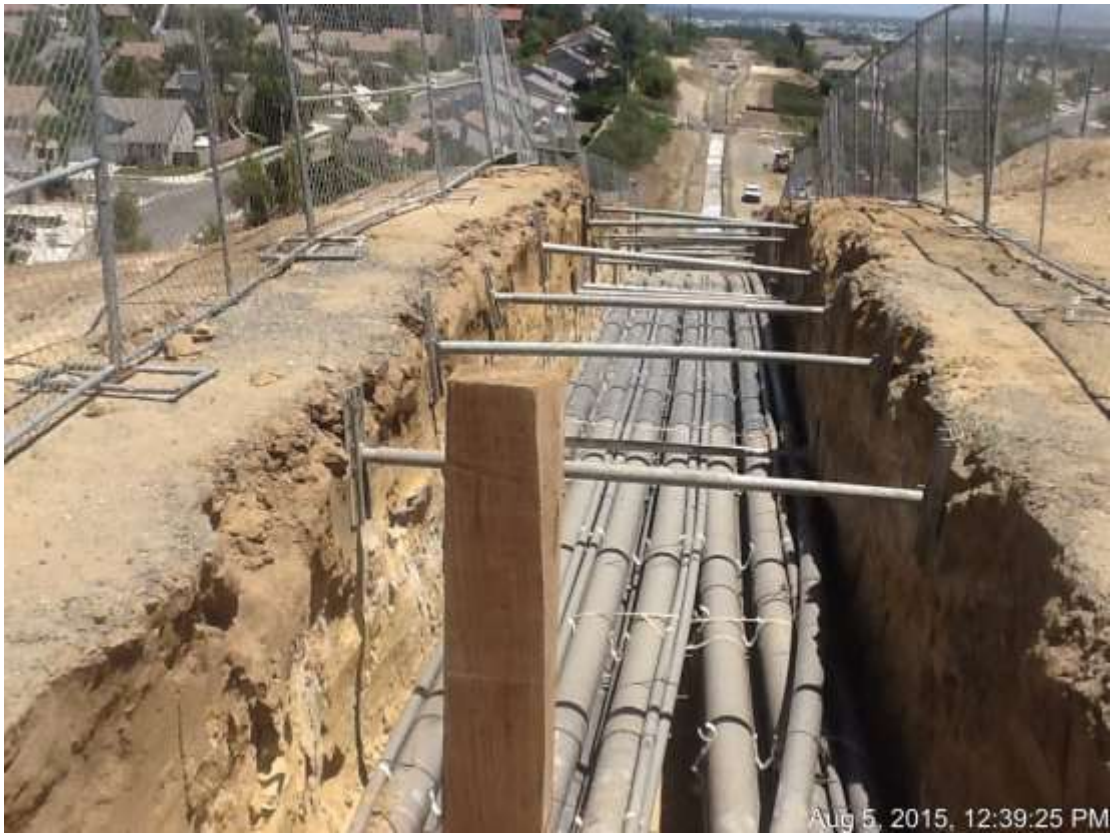
Figure 7: Conduit placement at VC #8, 500 kV Underground.
