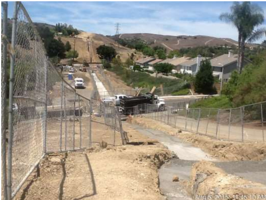
Figure 6: Trenchline at Little Bend up to VC #9, 500 kV Underground.
