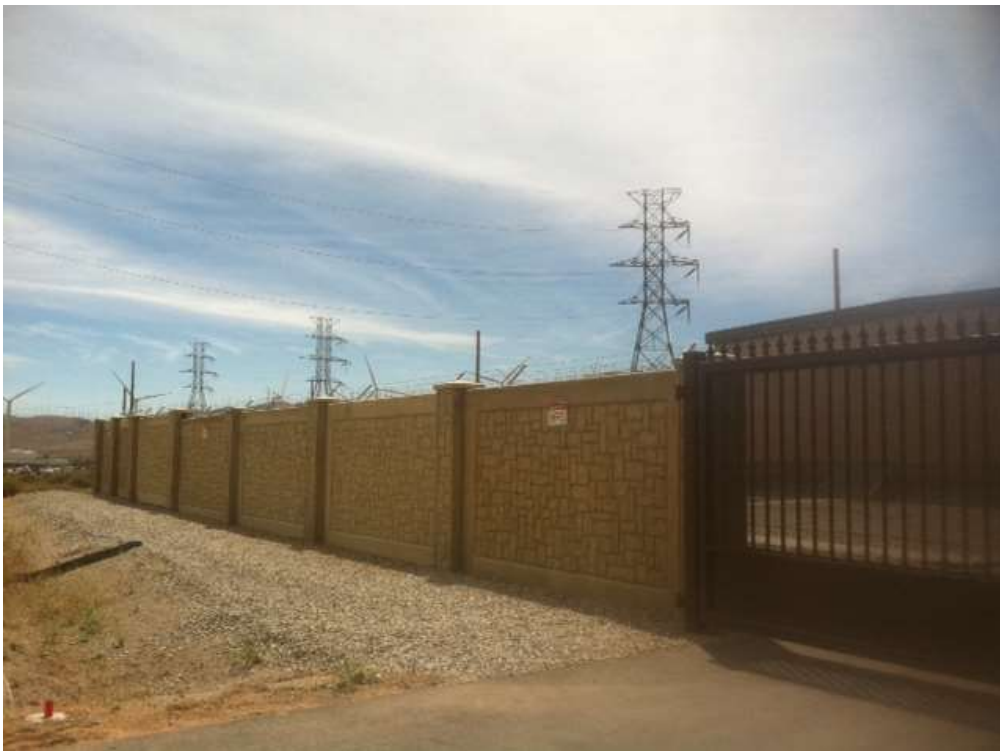
Figure 2: Barbed wire installation along top of wall at Highwind Substation.
