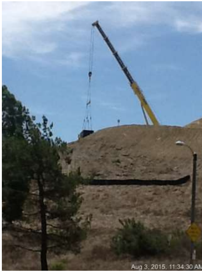
Figure 4: Vault delivery at VC #3 occurred, 500 kV Underground.
