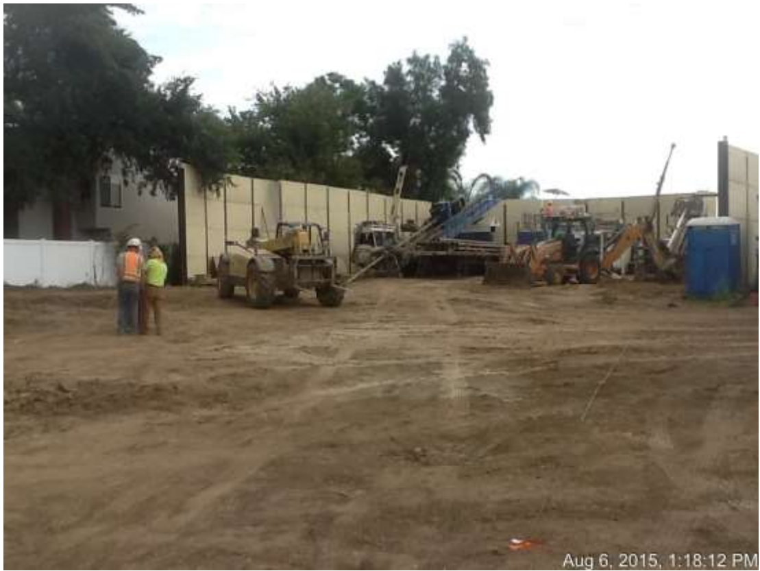
Figure 8: HDD operations at VC #12, 500 kV Underground.
