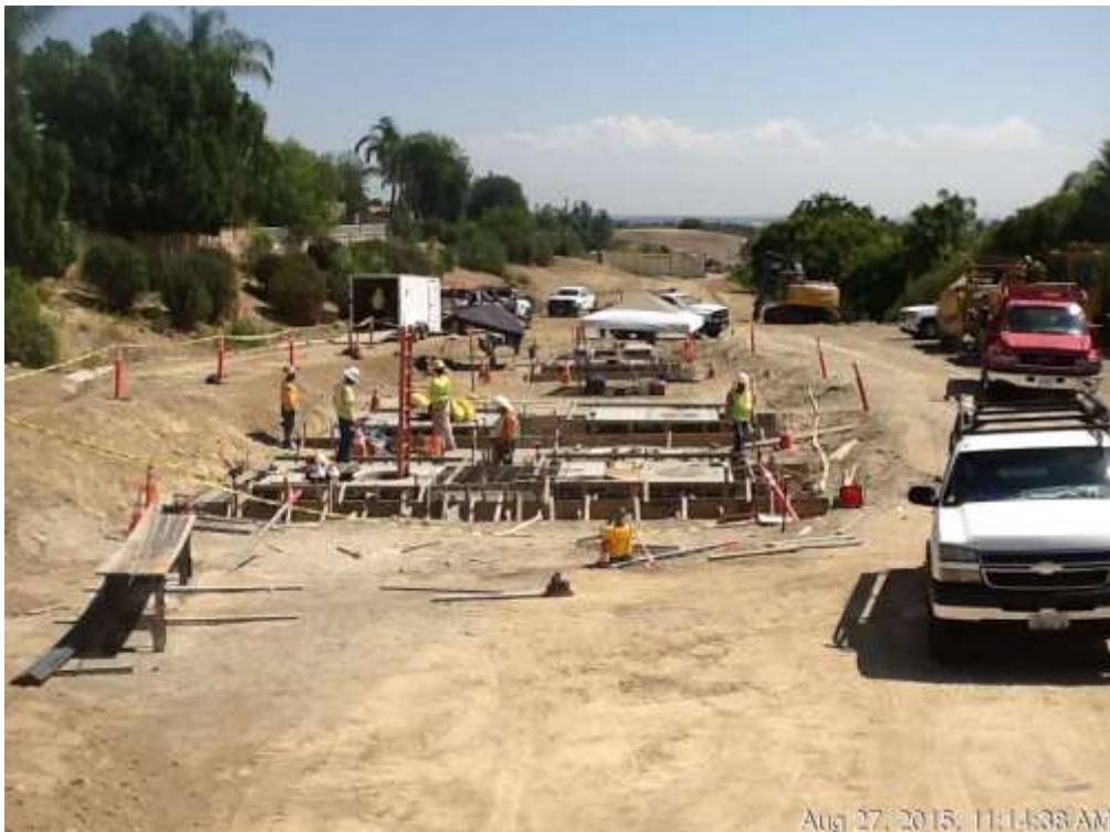
Figure 2: Concrete apron installation at VC #10, 500 kV Underground.
