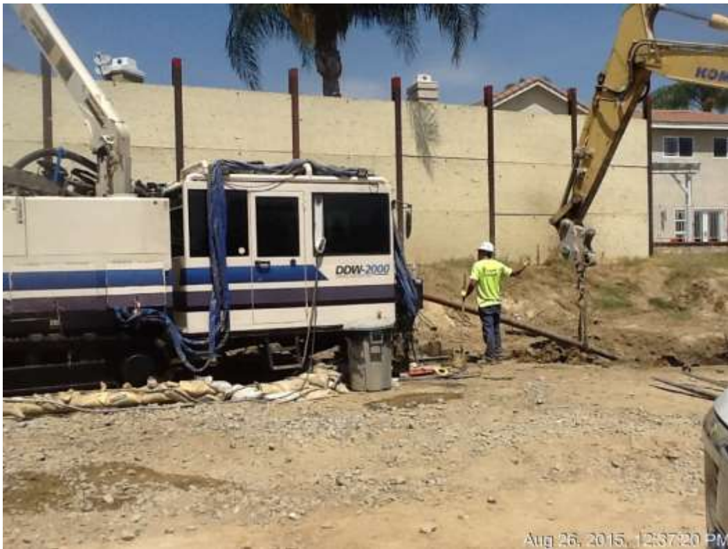
Figure 5: Swabbing activities being completed at VC #11 for conduit installation of HDD C1-S2, 500 kV Underground.
