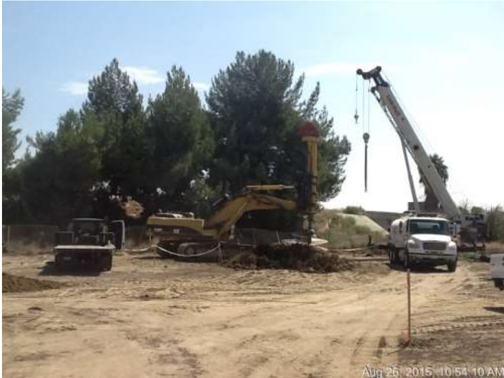
Figure 1: Foundation installation occurring at Transition Tower M64-T1 at the ETS, 500 kV Underground.
