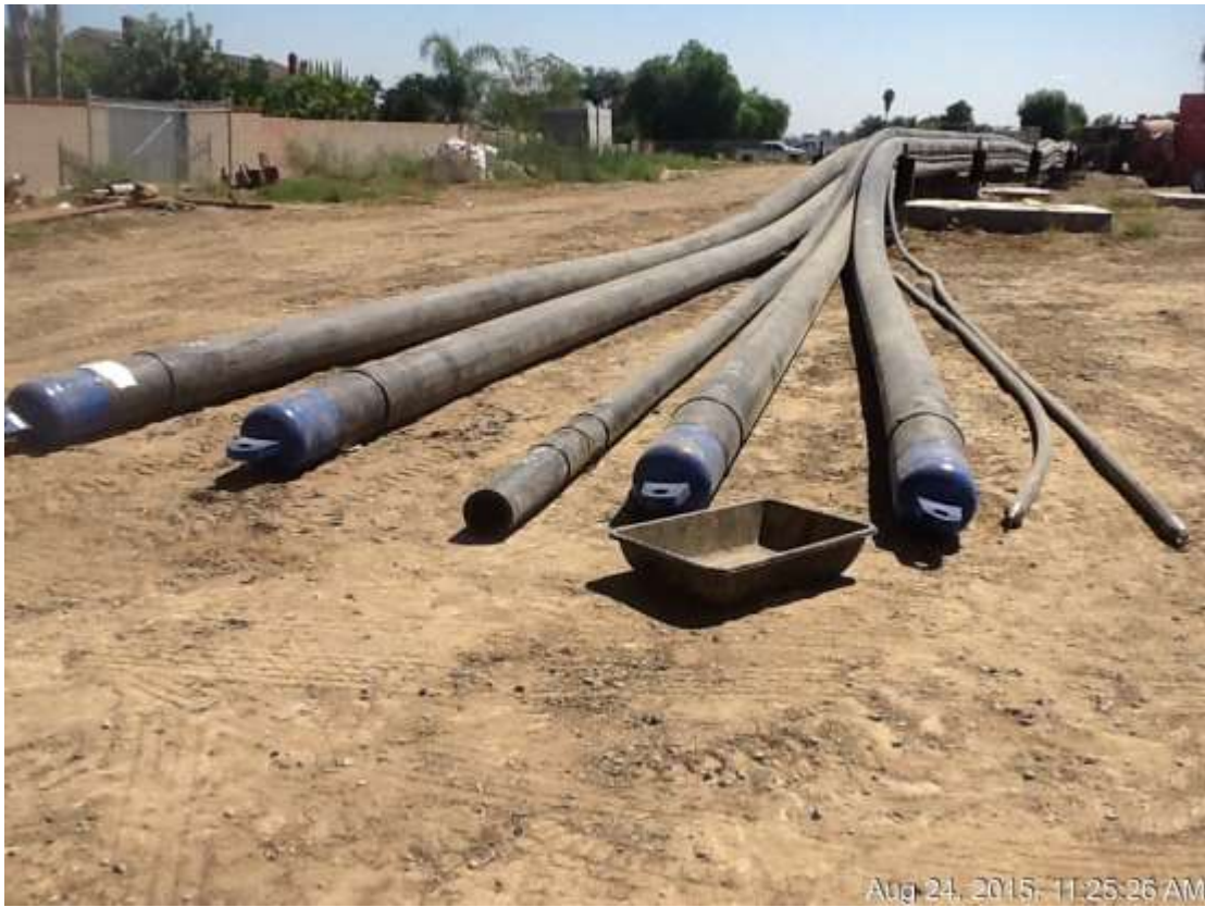
Figure 3: Conduit preparation for pending pulling activities at HDD C1-S2, 500 kV Underground.
