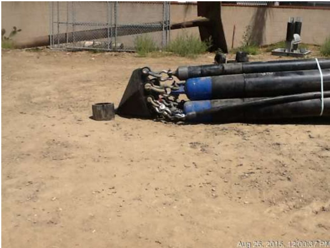
Figure 4: Conduit preparation for pending pulling activities at HDD C1-S2, 500 kV Underground.
