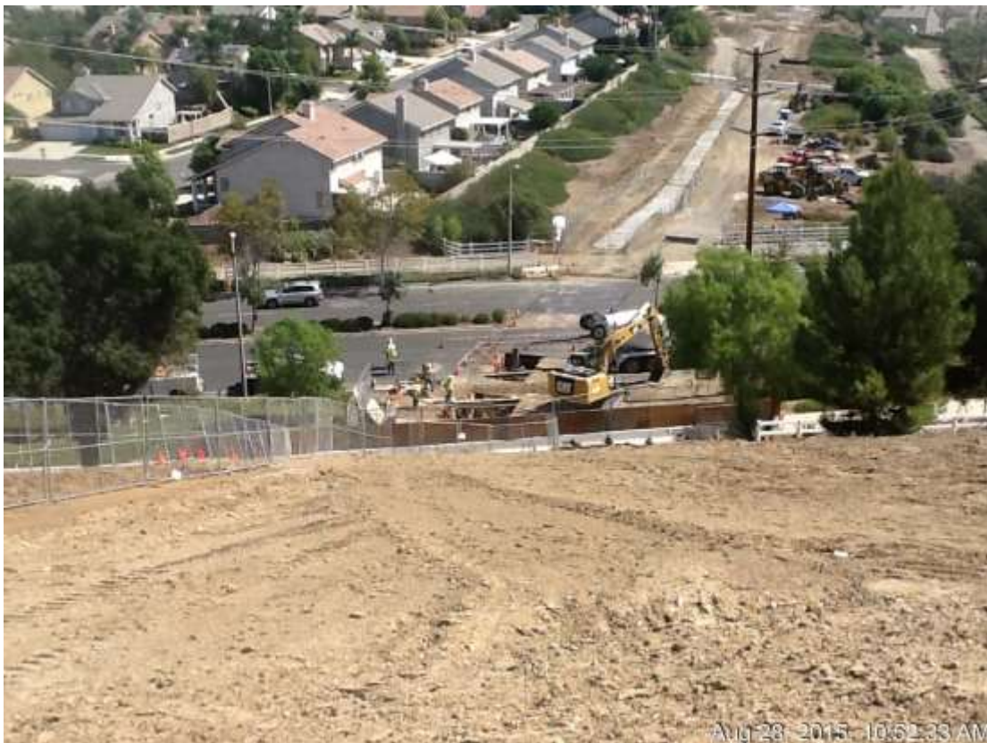
Figure 6: Concrete placement in trenchlines across Chino Hills Parkway, 500 kV Underground.
