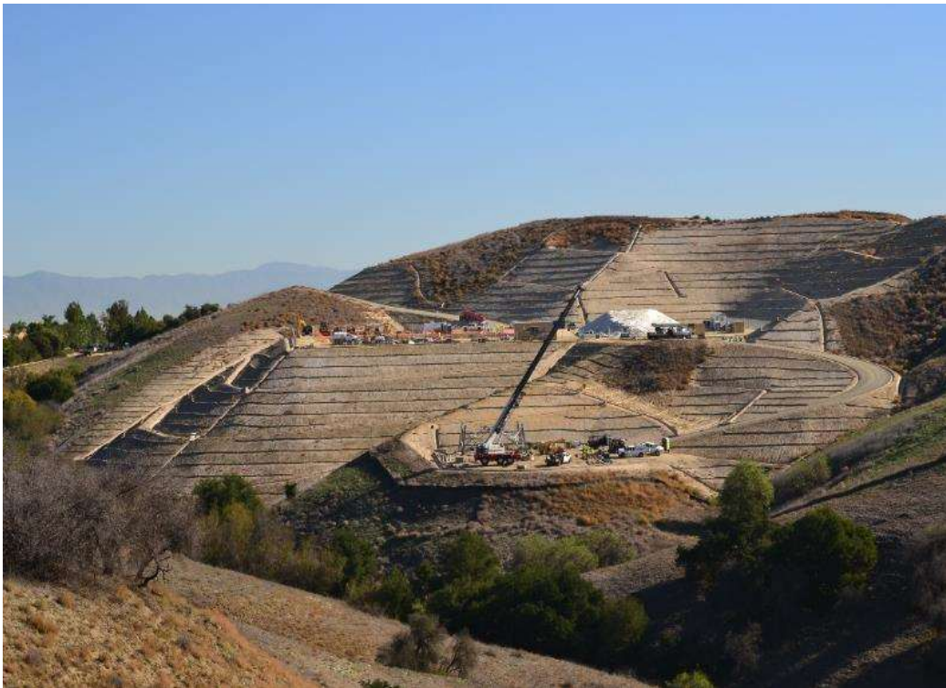
Figure 6: Tower erection at Tower M60-T1X, near the WTS, 500 kV Underground.
