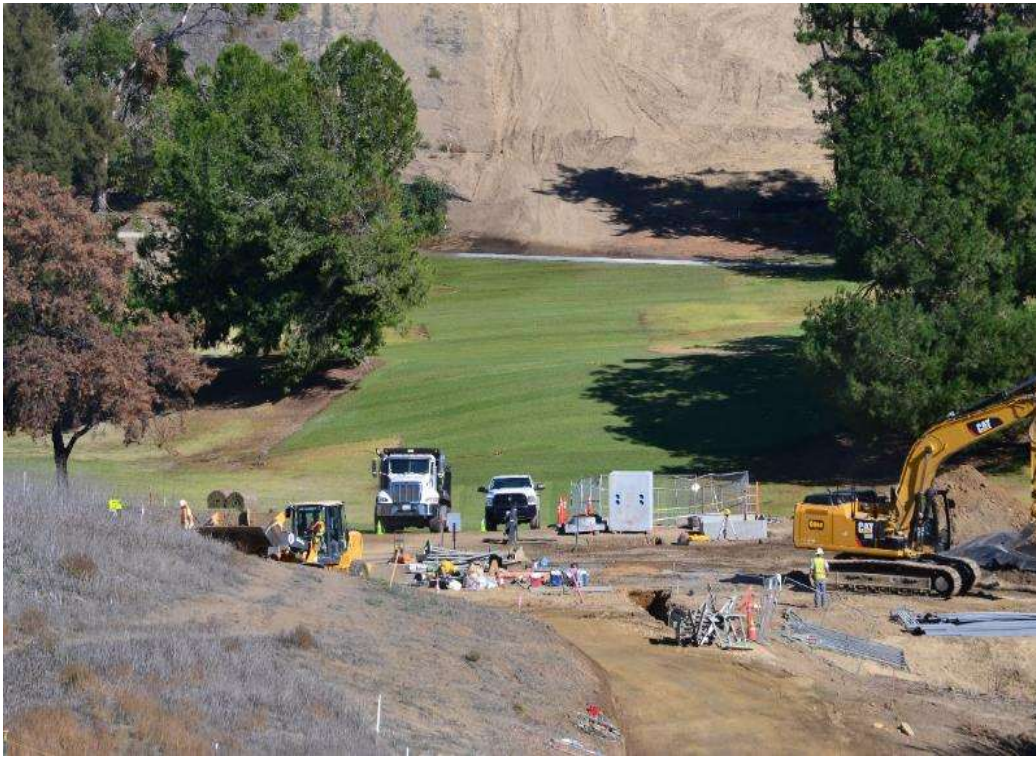
Figure 5: Sod replacement at the golf course, 500 kV Underground.
