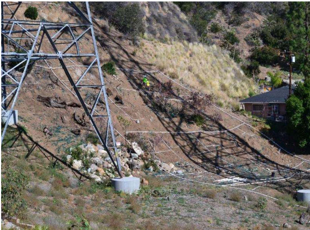
Figure 2: Installation of irrigation system at Tower M27-T4, Segment 7.
