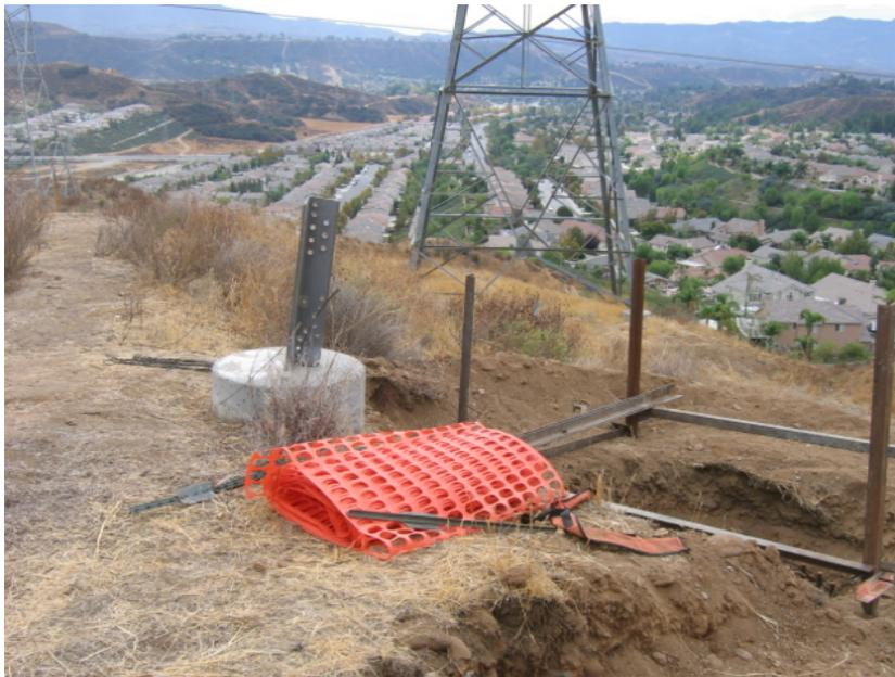
Figure 3: Foundation from the wreck out tower is proposed to be left as is, in stead of being dug down to two feet below grade. SCE was informed to submit a Variance for leaving the two foundations in place.
