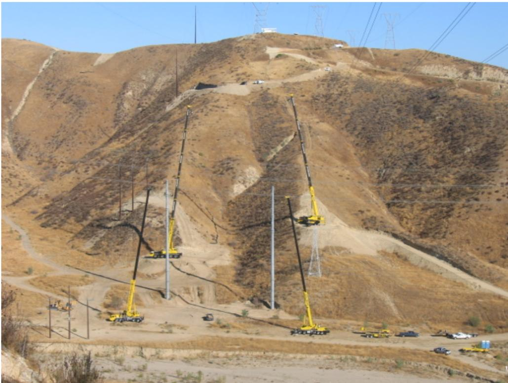
Figure 2: Cranes and steel guard structures were used to protect the LADWP corridor during wire removal over Haskell Canyon.
