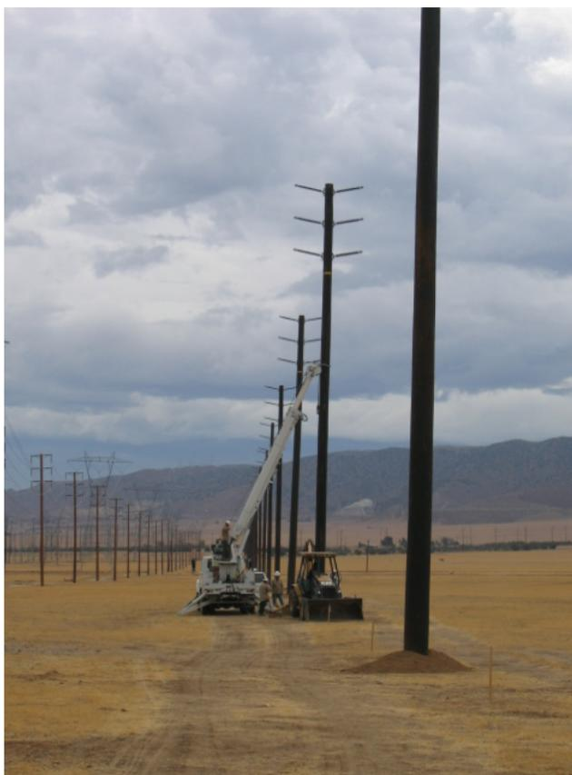
**Figure 5:** On Segment 2, SCE crews began setting wood poles for the relocation of the 66 kV line near the Antelope Substation. The existing 66 kV poles will need to be removed in order to construct the 500 kV structures, later this year.
