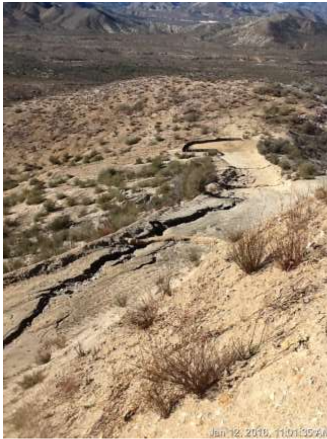
Figure 4: Erosion at Segment 11 Tower 18. This is one of the locations that still needs to be completely recontoured and restored.
