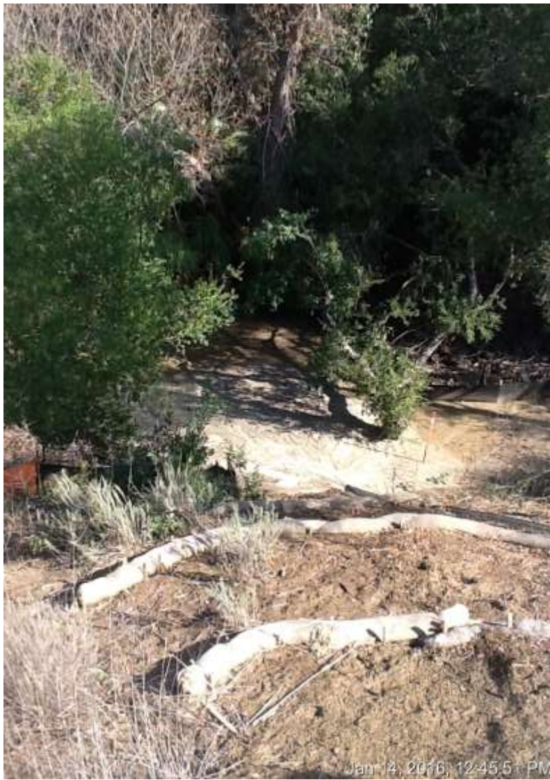
Figure 7: Sediment discharge off the access road at Tower M49-T1. H&M crews have mobilized to the site to begin repair work.
