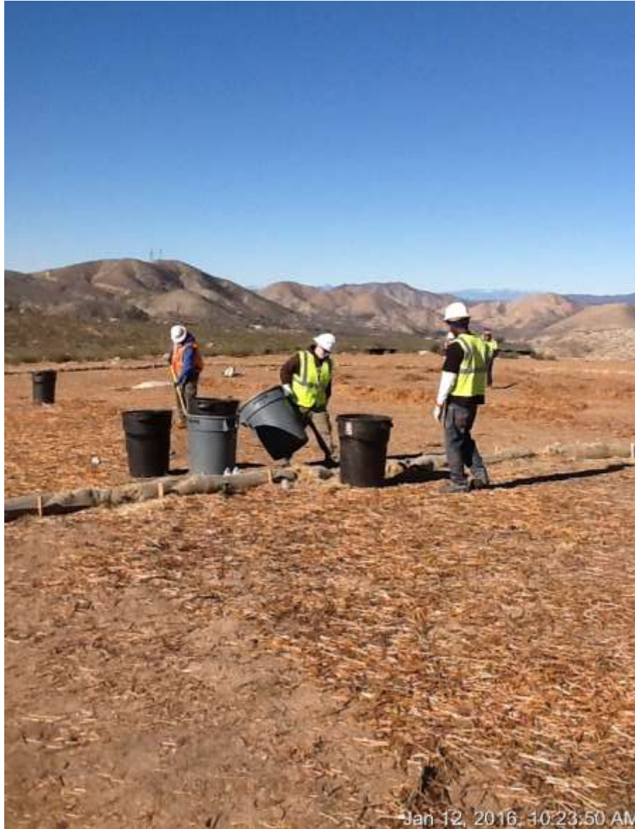
Figure 1: Restoration crews removing wood mulch at Aliso HAY to prepare the site for hydroseeding, Segment 11.
