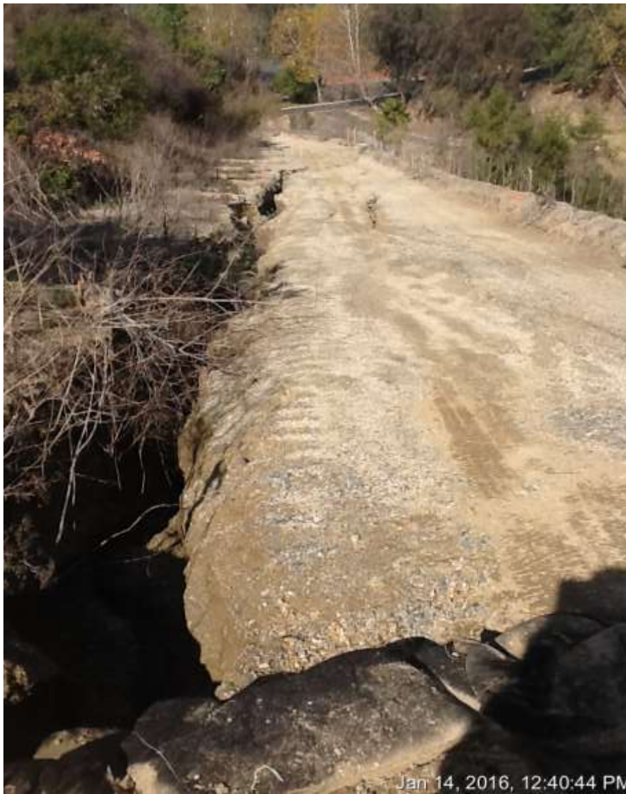
Figure 6: Erosion gully along the access road leading to Tower M49-T1 in Segment 8 Phase 4. H&M crews have mobilized to the site to conduct erosion repairs.
