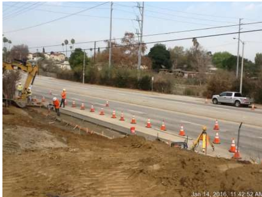
Figure 5: Henkels and McCoy crews constructing an additional driveway entrance at Segment 7 Tower M40-T4.
