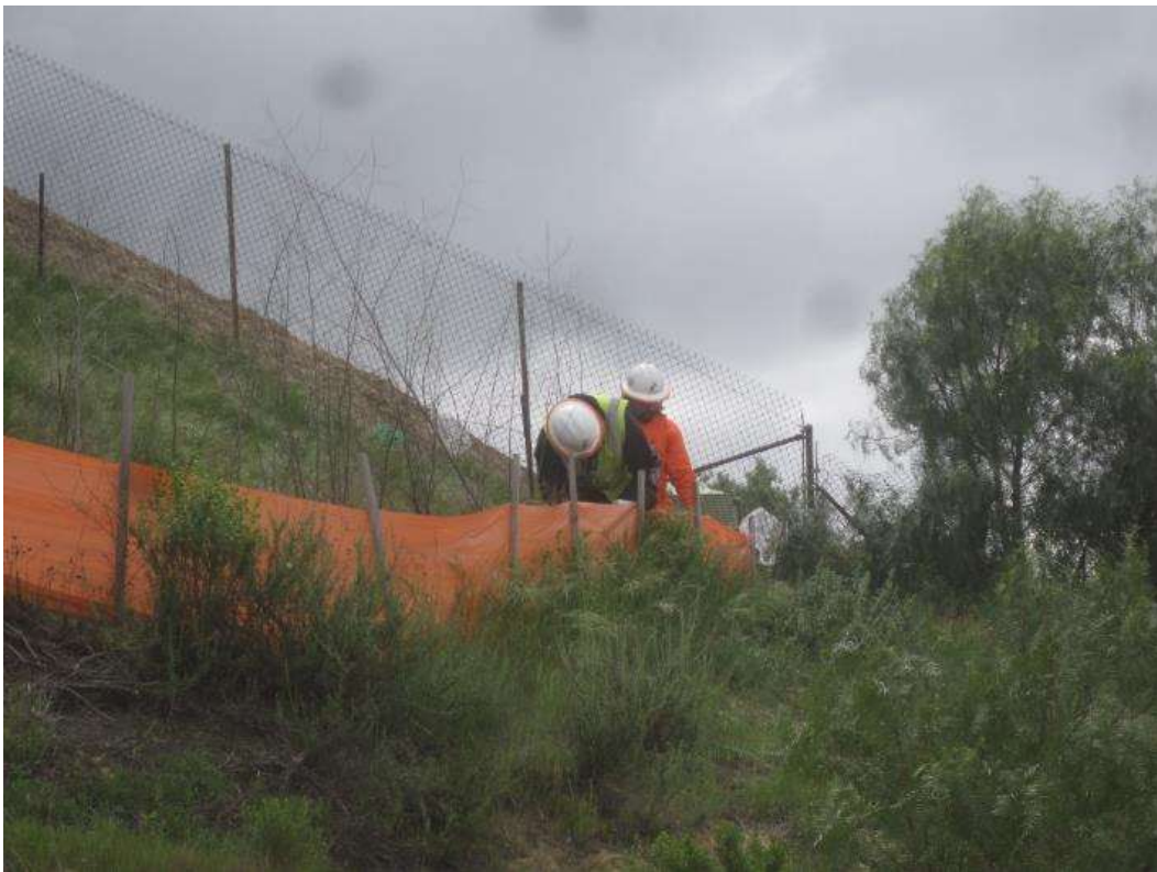
Figure 4: BMP maintenance at Tower M44-T2, Segment 8 Phase 4. Photo courtesy of SCE.
