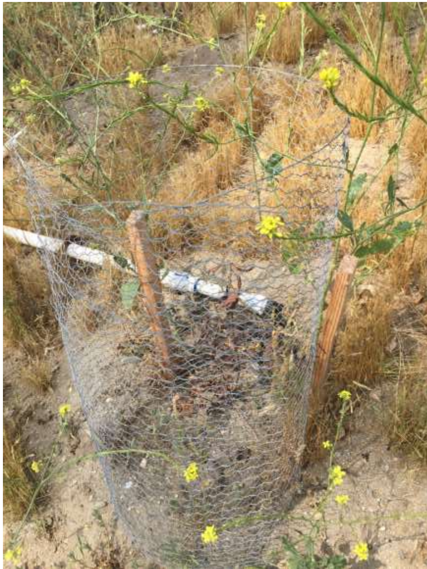
Figure 2: Dead container plant at Tower M38-T5, Segment 7 Whitter Narrows restoration site.
