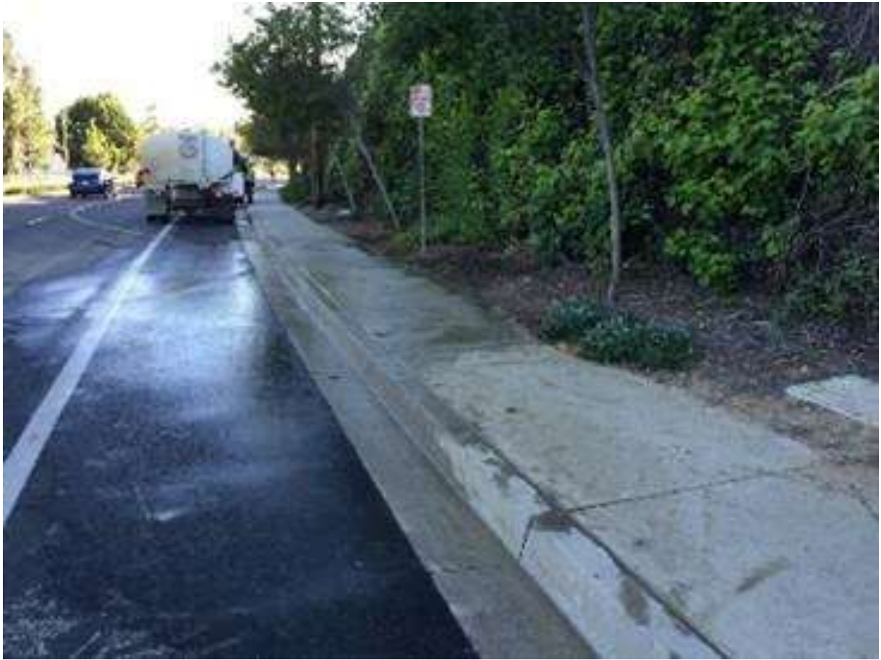
Figure 5: After clean-up photo of frac-out location along Peyton Avenue, 500 kV Underground.
