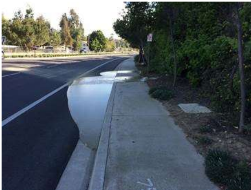
Figure 4: Frac-out along Peyton Avenue in Chino Hills, 500 kV Underground. The spill was contained and did not enter any storm drains or jurisdictional drainages.
