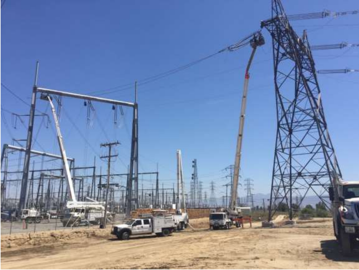
Figure 1: SCE crews completed conductor OPGW and static wire connections from Segment 8 into the Mira Loma Substation.
