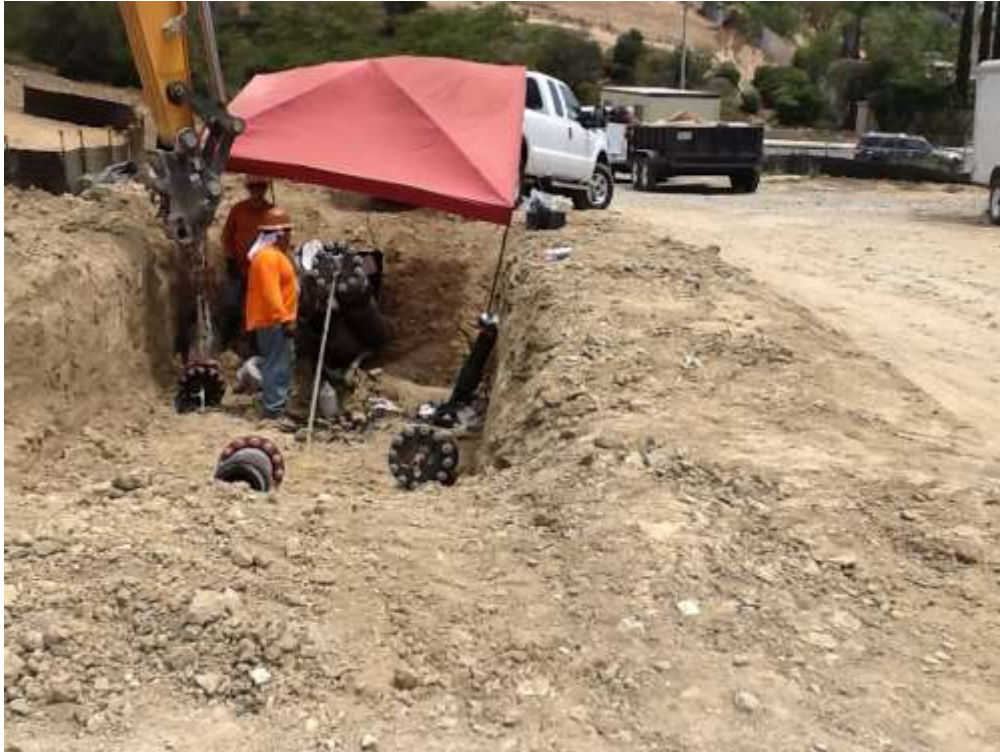
Figure 1: Pressure testing of the HDD casings near VC #11, 500 kV Underground.
