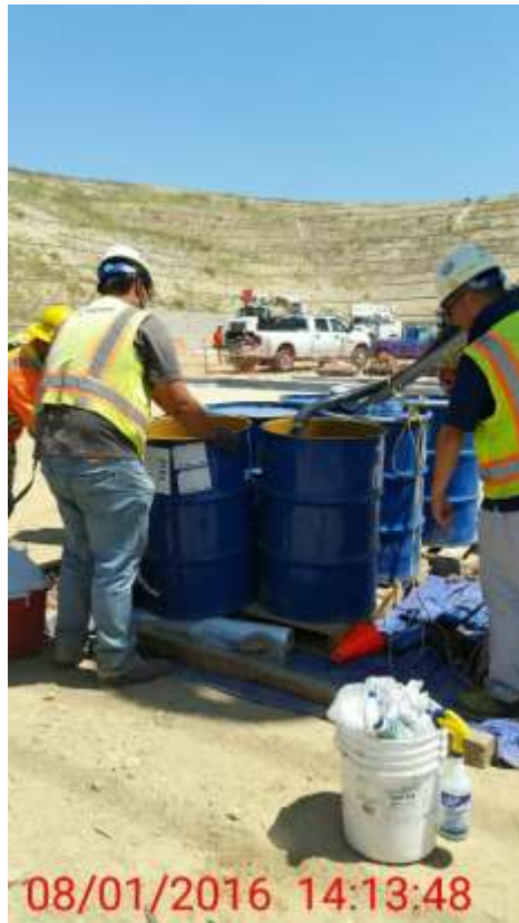
Figure 4: Crews contained and removed contaminated materials from a silicon spill at the WTS during cable removal operations, 500 kV Underground. Photo courtesy of SCE.
