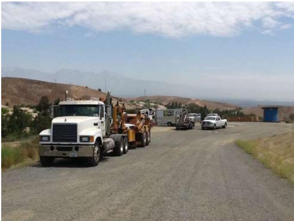
Figure 2: Cable replacement operations at VC #1 to remove one damaged cable from the WTS, 500 kV Underground.
