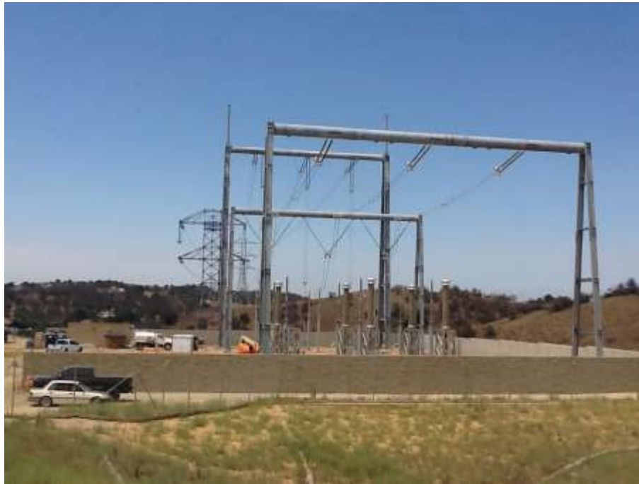
Figure 3: SCE crews completed conductor OPGW and static wire connections from Segment 8 into the WTS, 500 kV Underground.
