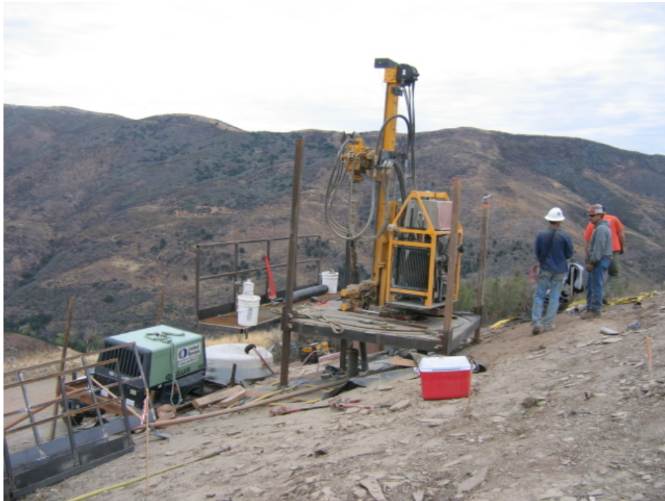
Figure 5: Micropile verification testing took place at the Tower 56 location.
