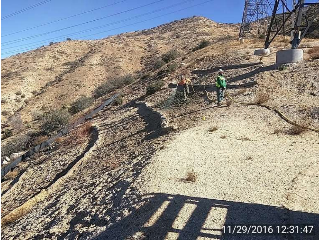
Figure 1: Hydroseeding at Tower 12X, Segment 11. (Photo courtesy of SCE.)
