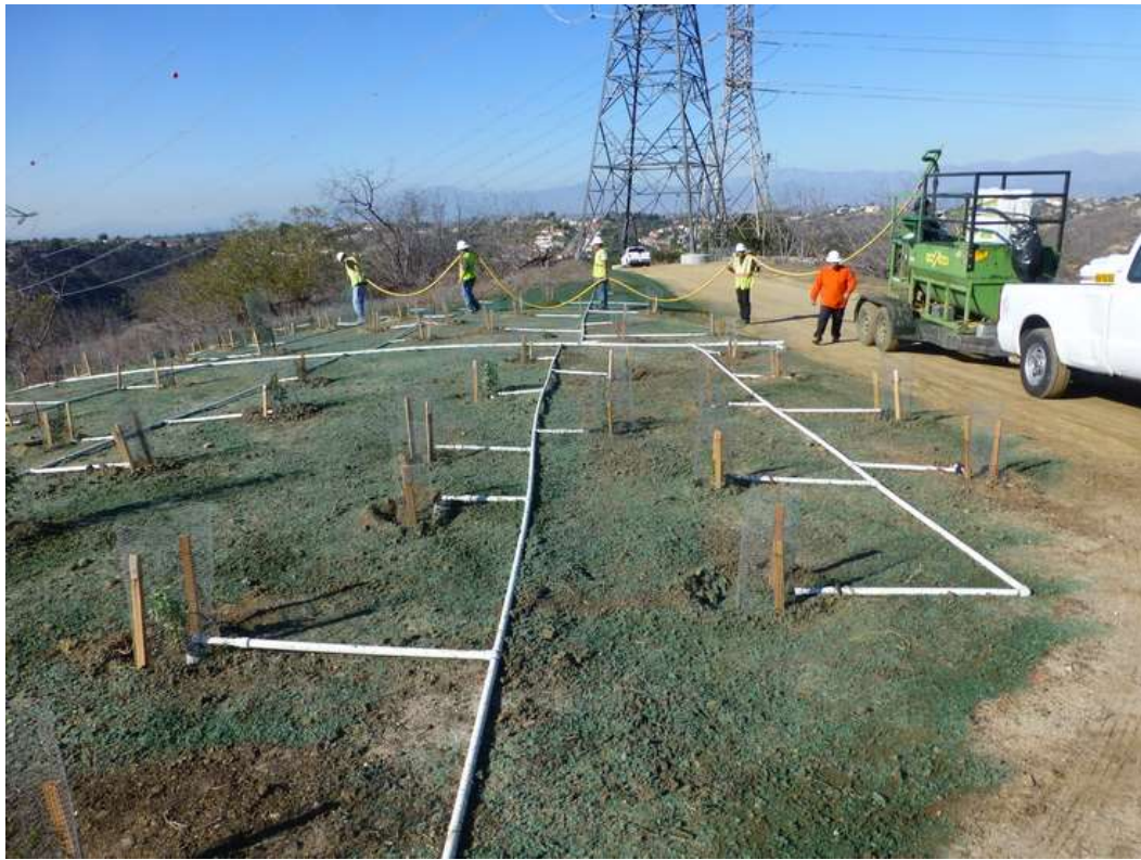
Figure 2: Weed abatement activities at Tower 57-2, Segment 8. (Photo courtesy of SCE.)
