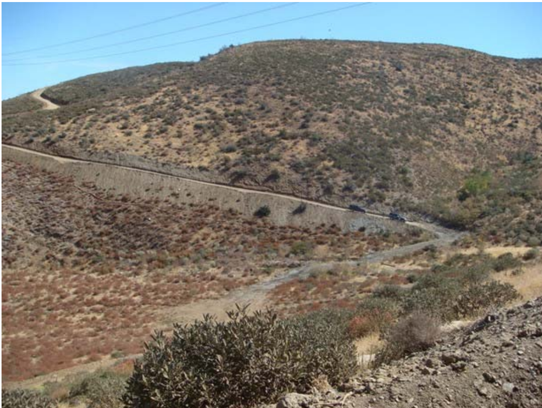
Figure 2: Temporary drainage crossing measures removed near Tower 46, Segment 2.
