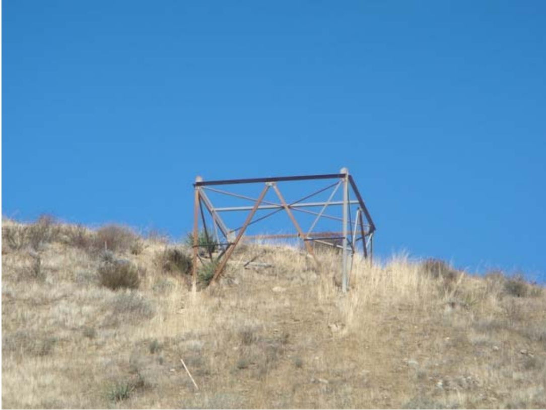
Figure 1: 66 kV Tower base left in Section 1.
