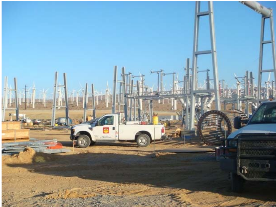
Figure 4: PAR crews conducting foundation drilling within Windhub Substation for the temporary bypass.
