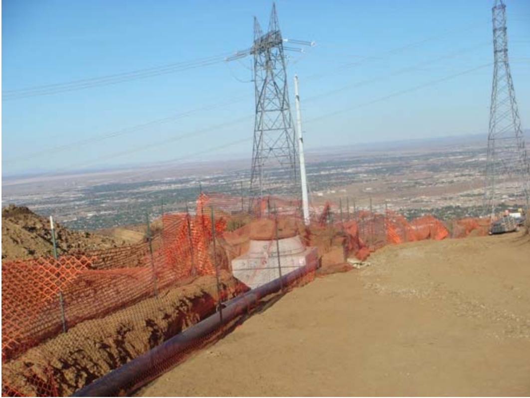
Figure 3: Trenching for fiber optic installations between towers in the hijacks, Segment 2.
