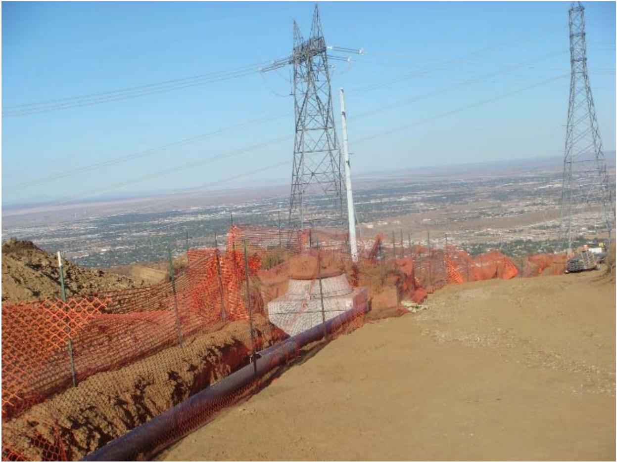
**Figure 3:** Fiber optic trenching at Tower 22, Segment 2.
