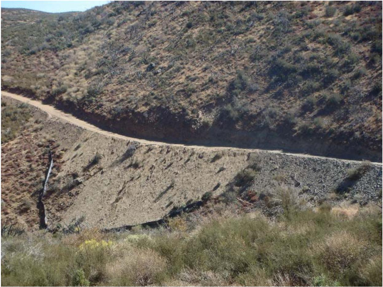
**Figure 2:** Side cast material along access road near Tower 48, Segment 2.
