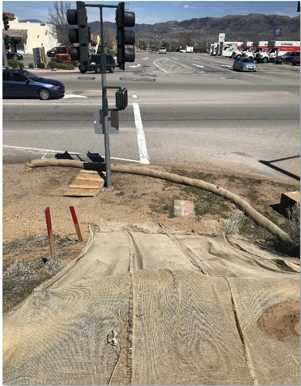
Figure 20. Areas disturbed during trenching activities were stabilized with erosion control blankets and later sprayed with hydroseed
