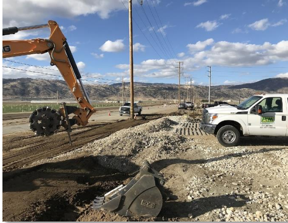
Figure 2. Construction of the stabilized construction entrance to the Banducci Substation built consistent with SWPPP requirements
