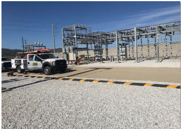
Figure 6. Base rock and rock driveway completed inside of the Banducci Substation (Photo courtesy of SCE)
