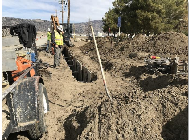
Figure 12. Crews installing conduit for the underground distribution line along Pelliser Road
