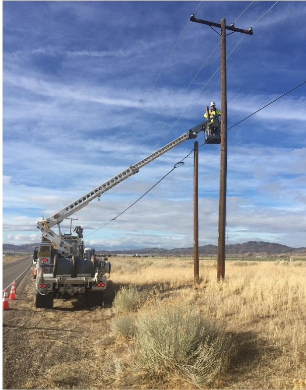
Figure 16. Henkels and McCoy telecom crews installing cable on existing wood poles along Highline Road near Tehachapi
