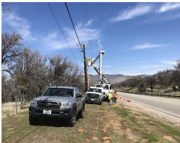
Figure 18. Distribution pole replacement along Highway 202 in Tehachapi
