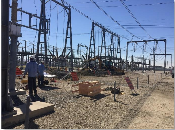
Figure 5. Bus structures and circuit breakers were installed at the Banducci Substation
