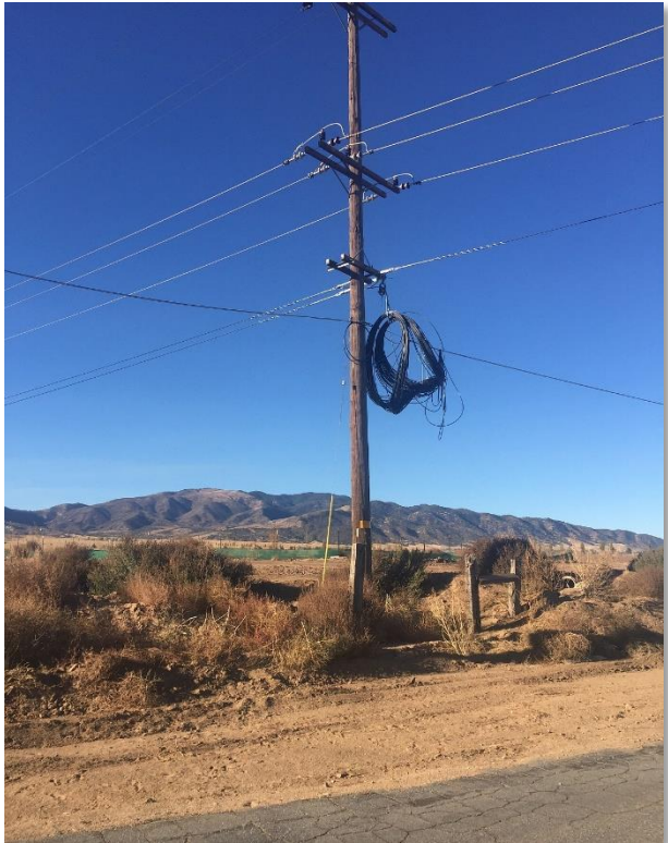
Figure 17. Telecom cable installed onto existing pole with excess cable ready for the Highway 58 Freeway crossing
