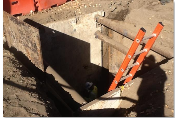
Figure 15. Bore pit for conduit installation under a culvert near Highline Road
