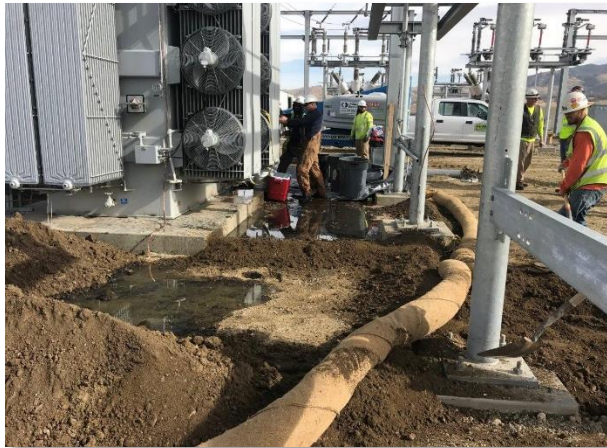
Figure 9. Spill and containment of the mineral oil spill from the damaged transformer
