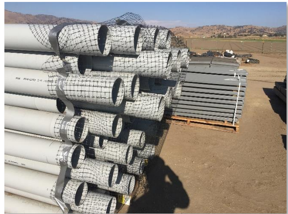
Figure 11. Open pipes were covered consistent with Mitigation Measure requirement to minimize wildlife entrapment
