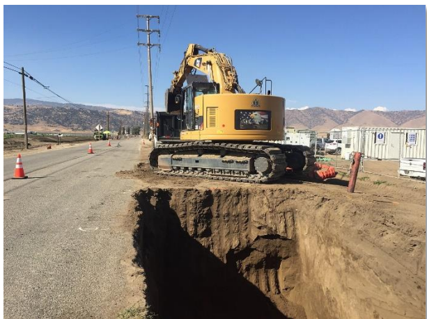
Figure 14. Traffic control was in place during vault excavation for the underground distribution work along Pelliser Road
