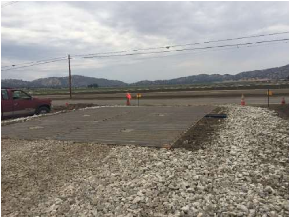
Figure 5 – Stabilized construction entrance was constructed at the substation site.
