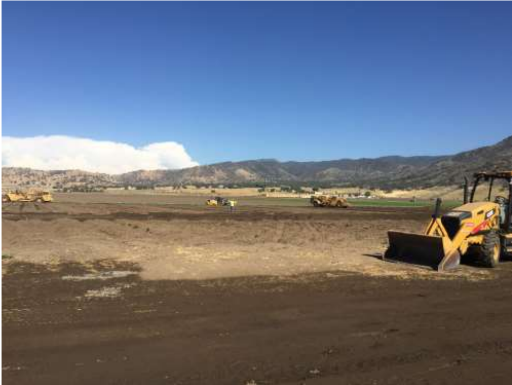
Figure 1 – Construction crews began grading activities at the Banducci Substation, July 26, 2017.
